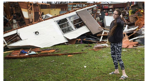
Homes destroyed by Hurricane Michael in Panama City, FL. Image source: P. 158
