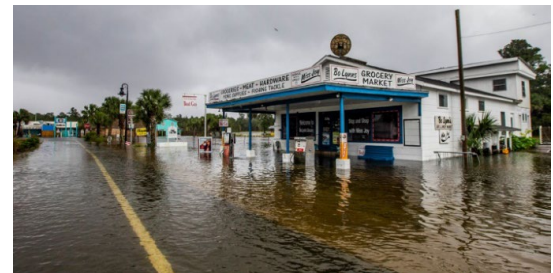
Flooding and destruction in St. Marks, Florida. Image source: AP. 159
