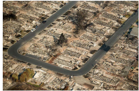
A burned out and collapsed neighborhood in Napa, CA after the Nuns fire. Source: Peter DaSilva/Special to the Chronicle 190
