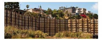
Temporary sound walls, like the ones at PDR, are commonly used in the natural gas industry to effectively block noise from propagating into the surrounding environment.
