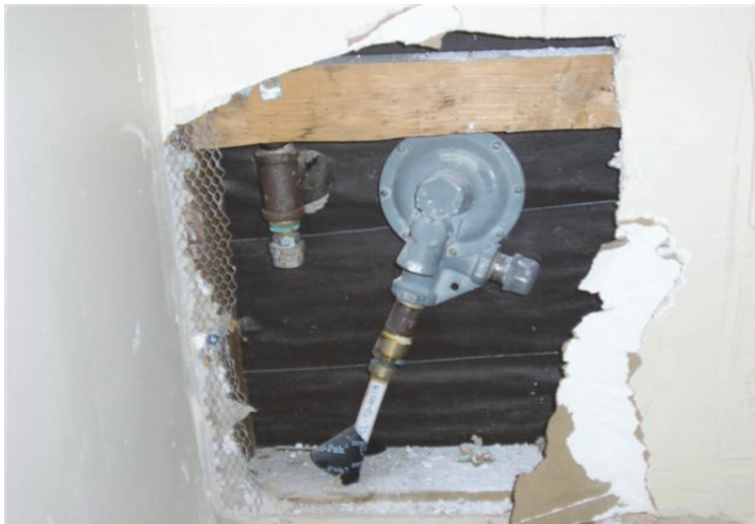
Someone tapped into SoCalGas' district pressure service and ran gas into the wall of the closet. A regulator was installed inside the wall and the wall was closed, leaving the regulator with nowhere to vent.
