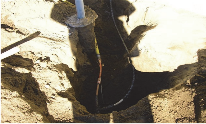
Someone tapped into SoCalGas' district pressure service and ran gas into the wall of the closet. A regulator was installed inside the wall and the wall was closed, leaving the regulator with nowhere to vent.
