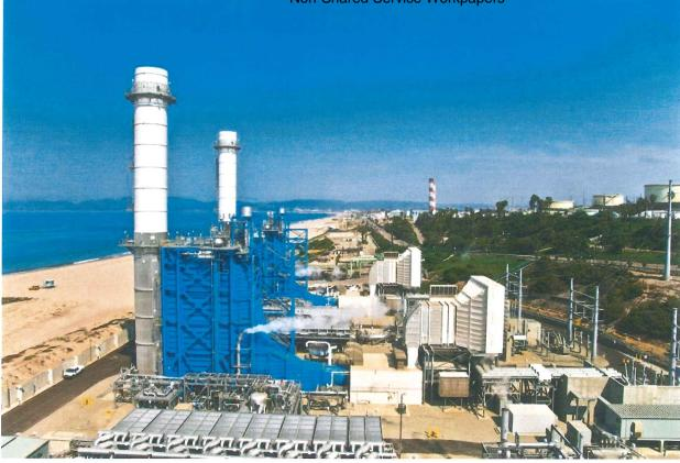
California's El Segundo Energy Center is the second power plant in the United States to be outfitted with technology that allows it to ramp up or down quickly with natural gas to accommodate a shifting supply of renewable energy.
