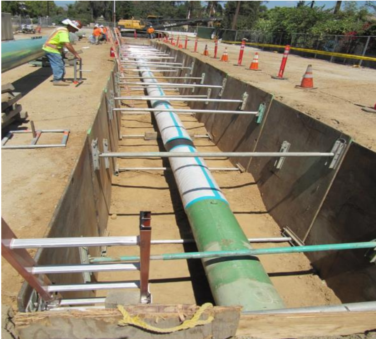
Figure 13: Exposed pipe on Section 5 with protective wrap in preparation for removal and asbestos abatement
