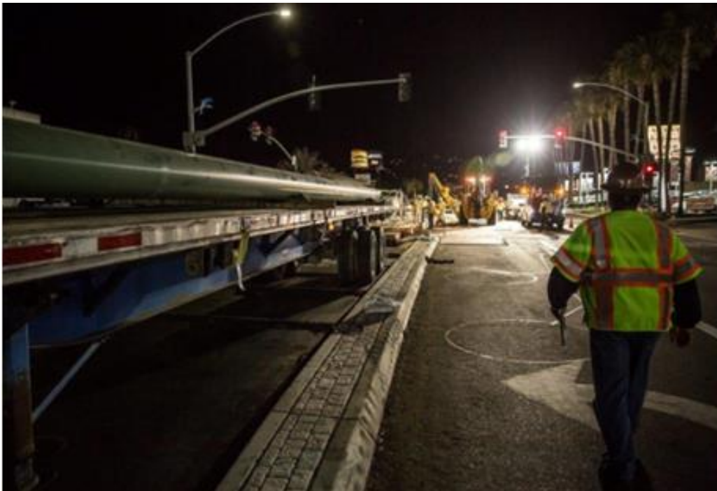
Figure 4: Night Work Construction Site
