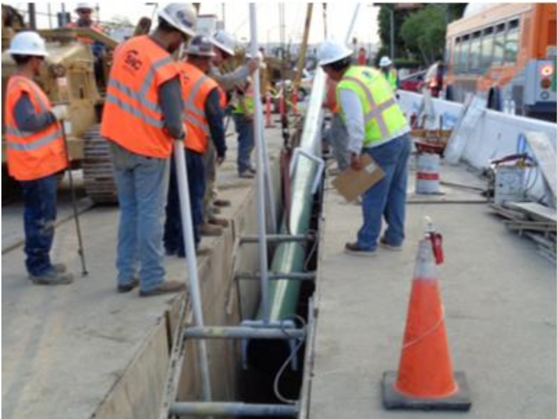
Figure2: Lowering Pipe in Congested City Area
