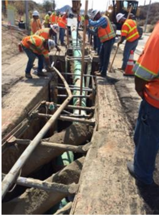
Figure 3: Installing Pipe in Trench with Existing Substructures
