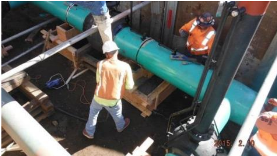
Figure 8: L-1005 Site 2 – Installation of New Valve and Supports
