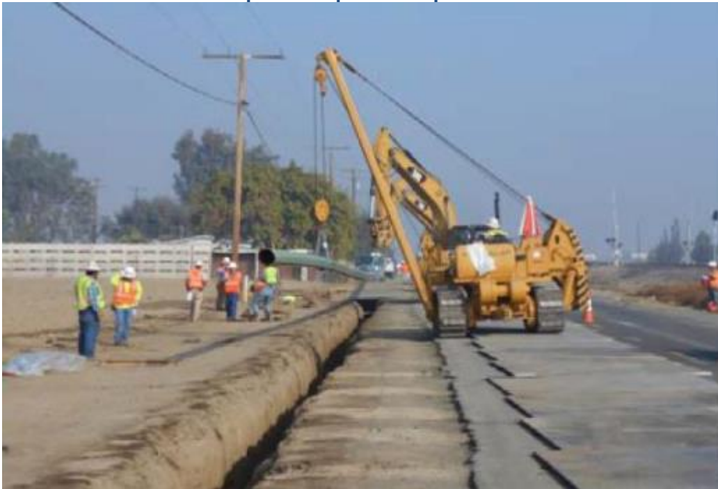
Figure 3: Placing Pipe in Trench with Side Boom Equipment along S I Street and plates to protect asphalt
