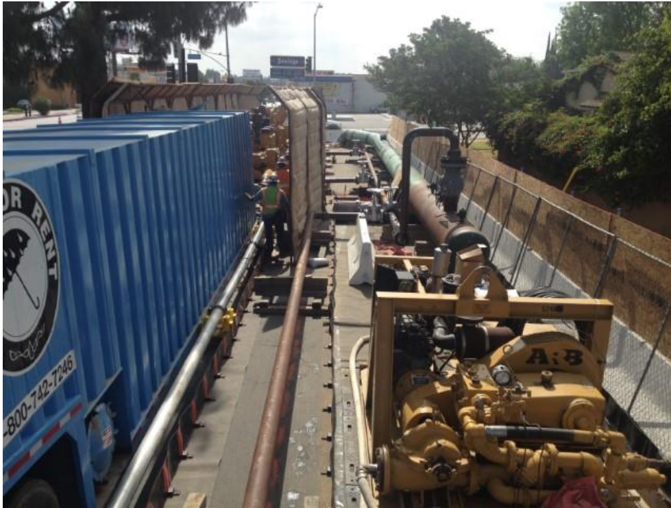
Figure 7: L-407 North Section work area showing Baker Tanks with sound proofing
