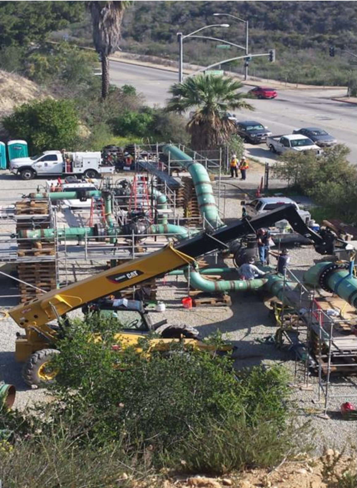
Figure 10: Above-Ground Pre-Fabrication of Valve Assembly
