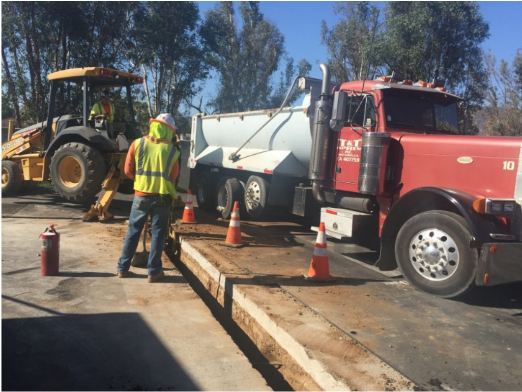
Fig. 3: Digging and hauling equipment used during trenching
