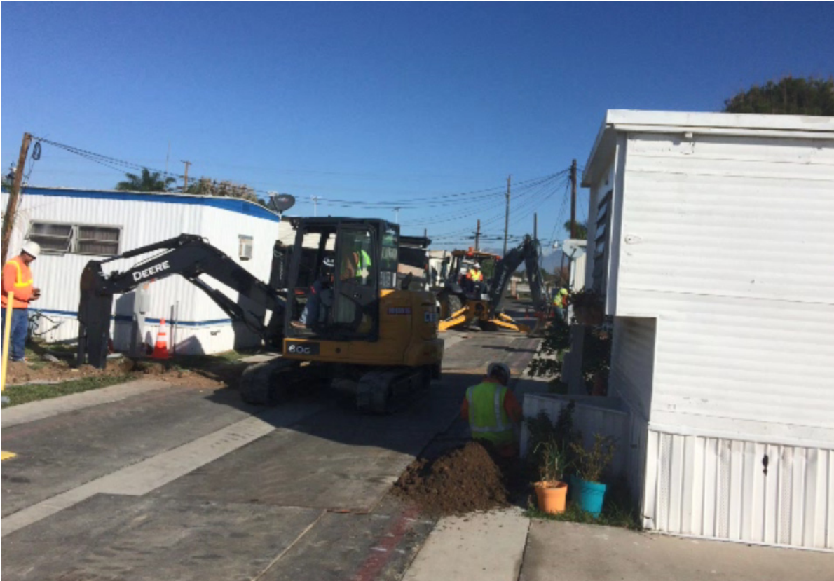
Fig. 4: Construction space limitations are common at mobilehome parks
