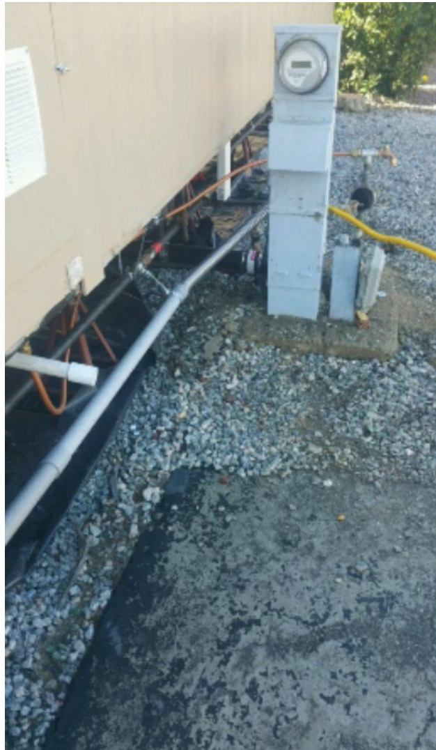
Fig. 6: Example of BTM service prior to conversion activities
