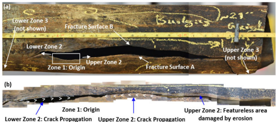
Figure 81: (a) Front and (b) Top Views of Fracture Surface B Identifying Zones 1 and 2
