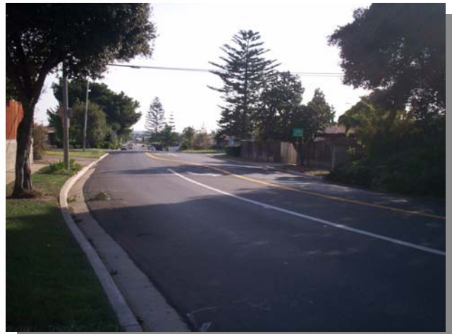
Johnson Avenue looking south from Swan Street at Project E13.
