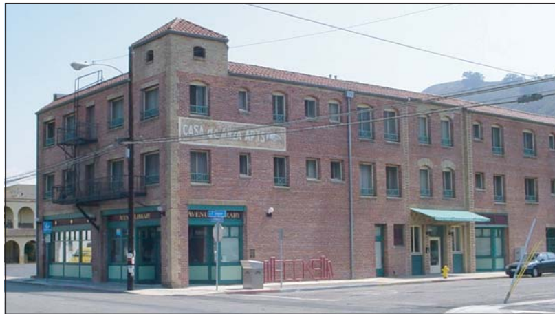
Photo 1 - Casa de Anza Apartment building on Ventura Avenue, with a ground floor library and apartments above. This is the type of intensification/reuse project anticipated for the Ventura Avenue corridor.
