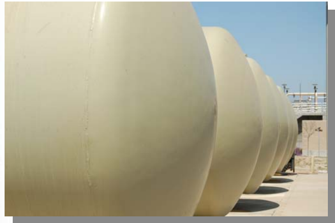
The existing mixed-media filters lack capacity to treat projected maximum day flows. A cloth media filter system is recommended to replace the existing tertiary filters.
