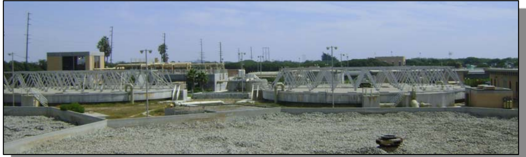
The Ventura WRF has two circular primary clarifiers, each with a diameter of 115 feet.
