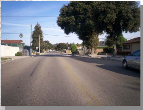
Maple Street looking east from College Avenue at Project E24.
