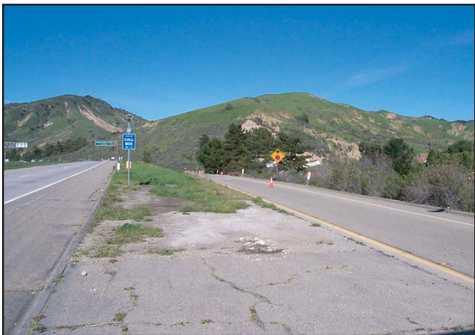
Photo 13 - Western Cañada Larga expansion area looking northeasterly from northbound SR 33. Portions of the hillside area fronting the freeway were graded for the construction of SR33 and could potentially be re-graded and developed if this expansion area is selected.
