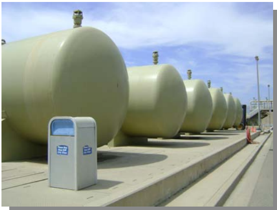
Six mixed-media filters are used for tertiary treatment.
