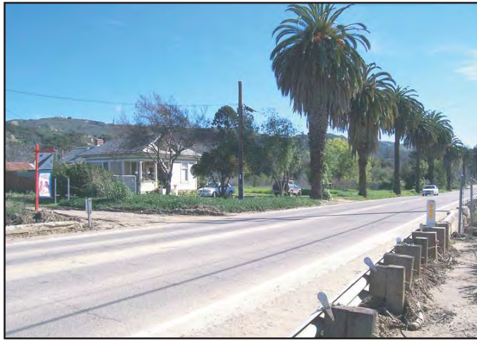
Photo 11 - North Avenue expansion area looking southeasterly from Ventura Avenue. The entire expansion area is visible to travelers on Ventura Avenue.
