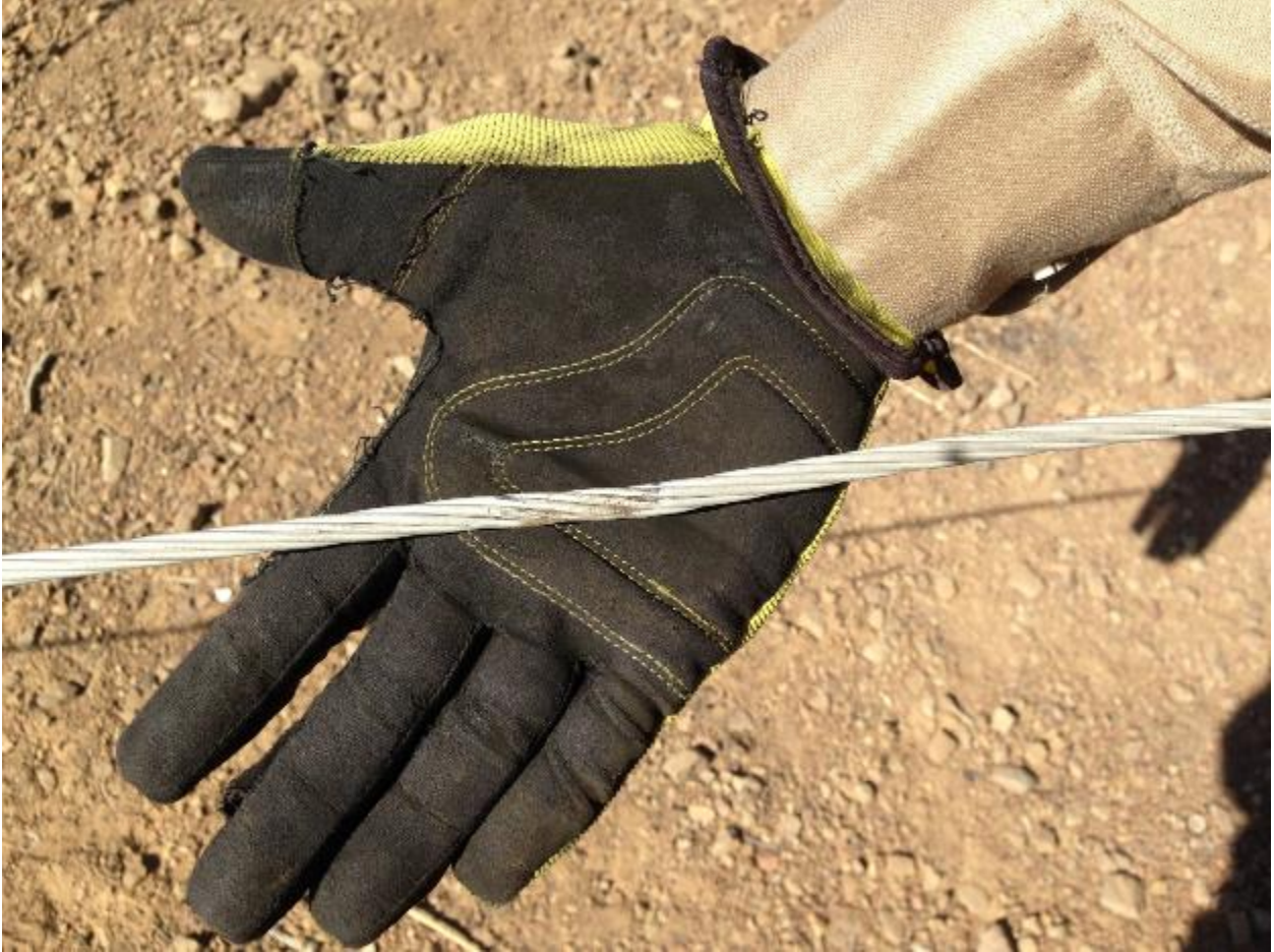
Figure 12: Edison photograph depicting damage on the center conductor between poles numbered 1025341E and 1202085E. 63
