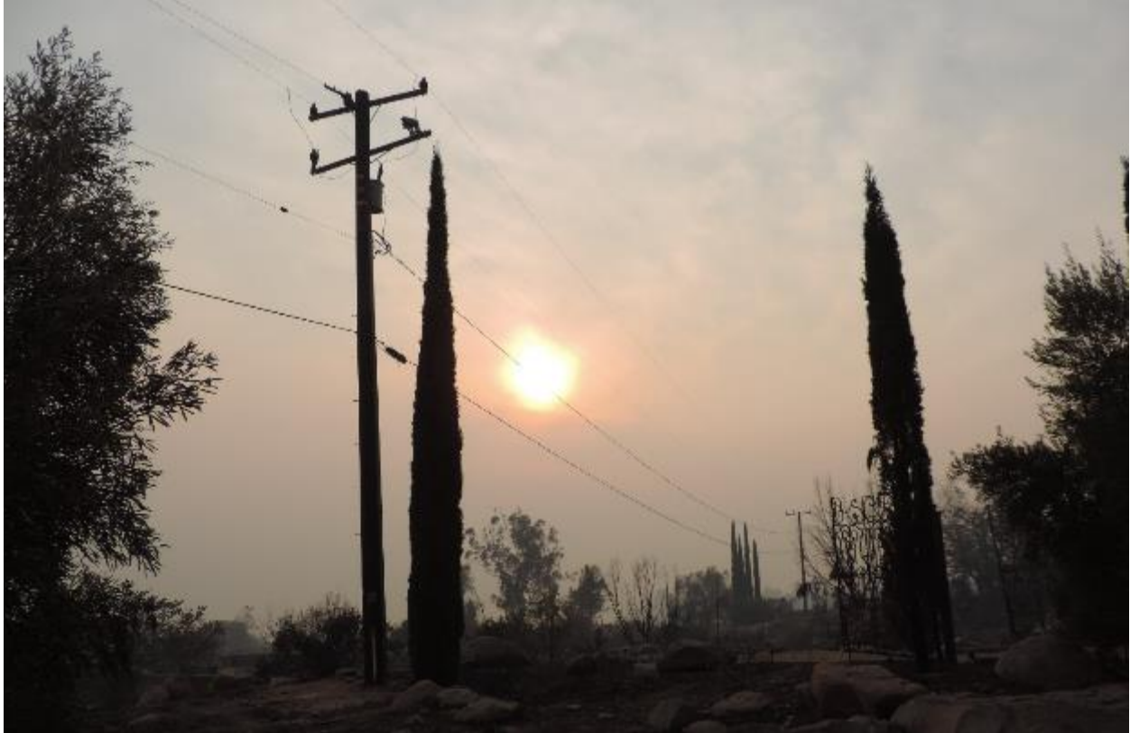
Figure 2: SED photo Koenigstein site, 729566E at the fore, 729565E at the rear.
