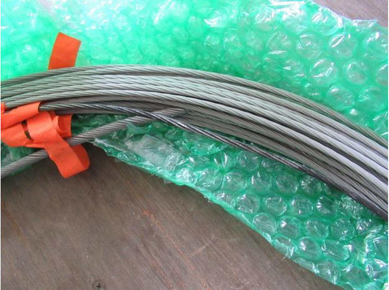
Figure 13: SED photo of February 2017 Anlauf Canyon evidence examination, damage on the east conductor between poles numbered 1025341E and 3002114E.
