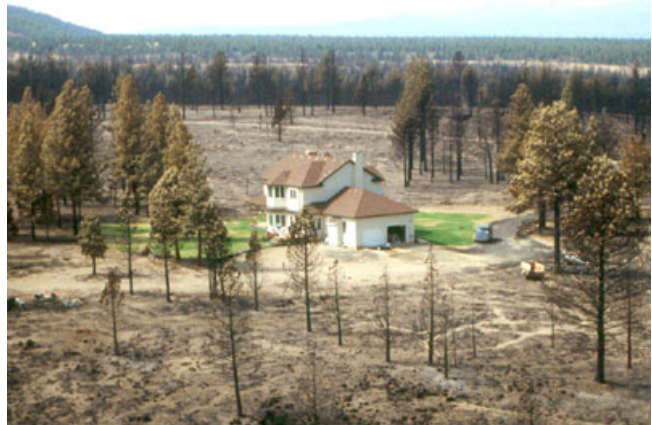
Home surrounded by wildland that survived a fire due to good defensible space.
