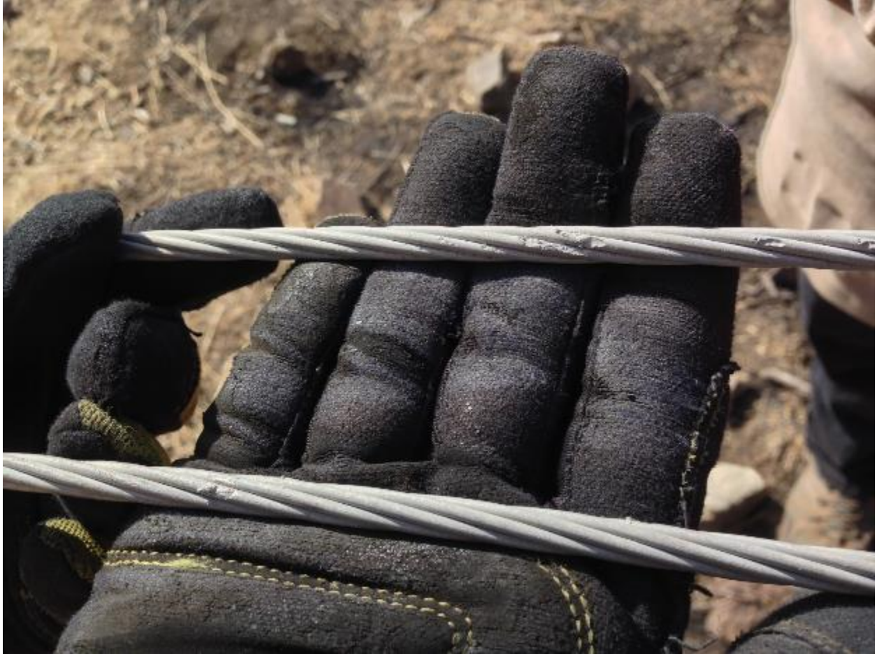
Figure 11: Edison photograph depicting damage on two unidentified adjacent conductors between poles numbered 1025341E and 3002114E. 62
