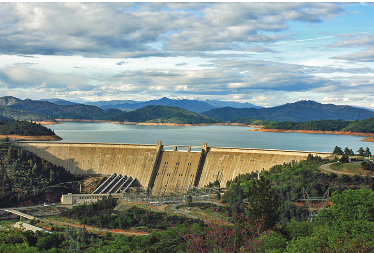
The Shasta Dam is one of California's two largest, with a storage capacity of 4.55 million acre feet. Photo credit: Apaliwal 2009.
