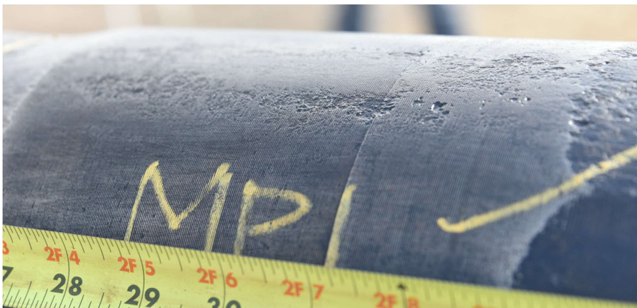
Figure 28: Shallow Metal Loss on Connection C014
