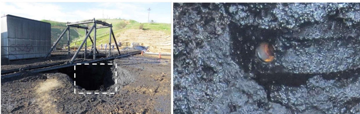
Figure 18: Photos of Missing 11 3/4 in. Casing Valve Taken on February 25, 2016
