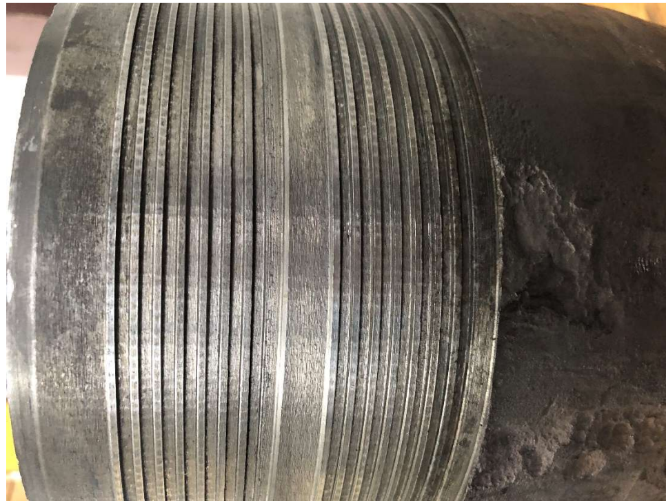
Figure 78: Pin and Box from Leaking Connection C023A1C
