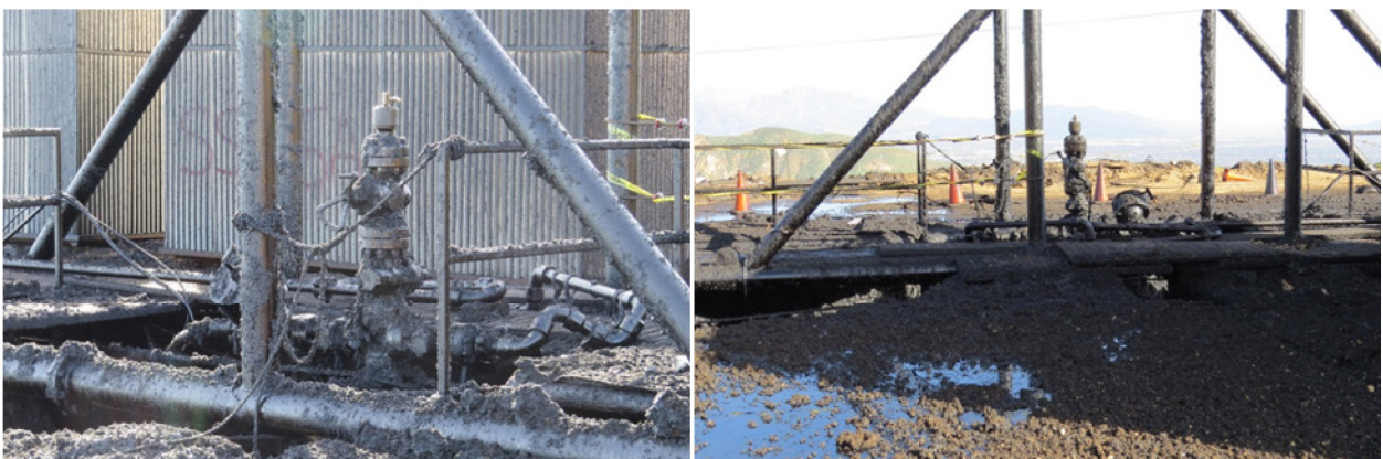
Figure 18: SS-25 Wellhead in February 2016
