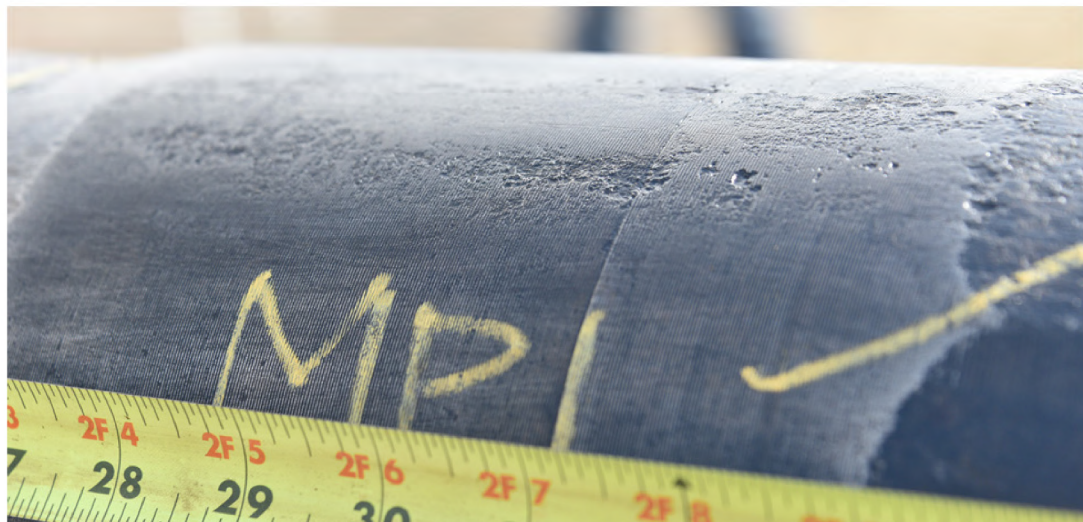
Figure 53: Shallow Metal Loss on Connection C014
