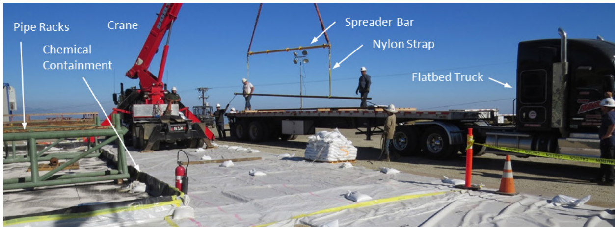
Figure 30: Unloading of Tubing at the PS-20 Site
