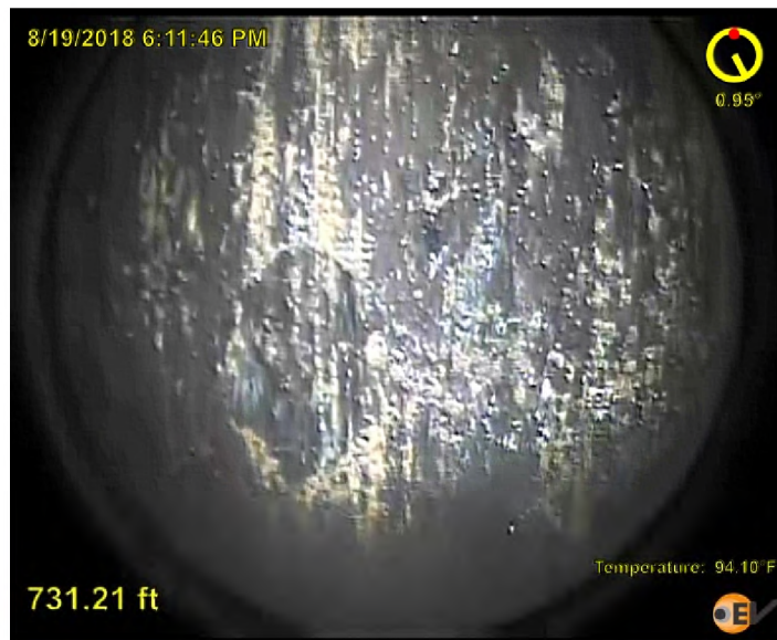
Figure 70: EV Camera Snapshot of ID Corrosion on 11 3/4 in. Casing
