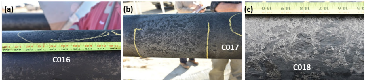
Figure 55: Pipe Body Corrosion on (a) C016, (b) C017, and (c) C018
