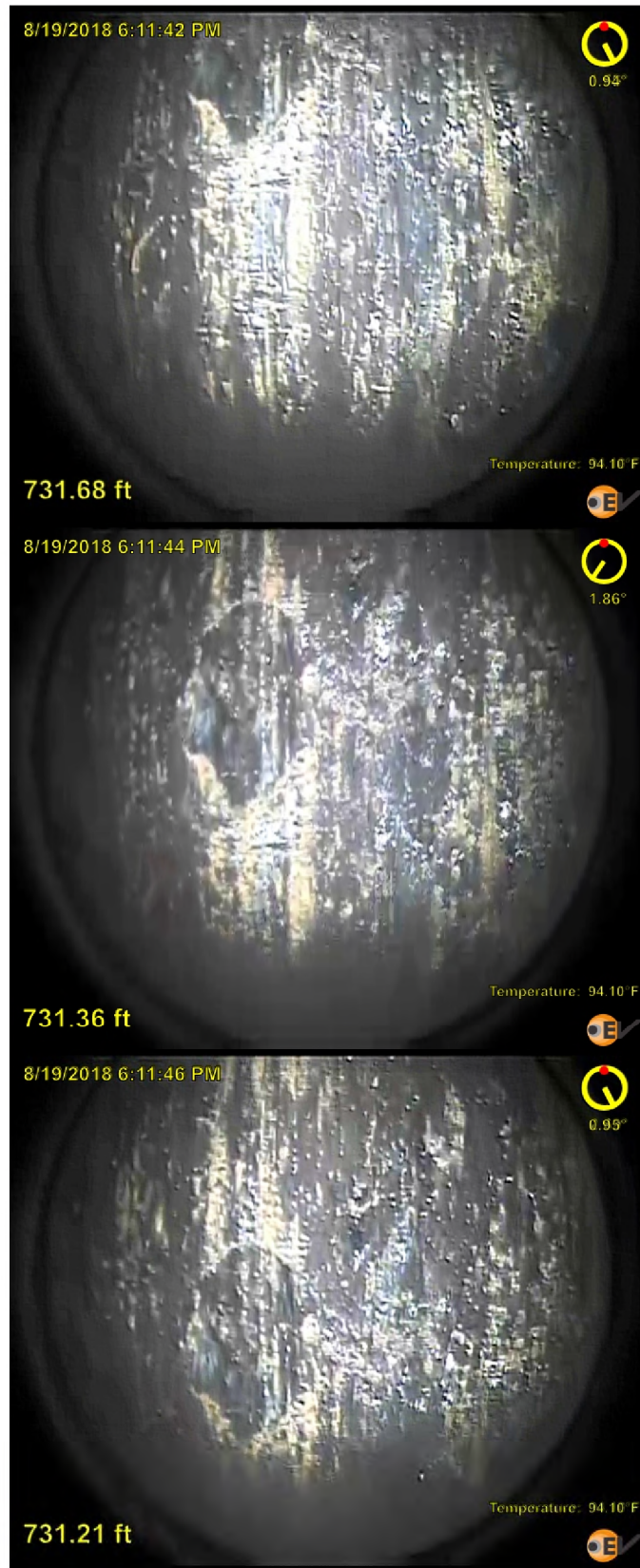
Figure 43: 11 3/4 in. Video Imaging at ~731 ft, Example of Pitting Observed
