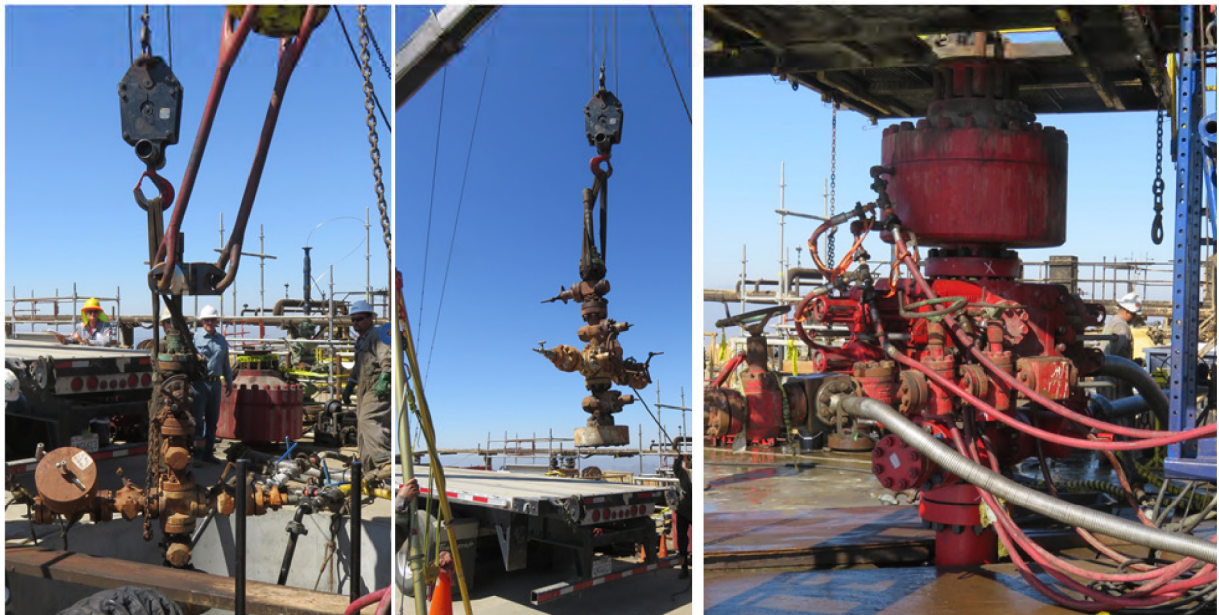
Figure 21: SS-25 Tree Removal and Blowout Preventer Installation
