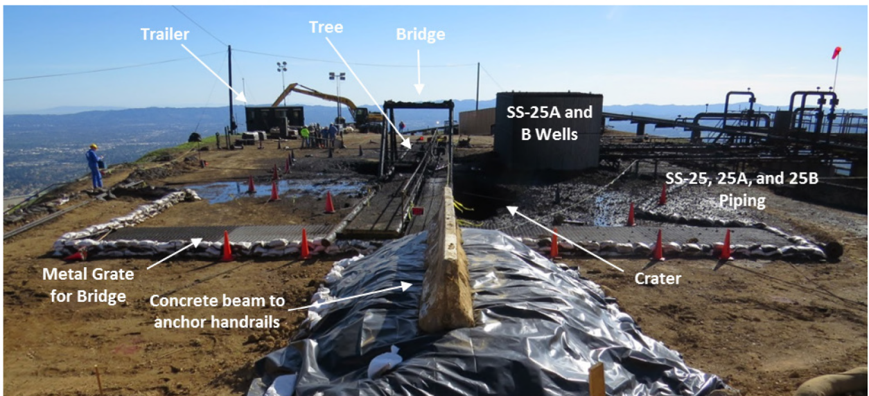
Figure 9: SS-25 Site Condition on February 25, 2016
