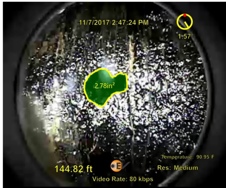
Figure 32: SS-25 Surface Casing Hole at 145 ft MD
