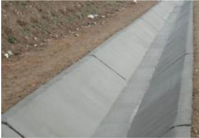
Figure 2: Site Concrete Drainage Ditch
