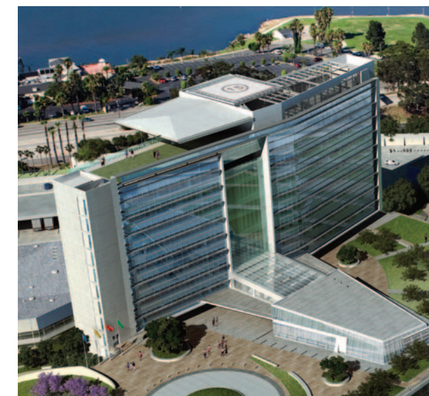
Port of Long Beach Photograph courtesy of Gensler, Santa Monica
