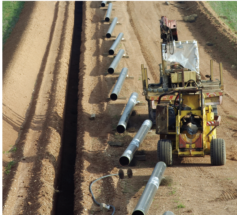
Natural gas pipeline sections are arrayed along a trench before being welded together.
