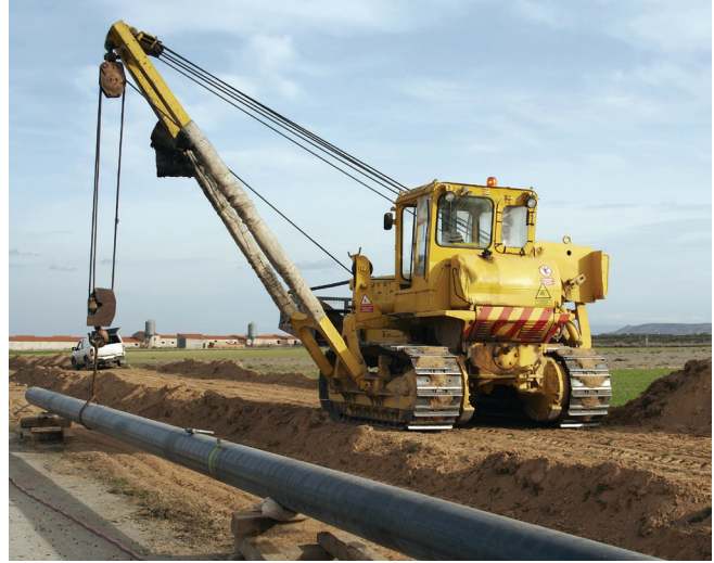
A crane lifts welded pipeline sections so more can be added.
