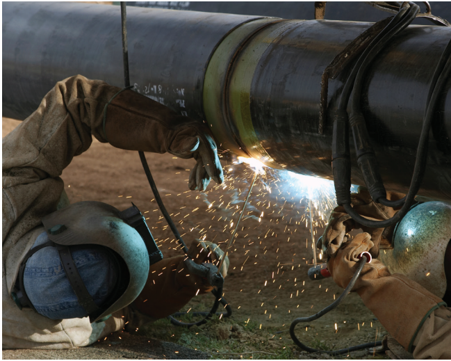
Workers carefully weld two pipeline sections together.
