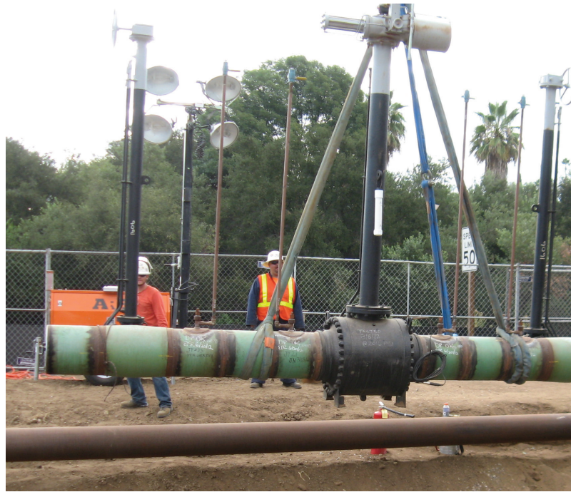
A valve in a pipeline section with an actuator on an extension stem in the process of being installed.
