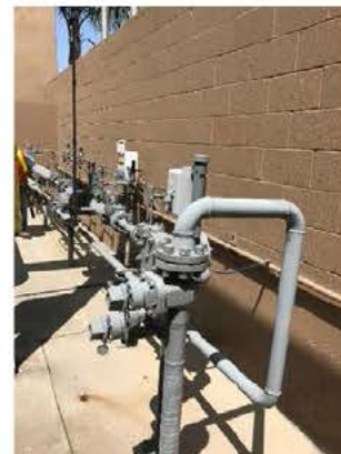
Industrial and Commercial Meter Sets
