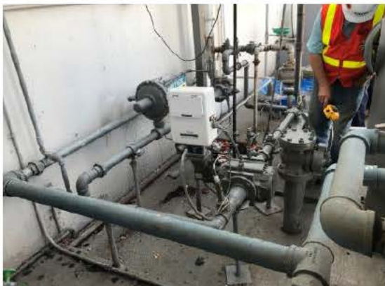
Industrial and Commercial Meter Sets
