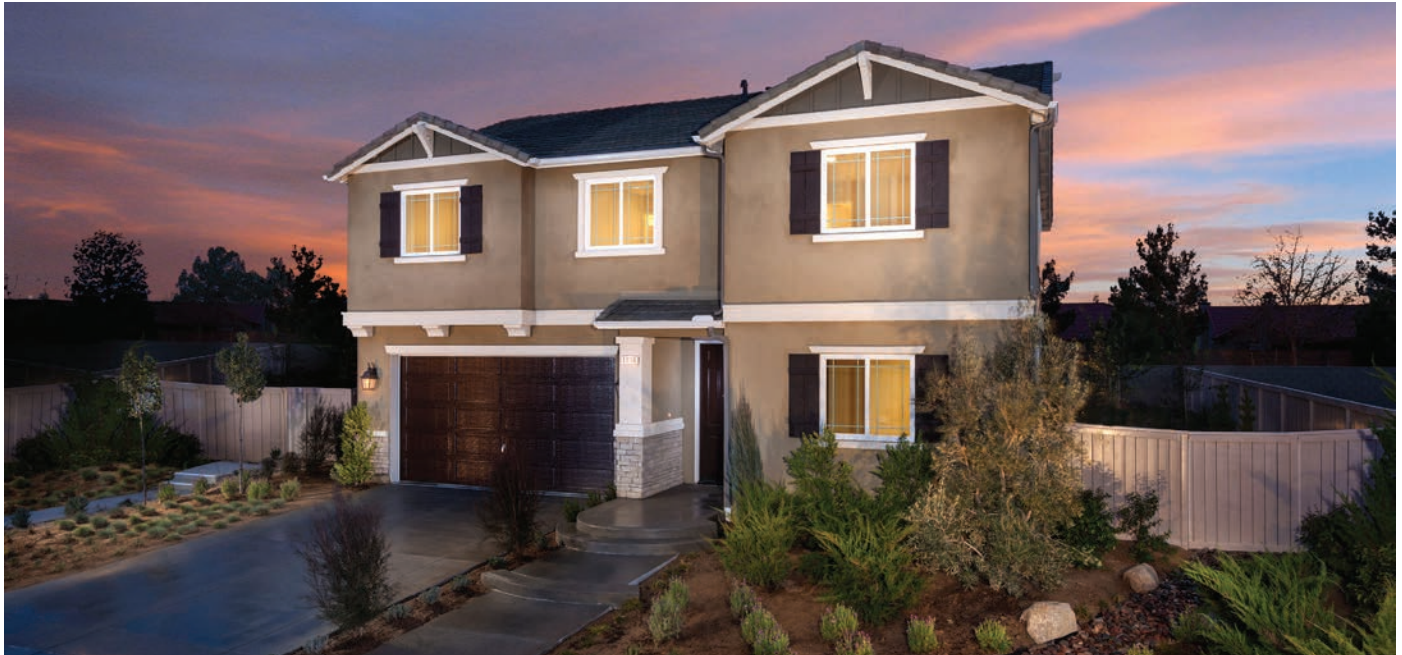
Innovation Goes Green: Sustainable design in a home that is functional, affordable and beautiful.
