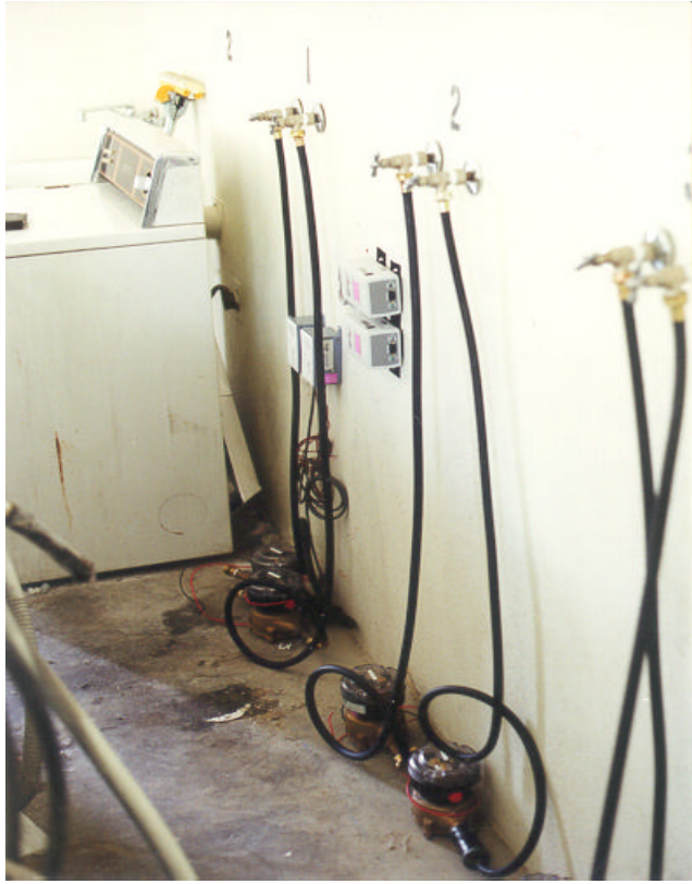
Figure B.5.1 Metering Equipment Installed at Leisure World Laguna Woods
