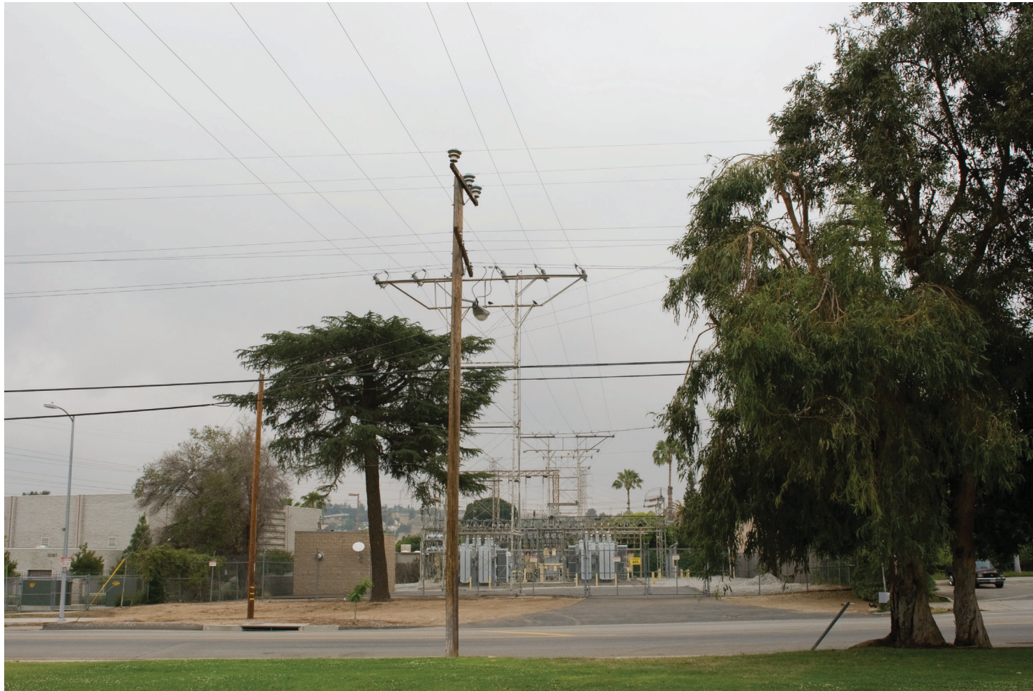
View Point 10 Existing Conditions: San Fernando Substation from Brand Park (Facing Northwest)
