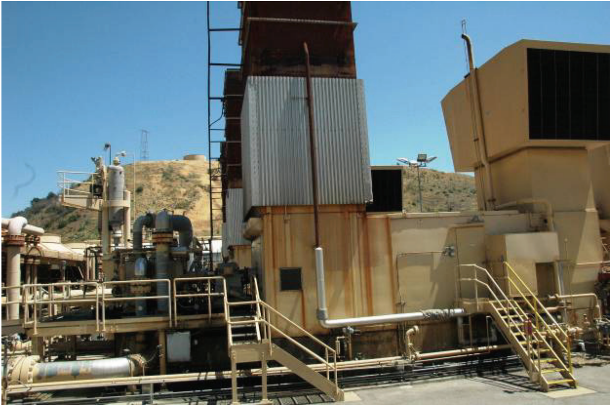
Figure 2 –Complete TDC from left to right: Compressor, gear, exhaust stack, LM1500 housing, air inlet.
