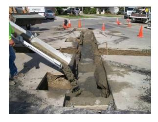
Hand Backfill - Typically one day and paving could be done same day, at lower labor cost
