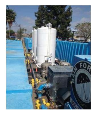
Figure 12: Hydrotest Set Up with Sound Proofing to Minimize Noise Complaints (located behind Baker tank)
