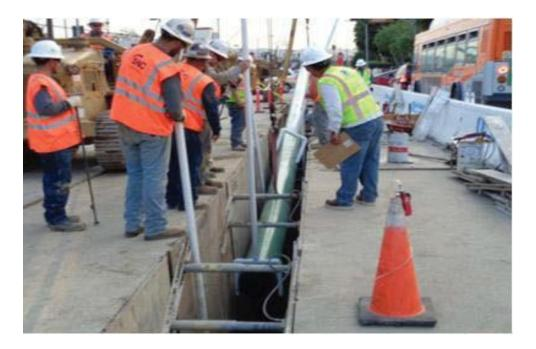
Figure 3: Installing Pipe in Trench with Existing Substructures
