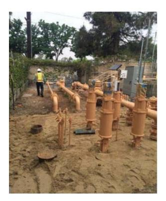
Figure 18: Large Valve Station with Numerous Above-Ground Features
