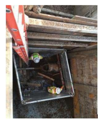
Figure 8: Jack and Bore Operation
