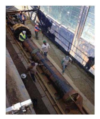
Figure 9: Lowering Section of Pipe into Trench
