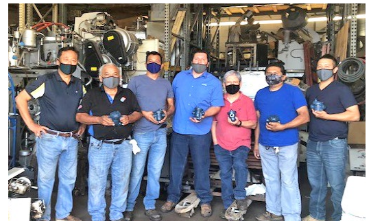
The Cleaner's Mart helps dry cleaners reduce their energy usage and costs by installing new steam traps, which remove condensate and air, while minimizing steam loss, in steam heating systems.
