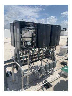
What is a Tankless Rack System? A single, self contained system consisting of multiple tankless units which replaces one larger heat source. Three key advantages are:
