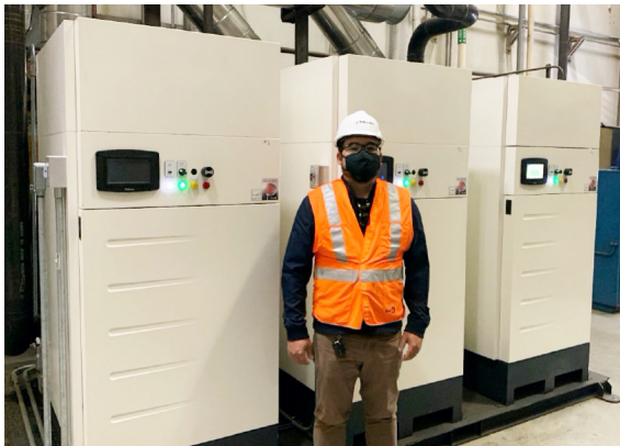
R.F. MacDonald replaced an old firetube boiler with three new high efficiency condensing boilers at a metal beverage container manufacturer.
