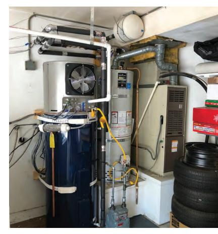
GTI field-tested 4th-generation gas-fired heat pump water heater prototypes in five single-family homes in the Los Angeles basin.
