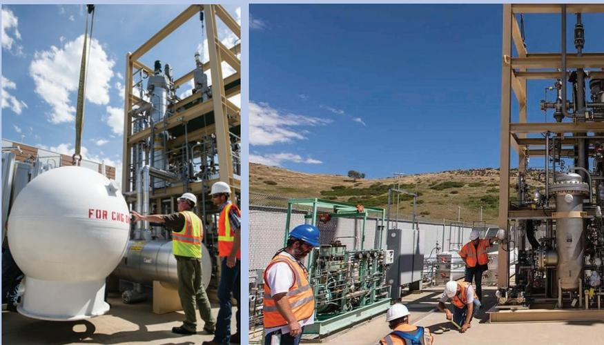
Recently, SoCalGas worked with DOE's National Renewable Energy Laboratory (NREL) and Electrochaea GmbH—a University of Chicago technology spin-off focused on converting low-cost and stranded electricity and carbon-dioxide into pipeline-grade RNG—to build the nation's first scalable renewable hydrogen biomethanation reactor system at the NREL Energy System Integration Facility in Golden, Colorado.
