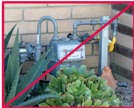
INADEQUATE WORKING SPACE
