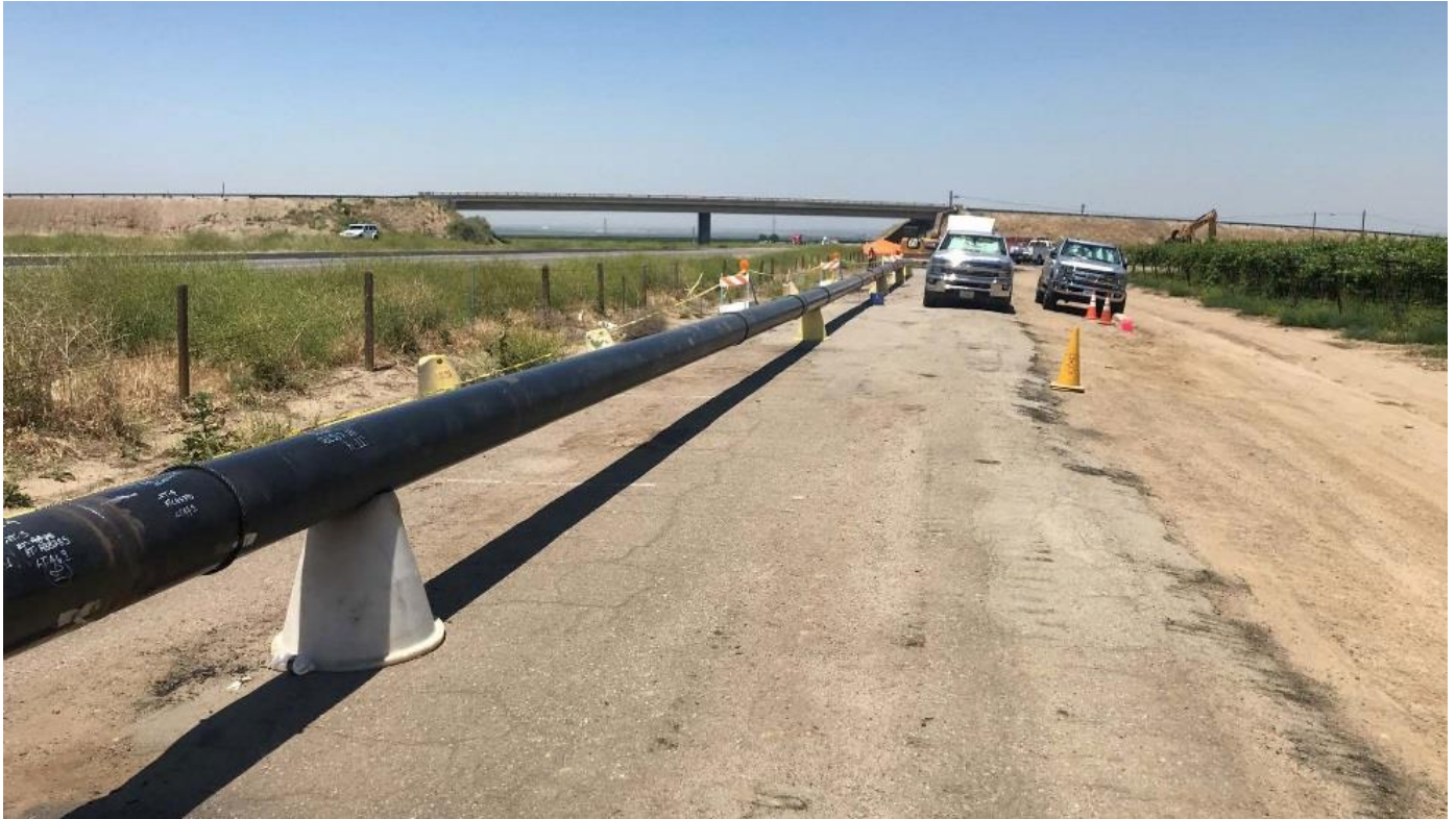
Figure 5: Pipe Prepared for HDD under Sabodan Street
