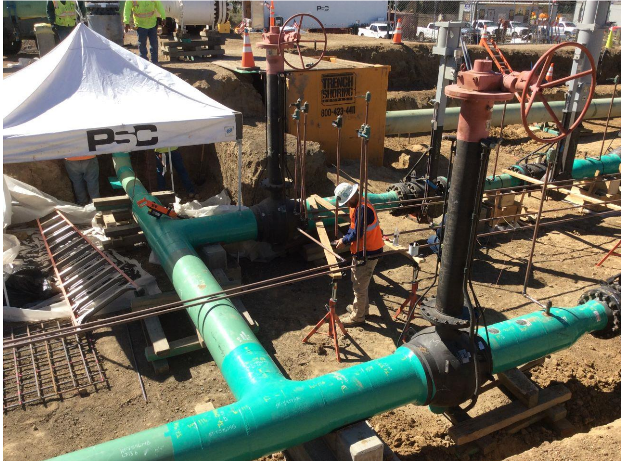
Figure 2: Applying Cathodic Protection Wrap
