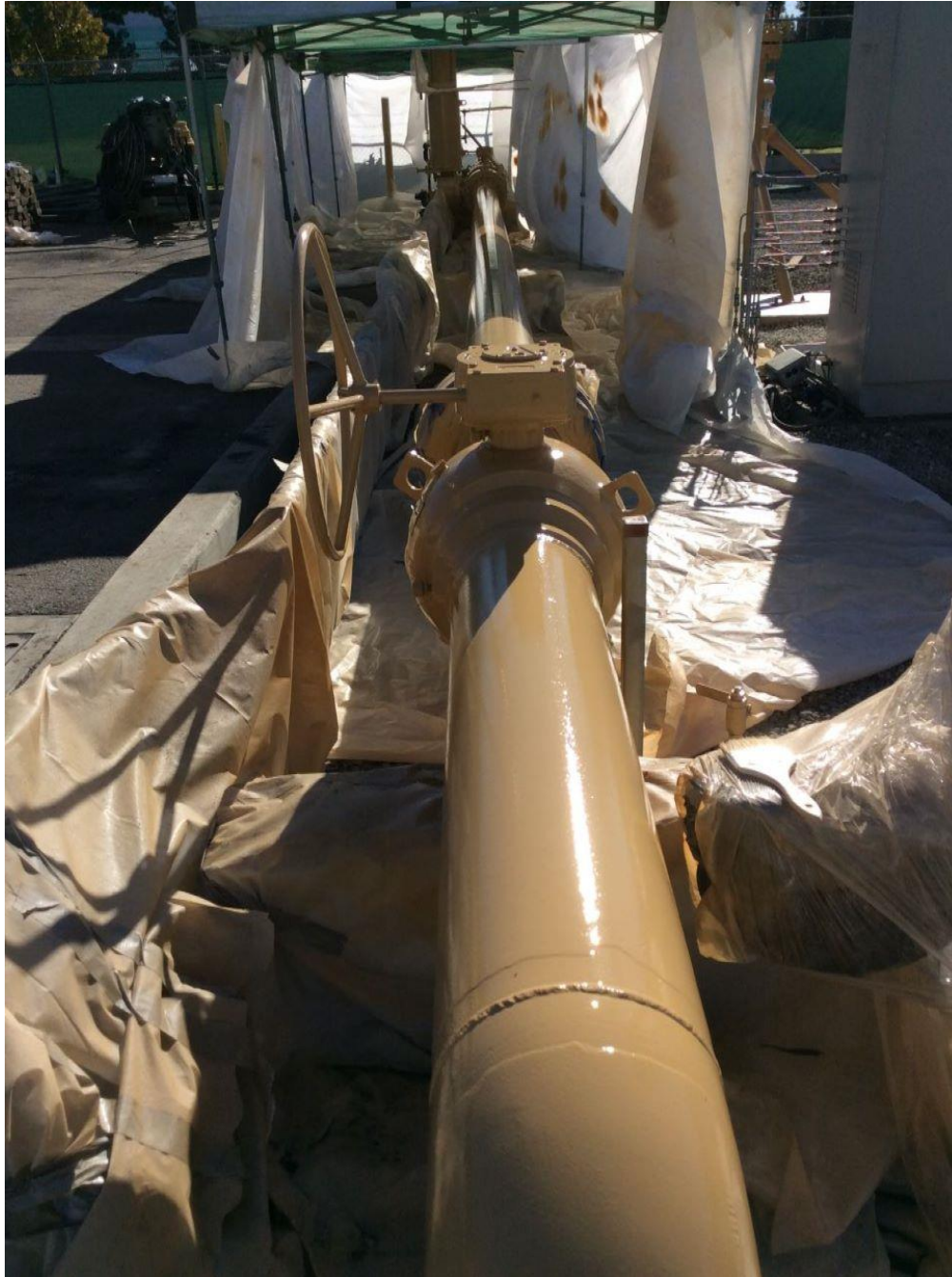
Figure 3: Newly Coated Pipeline
