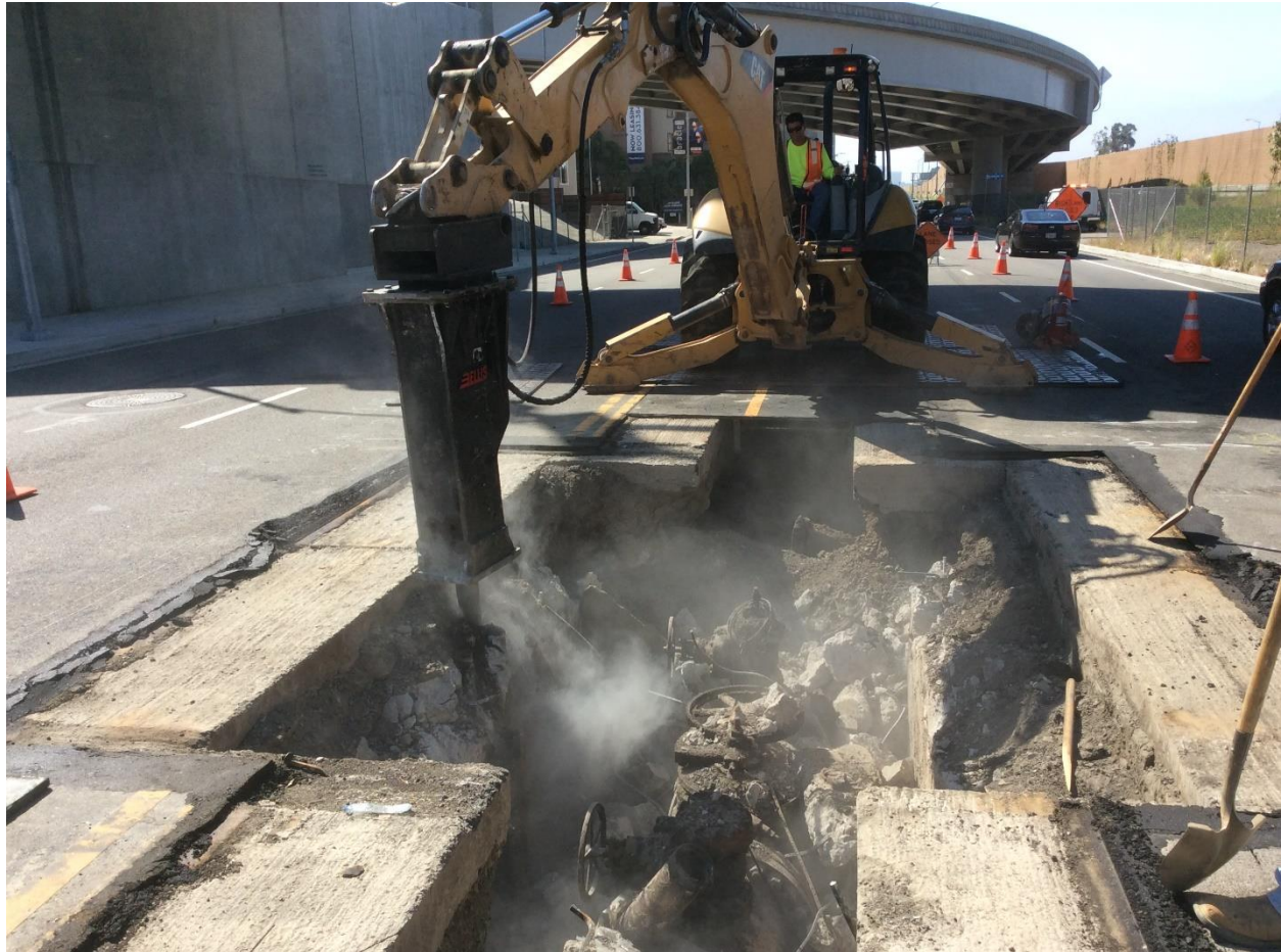
Figure 9: Demolition of a Concrete Vault
