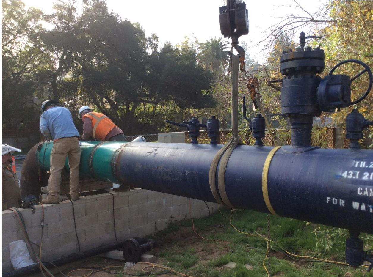
Figure 3: Installing Test Head
