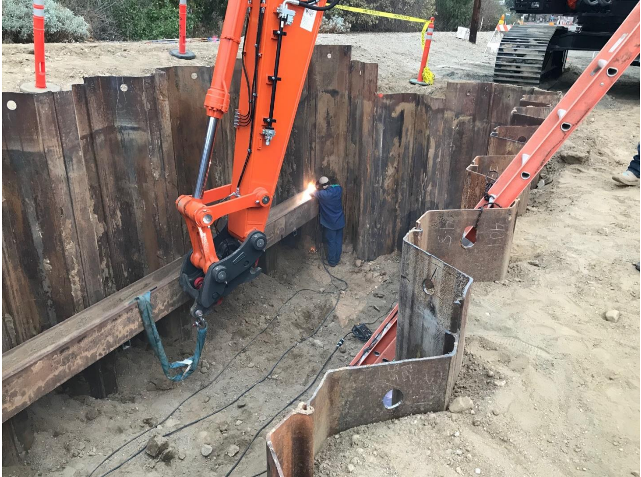
Figure 5: Welding Support Beams for Entry Bore Pit
