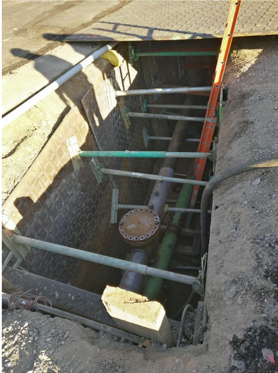
Figure 4: PCF Connecting the Old and New Pipeline
