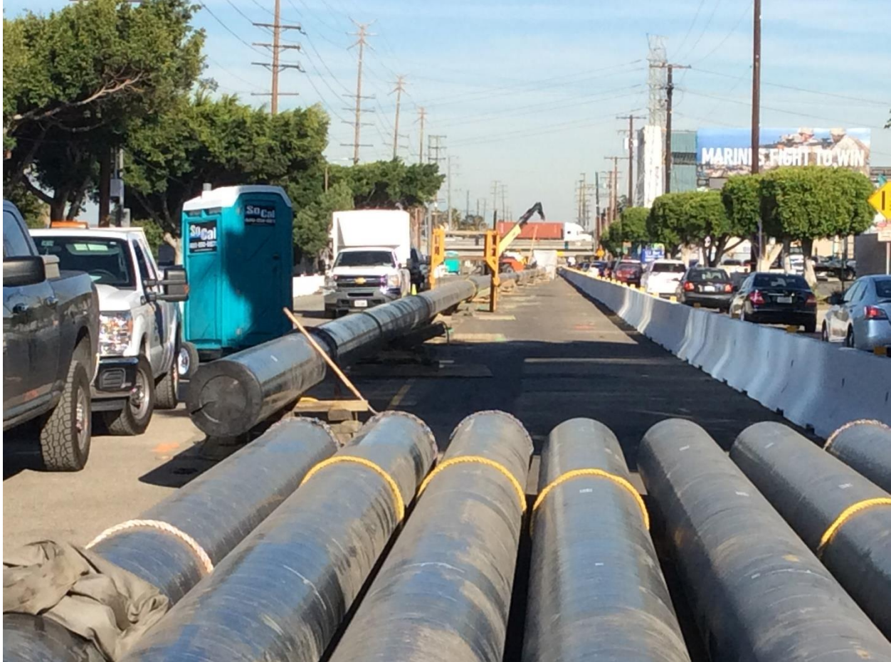
Figure 5: Preparing for Horizontal Directional Drill Pullback
