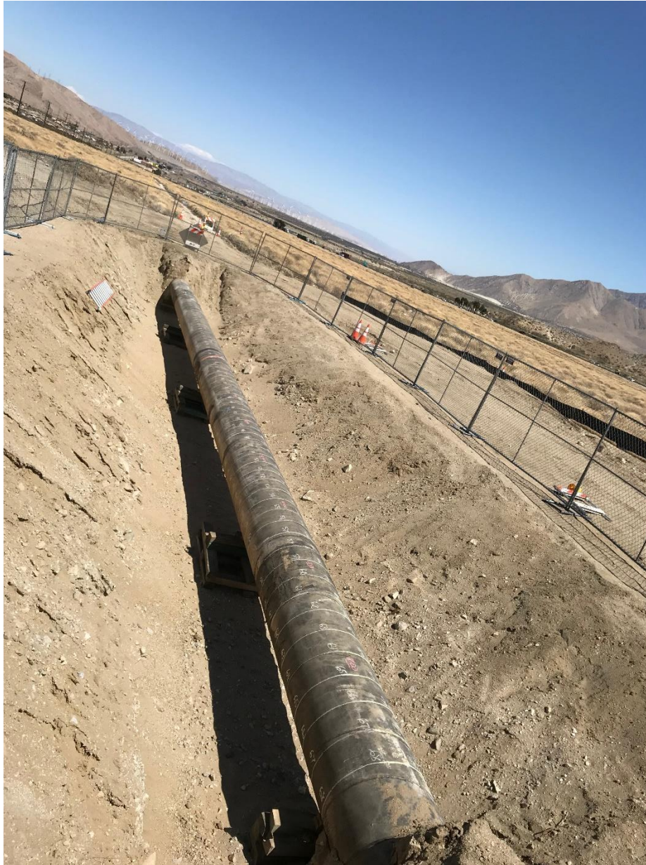
Figure 8: Excavated Leak Location
