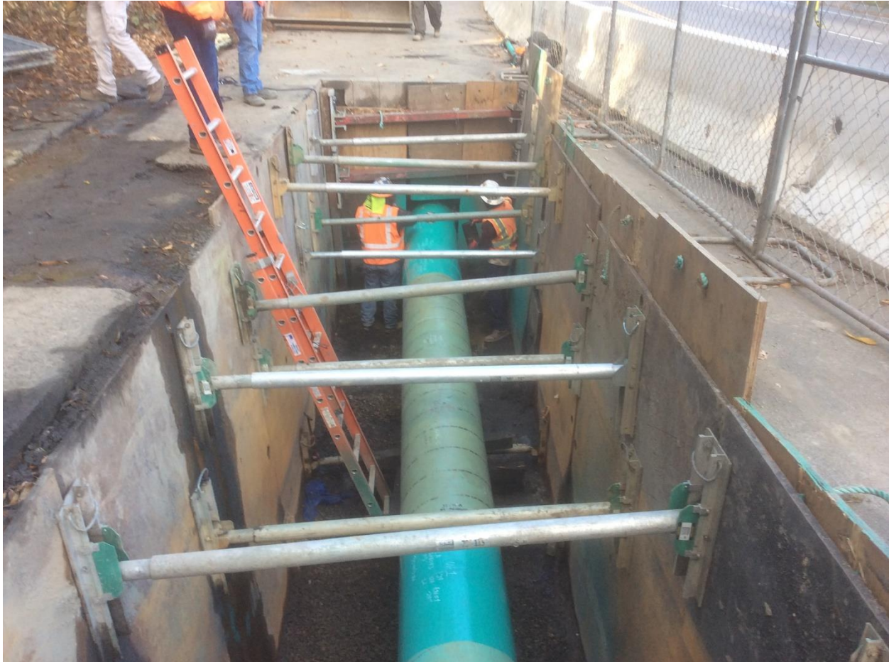
Figure 4: Prepping for Slurry and Backfill
