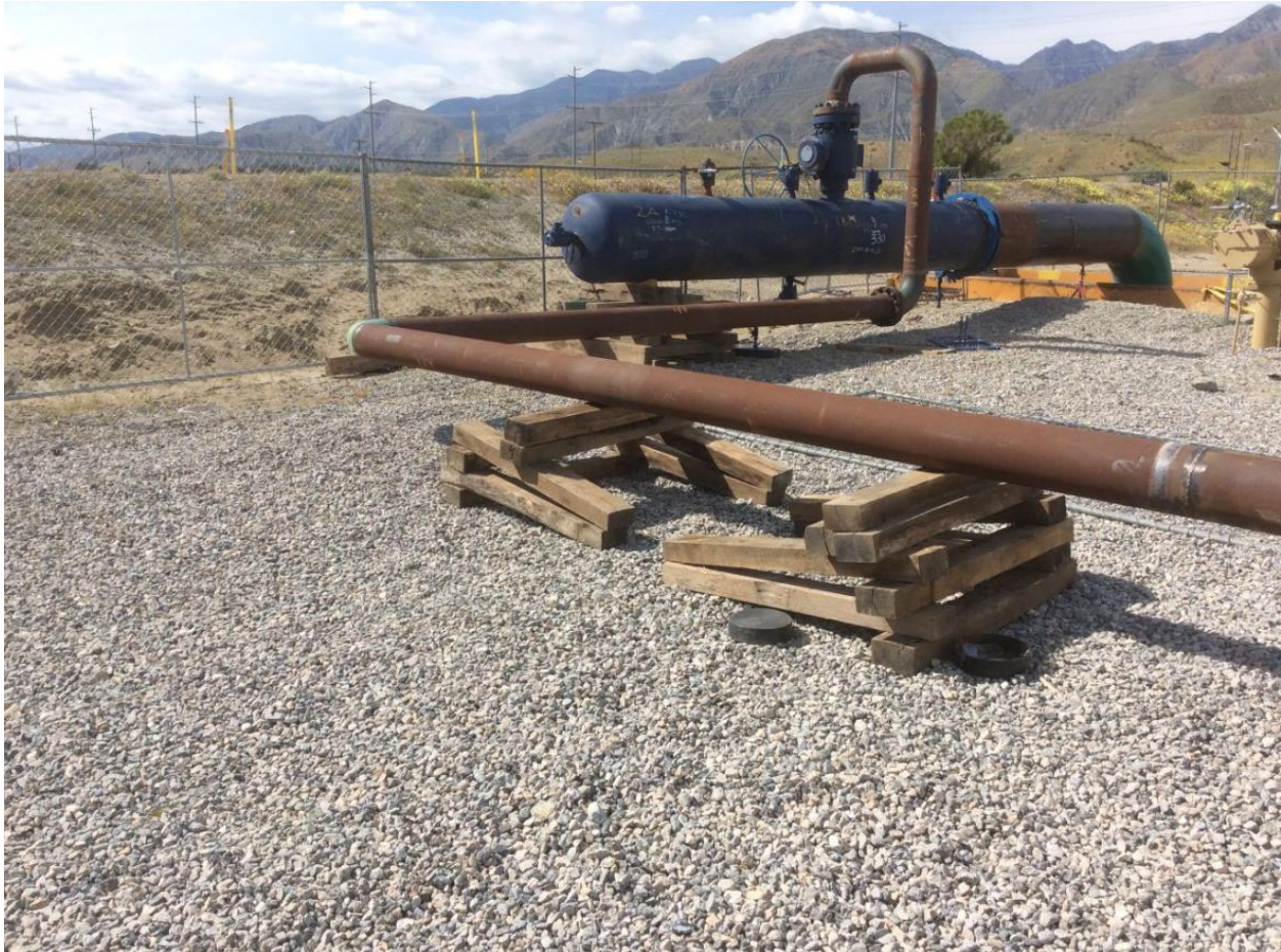
Figure 4: Test Head Water Pipe
