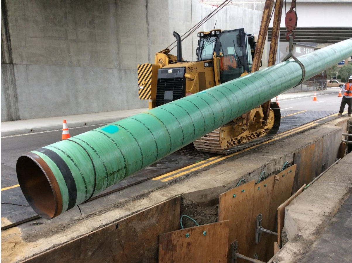
Figure 10: Lowering in of New Pipe
