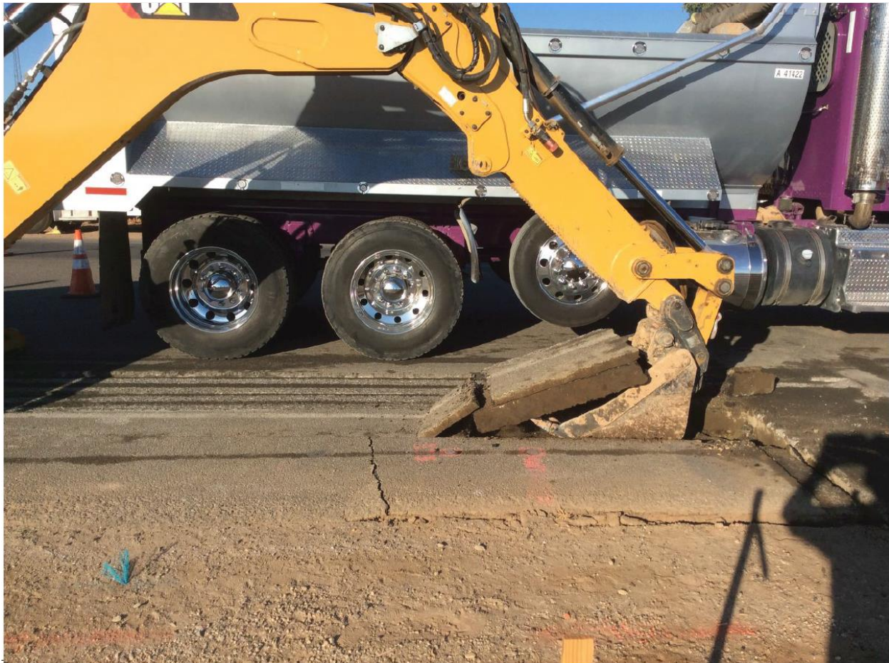
Figure 3: Excavation and Removal of Asphalt
