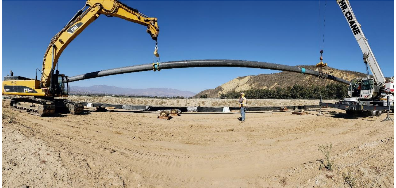
Figure 5: Horizontal Directional Drill Pullback
