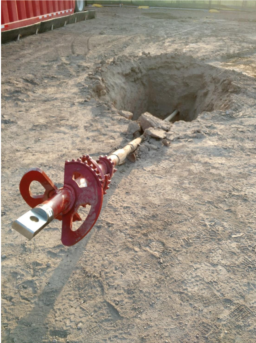
Figure 6: Back Reamer for HDD
