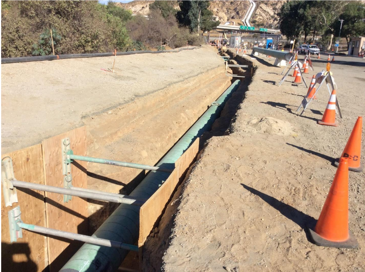
Figure 6: New Pipe Lowered into Trench
