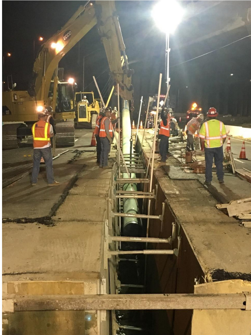
Figure 12: Lowering in New Pipe
