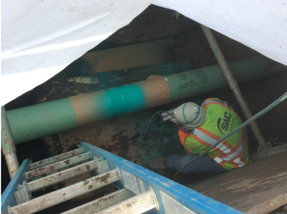
Figure 9: Applying Epoxy Coating to New Pipeline
