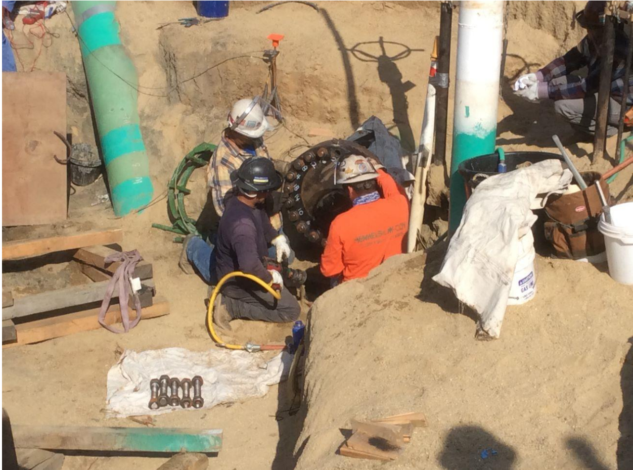
Figure 3: Bolting up Blind Flange
