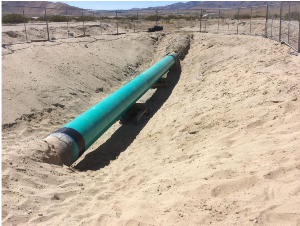
Figure 7: Feature Repair and Recoating
