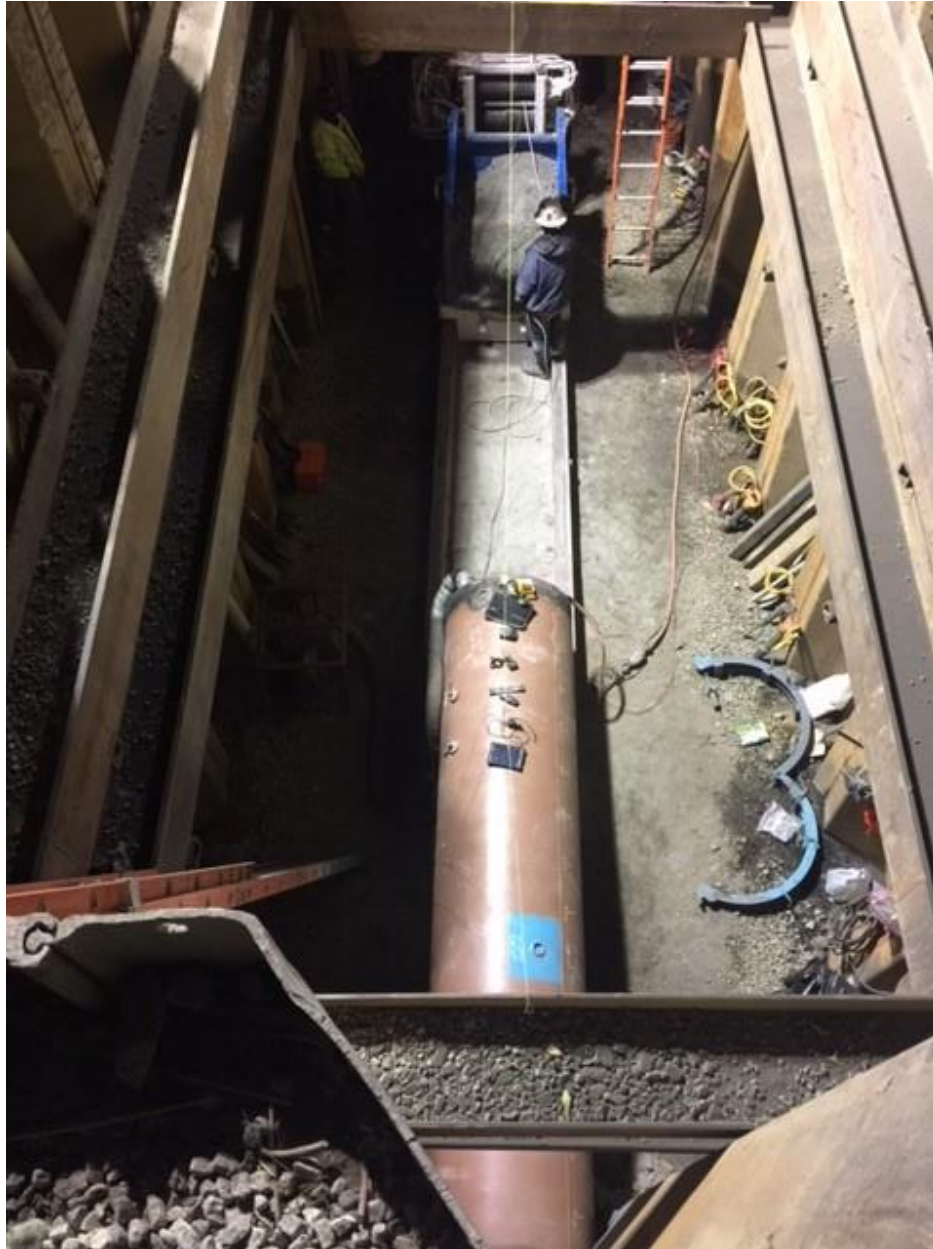
Figure 13: Bore Casing for Interstate 5 and Metrolink Crossing
