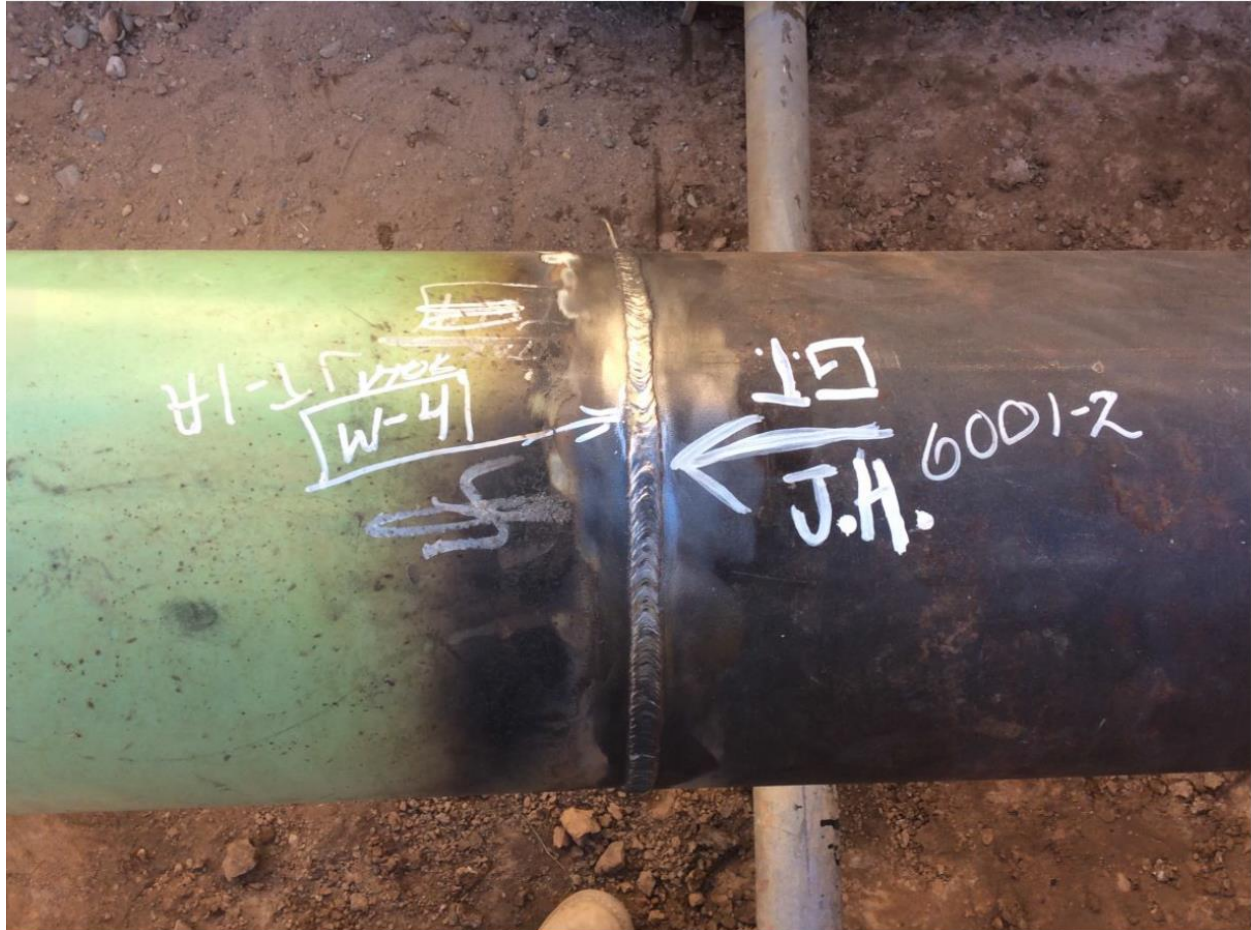
Figure 5: Tie-in Weld
