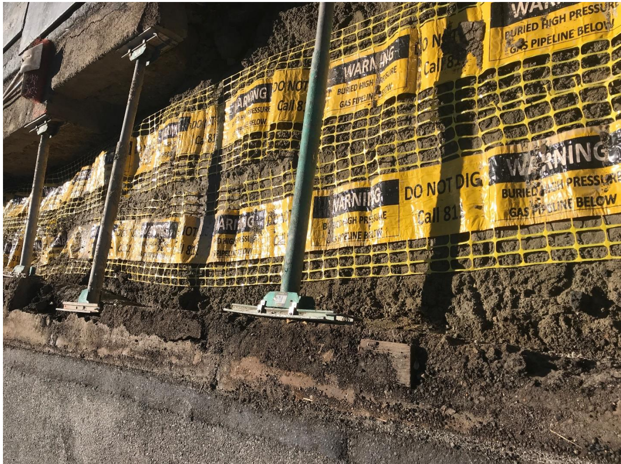
Figure 13: Pipeline Warning Tape
