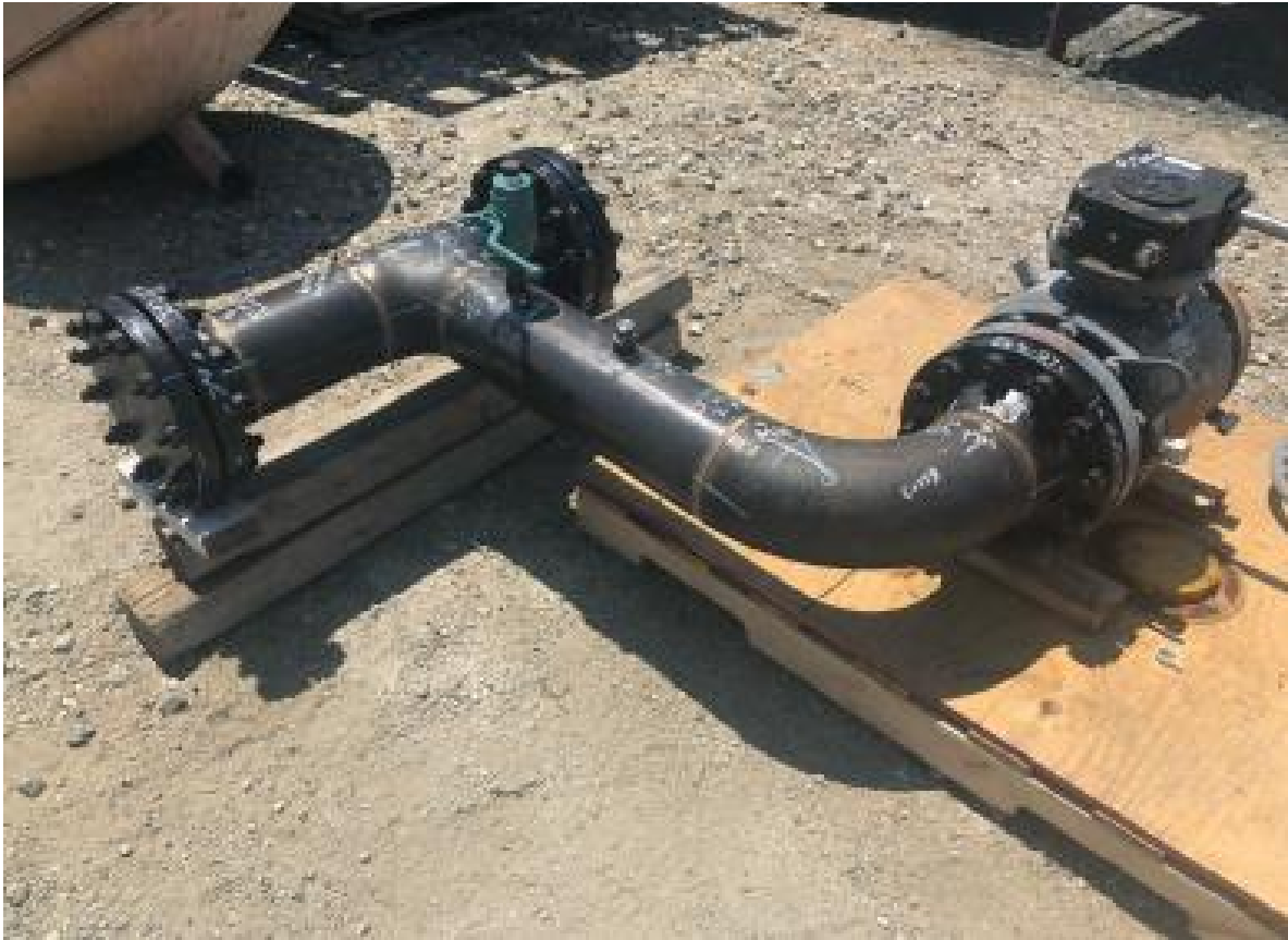
Figure 4: Prefabricated Assembly for Regulator Station
