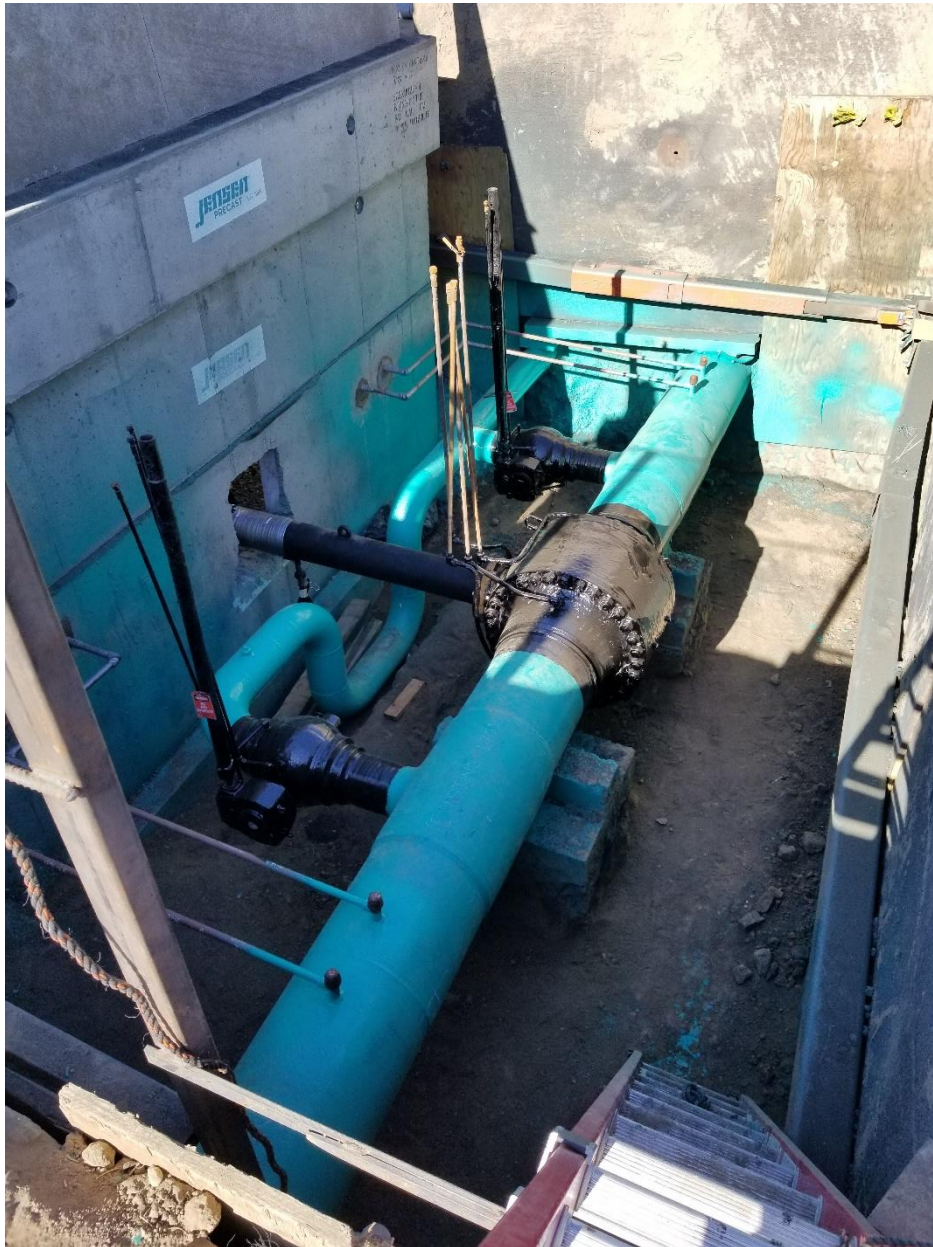
Figure 4: Excavation Around Existing Valve Assembly
