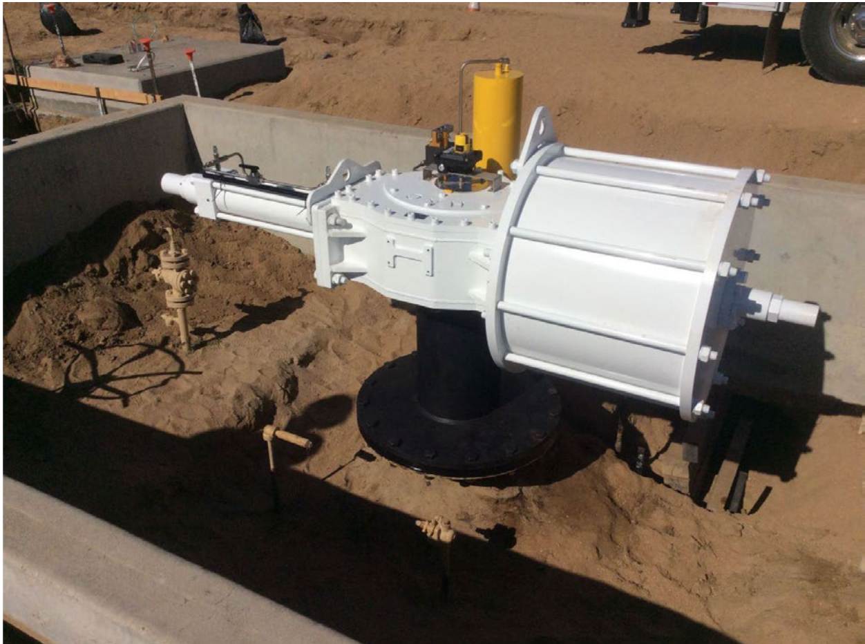
Figure 4: New Actuator
