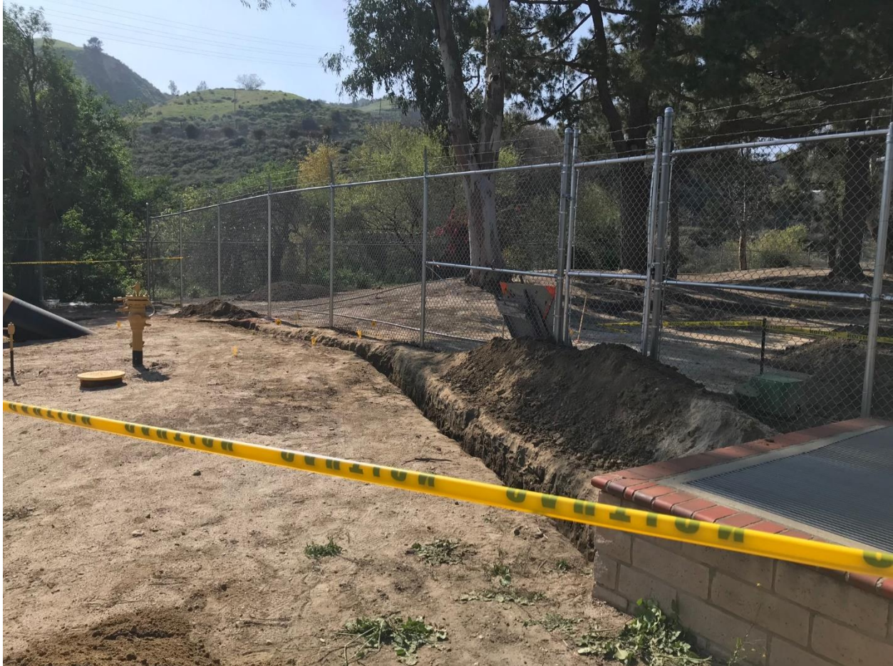
Figure 4: Trench for Conduit Run
