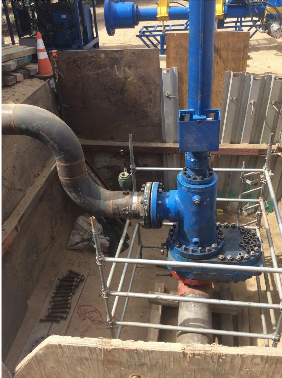
Figure 4: Stopple Fitting with Temporary Bypass
