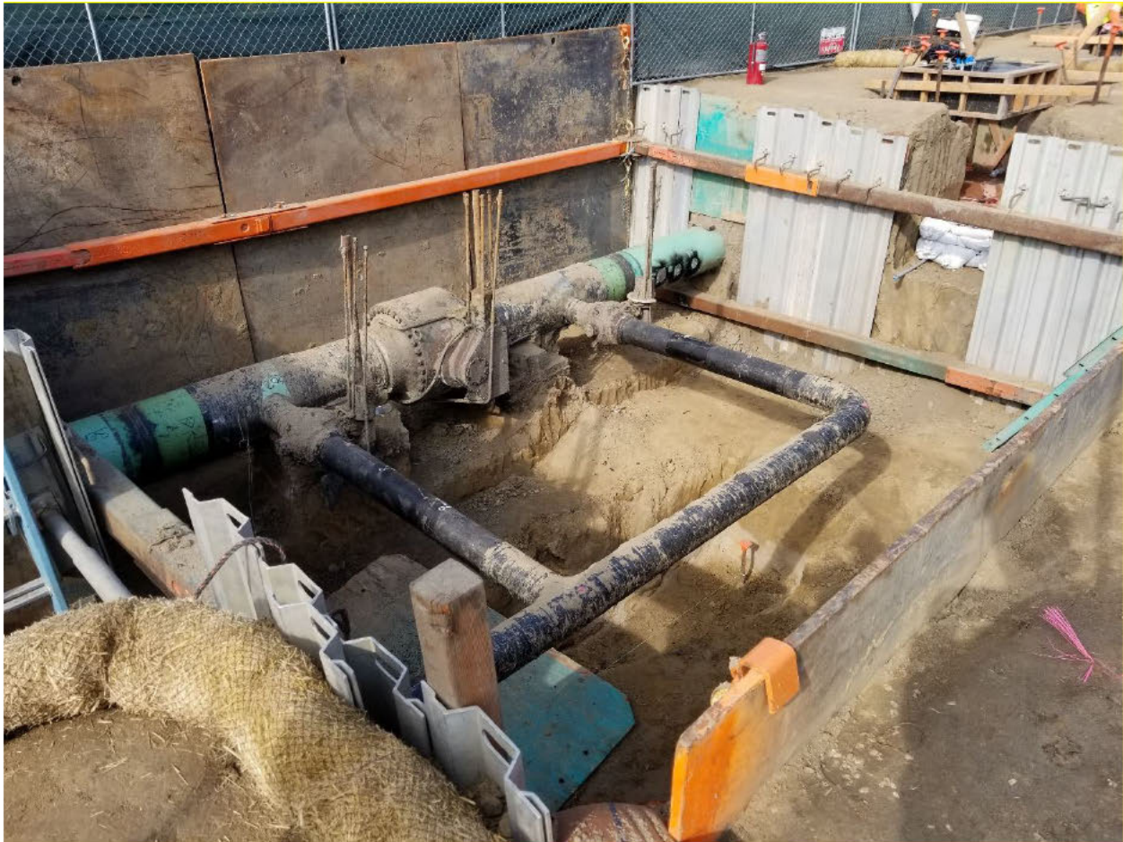
Figure 4: Excavation around Mainline Valve Assembly
