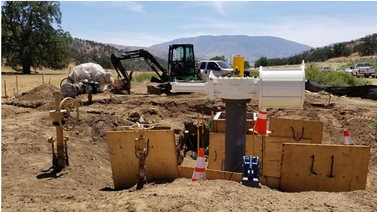
Figure 4: New Actuator and Excavation for Instrument Taps
