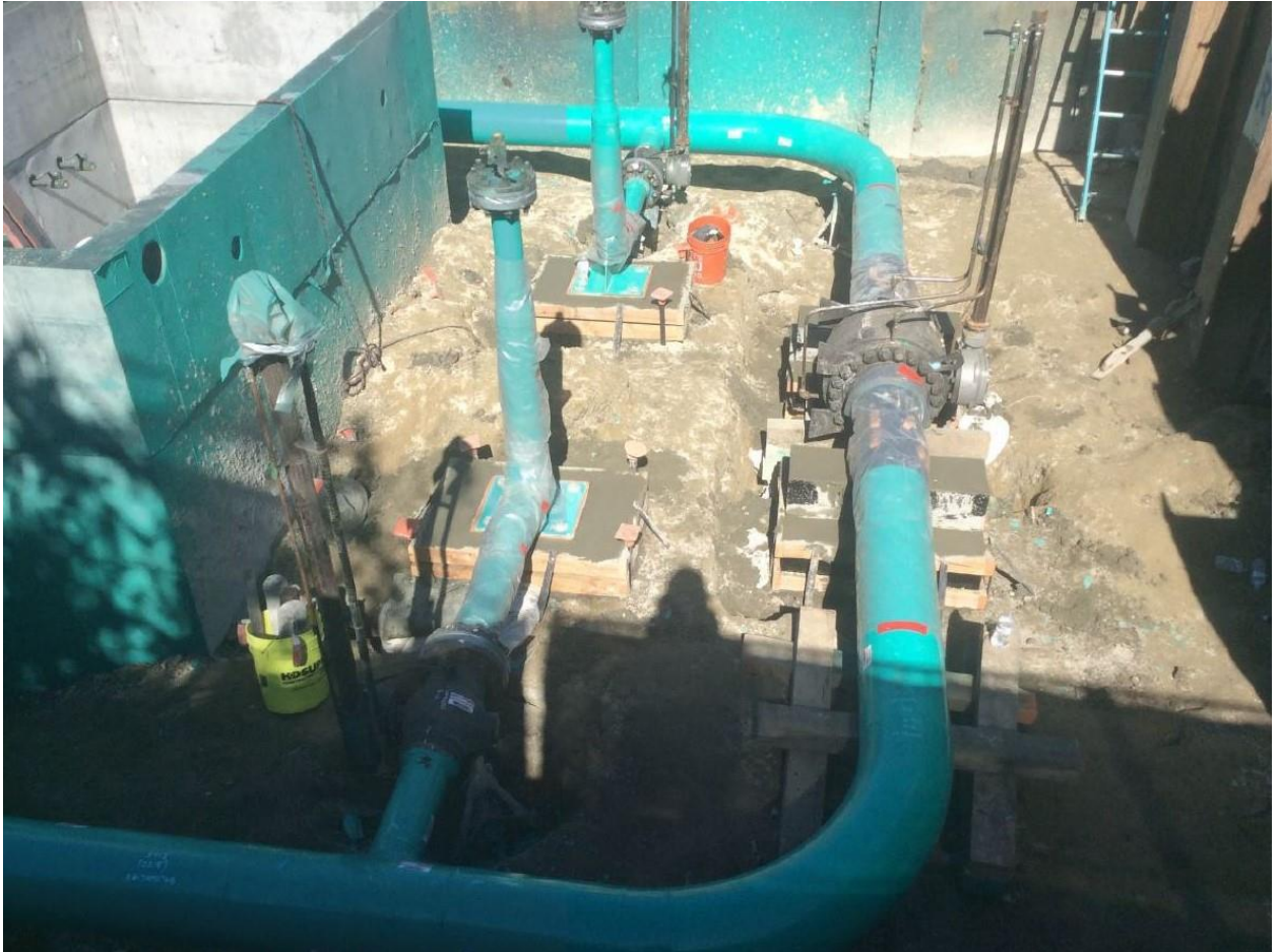
Figure 4: New Valve Assembly and Concrete Supports
