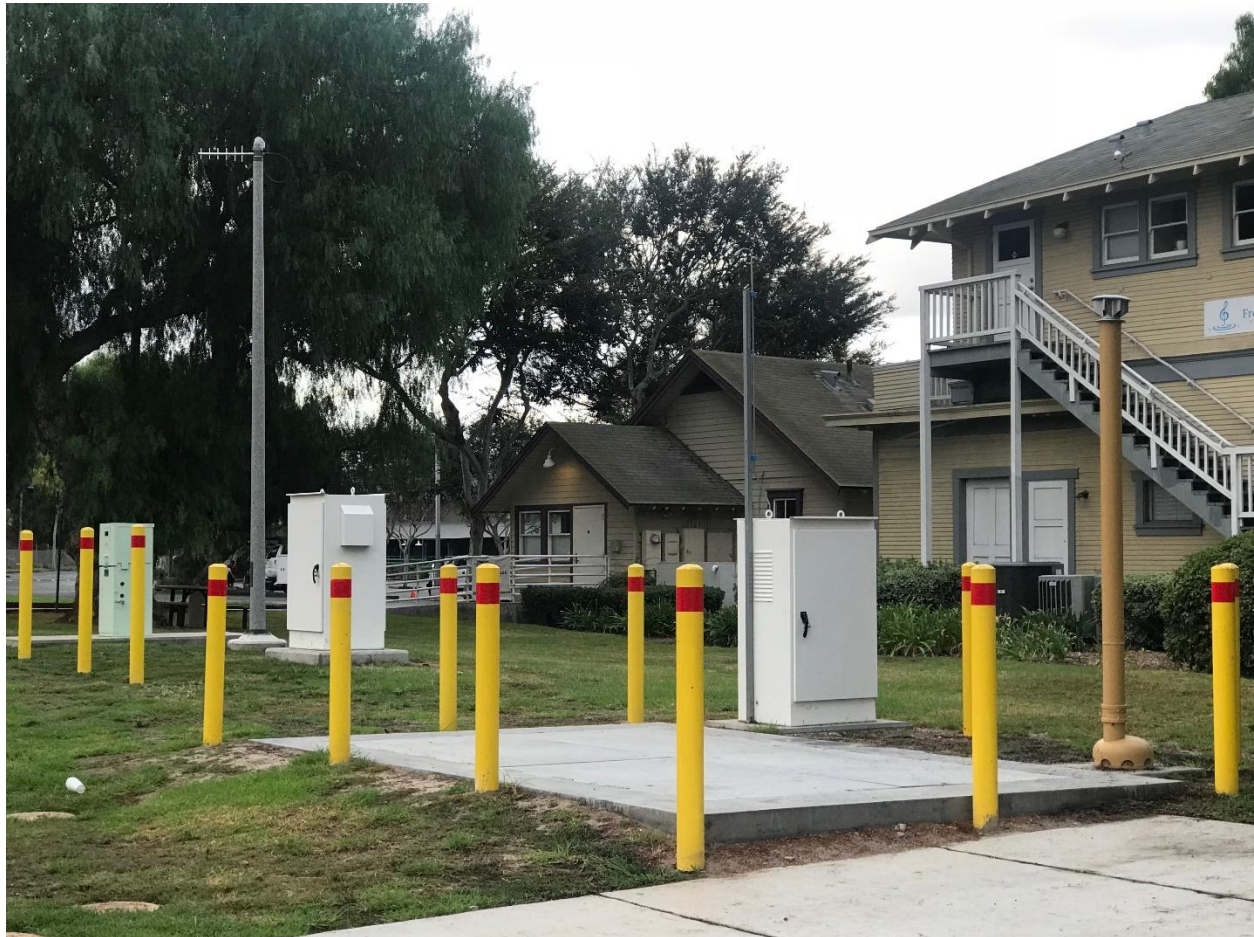
Figure 4: Project Site Post-Construction, New Vault in the Foreground, New Automation Equipment Cabinets in the Background
