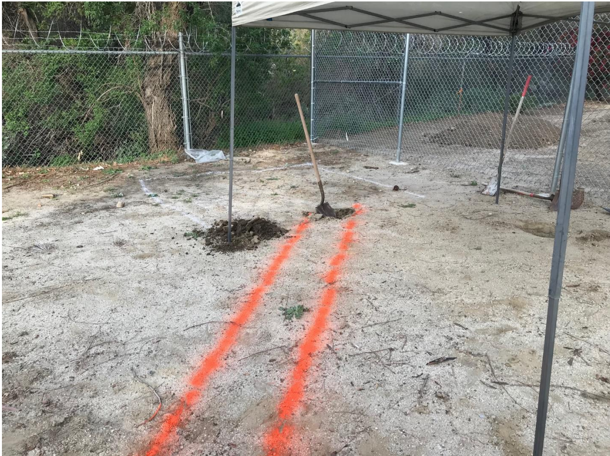
Figure 3: Marking of Trench Line for Conduit Run
