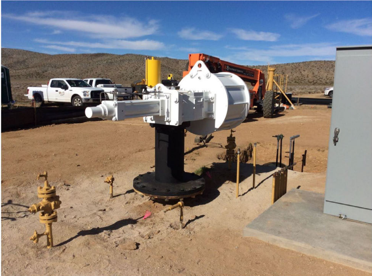
Figure 3: New Mainline Valve Actuator
