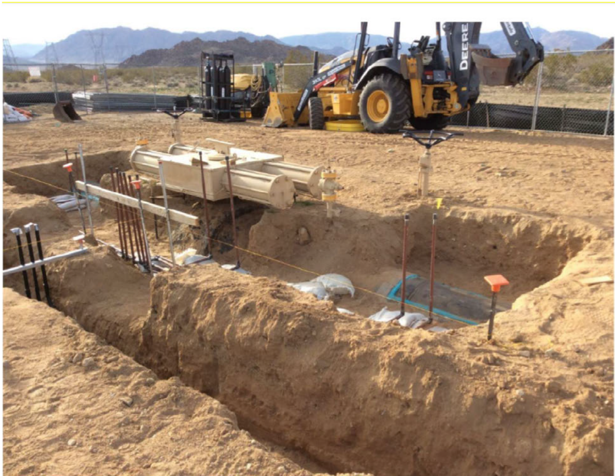
Figure 4: Excavation For New Sense Lines and Conduit
