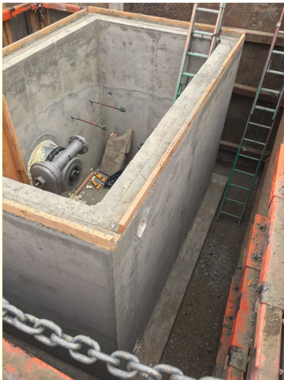
Figure 4: New Concrete Vault
