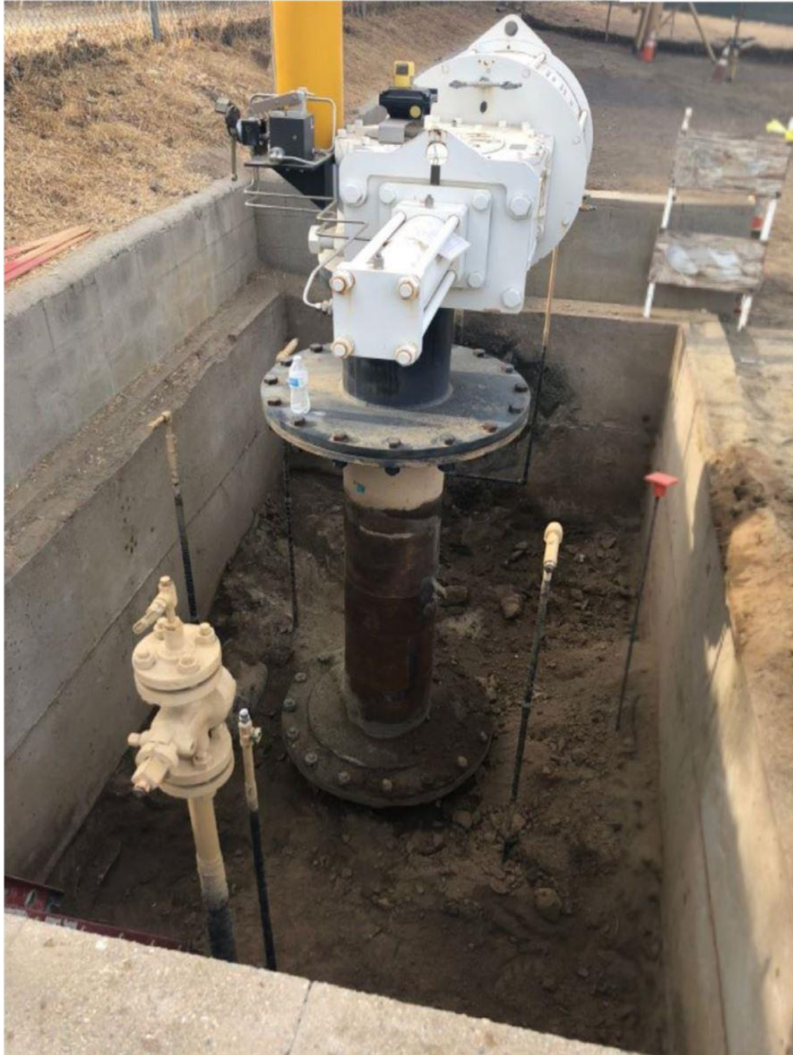
Figure 3: Existing Mainline Valve 4002-72.70-0 With Actuator
