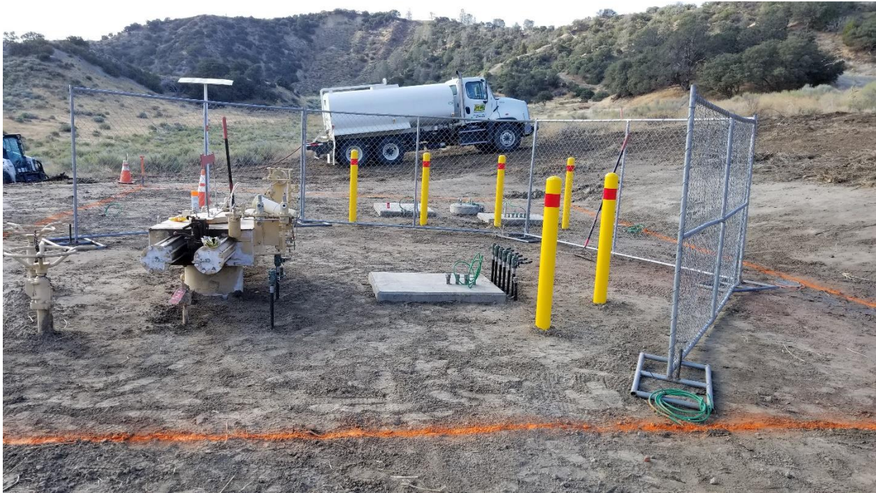
Figure 4: Project Site During Construction Foundation for the Linebreak Cabinet in the Foreground; Foundations for Solar Panel and Pole, New Battery Enclosure and New SCADA Enclosure in the Background
