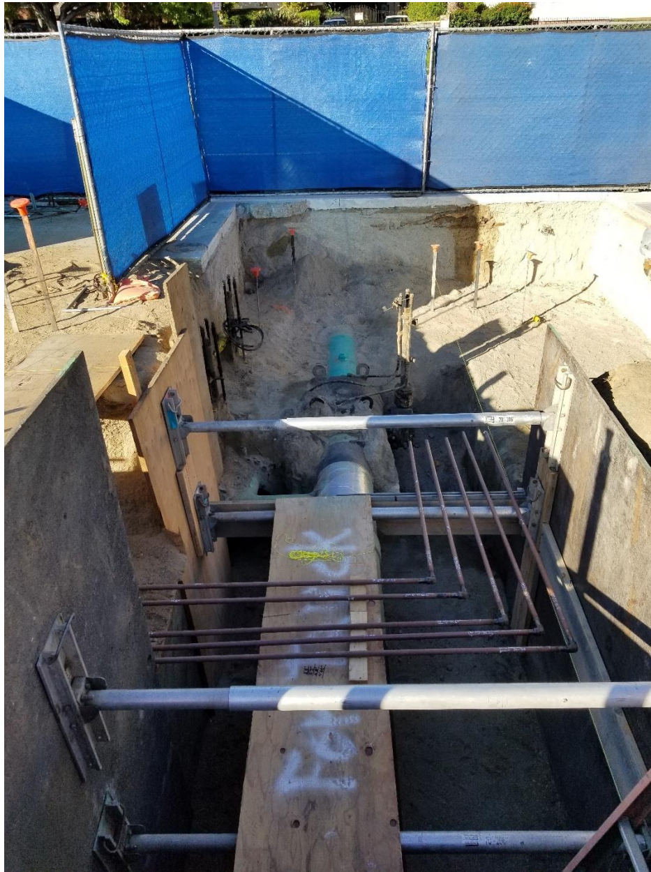
Figure 8: Mainline Valve Excavation and Instrument Piping
