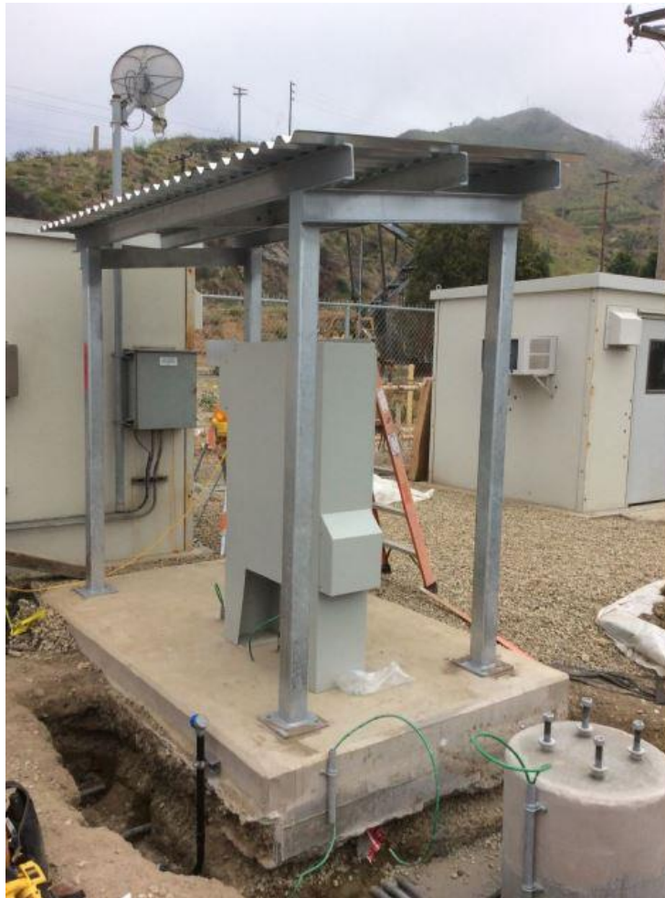
Figure 4: Linebreak Cabinet in Existing Shelter
