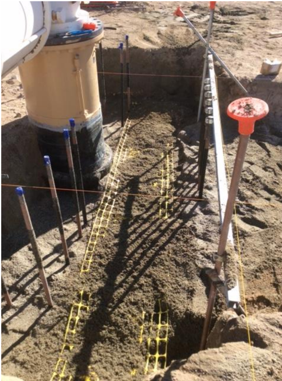
Figure 6: MLV 8B site: Sense Lines Back-Filled with Warning Mesh
