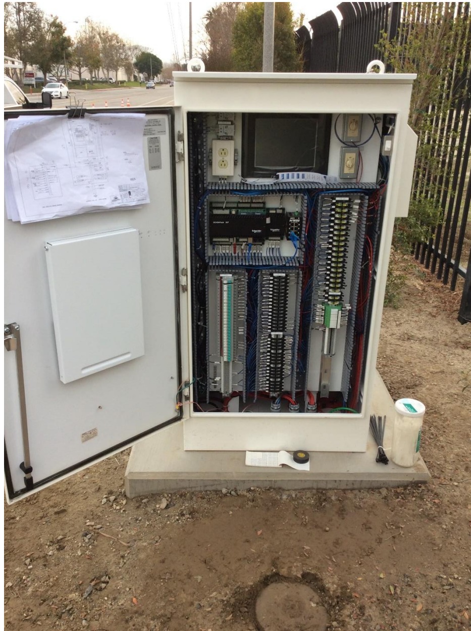
Figure 6: New SCADA Panel
