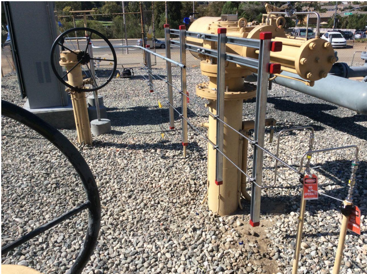
Figure 4: Existing Actuator With New Instrumentation Tubing in the Foreground, New Linebreak Cabinet in the Background
