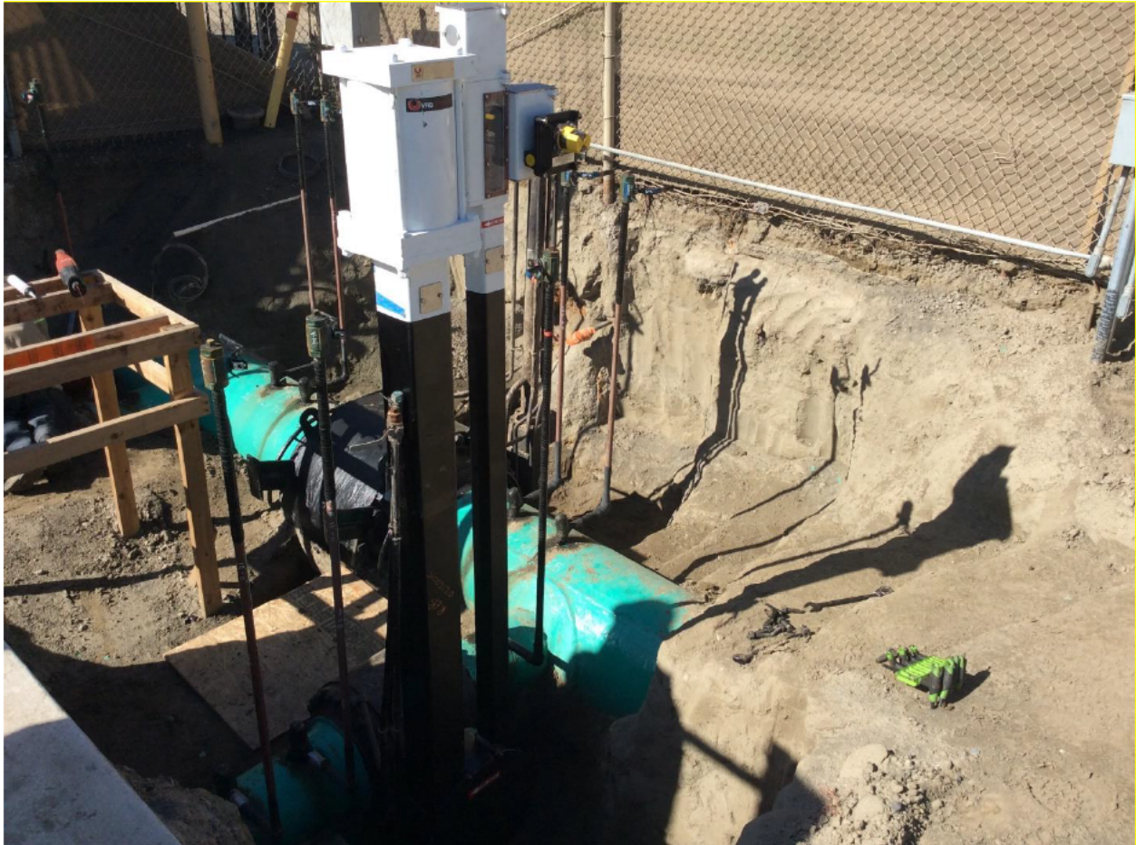
Figure 3: Excavation and New Actuator
