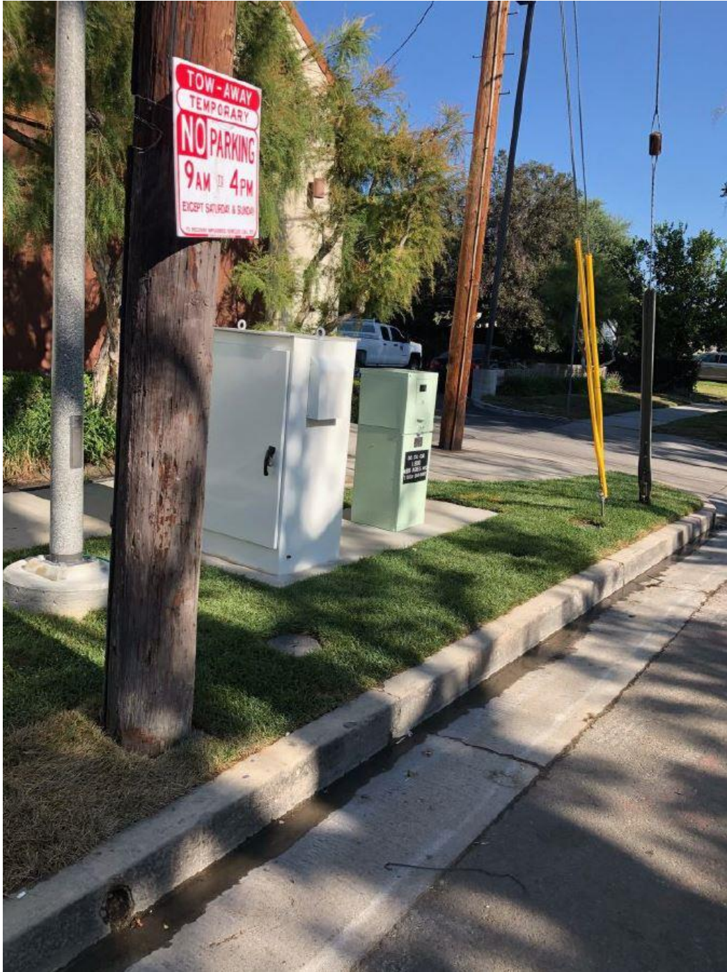
Figure 3: New Linebreak Cabinet and SCADA Cabinet
