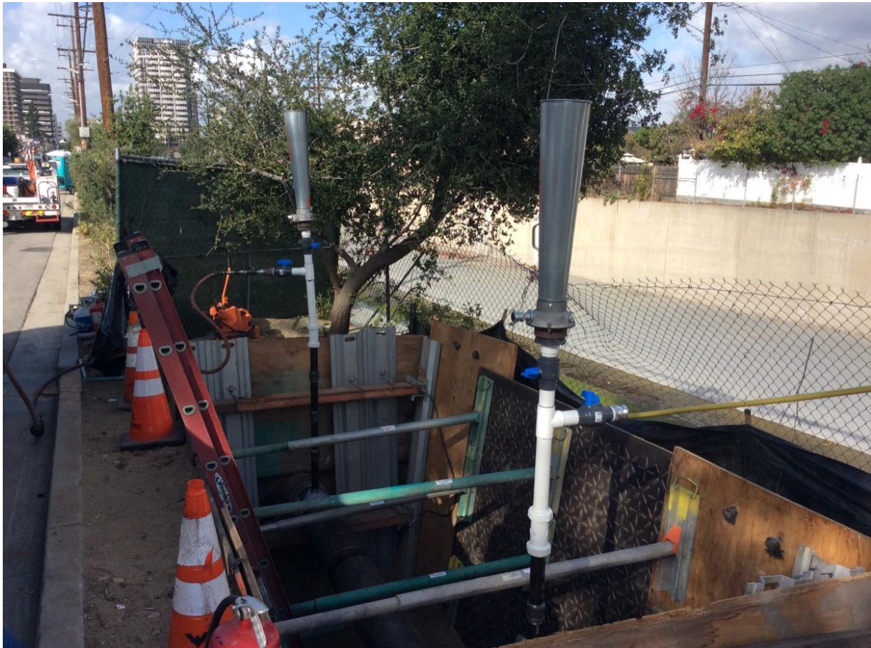
Figure 4: Excavation and Fire Control Fittings for the Tie-In
