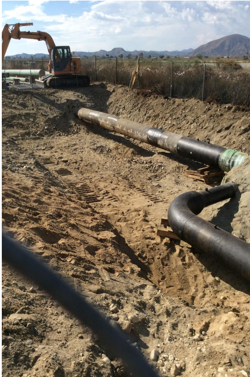
Figure 3: Excavated Line 2000 Prior to Installation of MLV 2000-138.71-0
