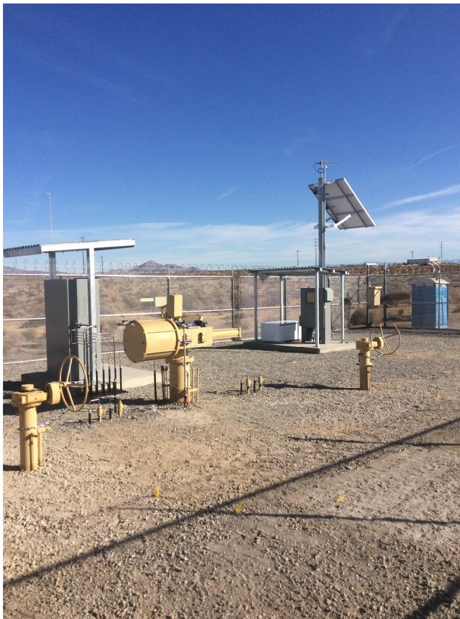
Figure 3: Project Site Post Construction, Existing Actuator and New Linebreak Cabinet in the Foreground, New Solar Array and Battery Cabinet in the Background
