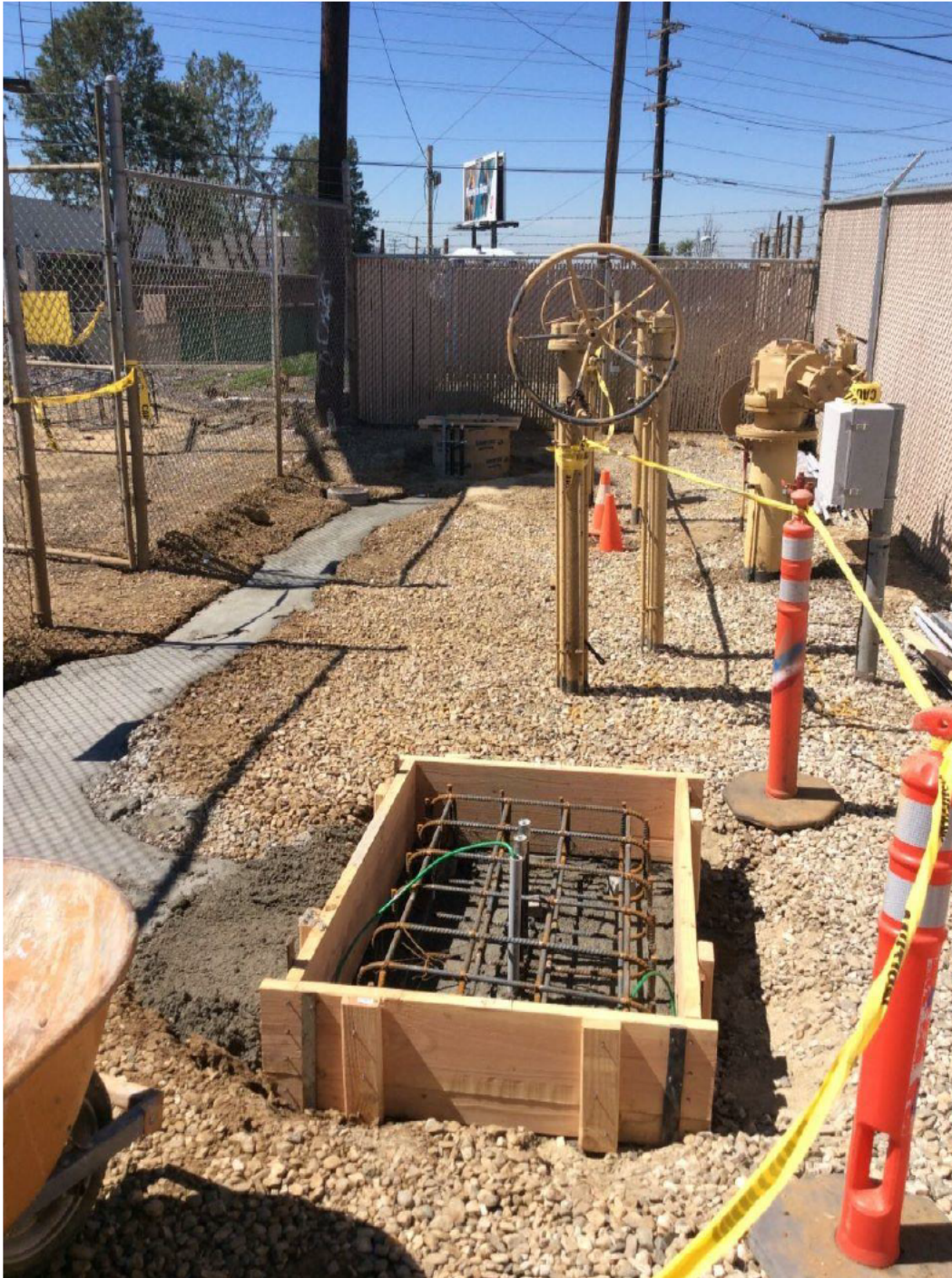
Figure 4: Linebreak Panel and Antenna Foundation Forms in Foreground, Trench for Underground in Background
