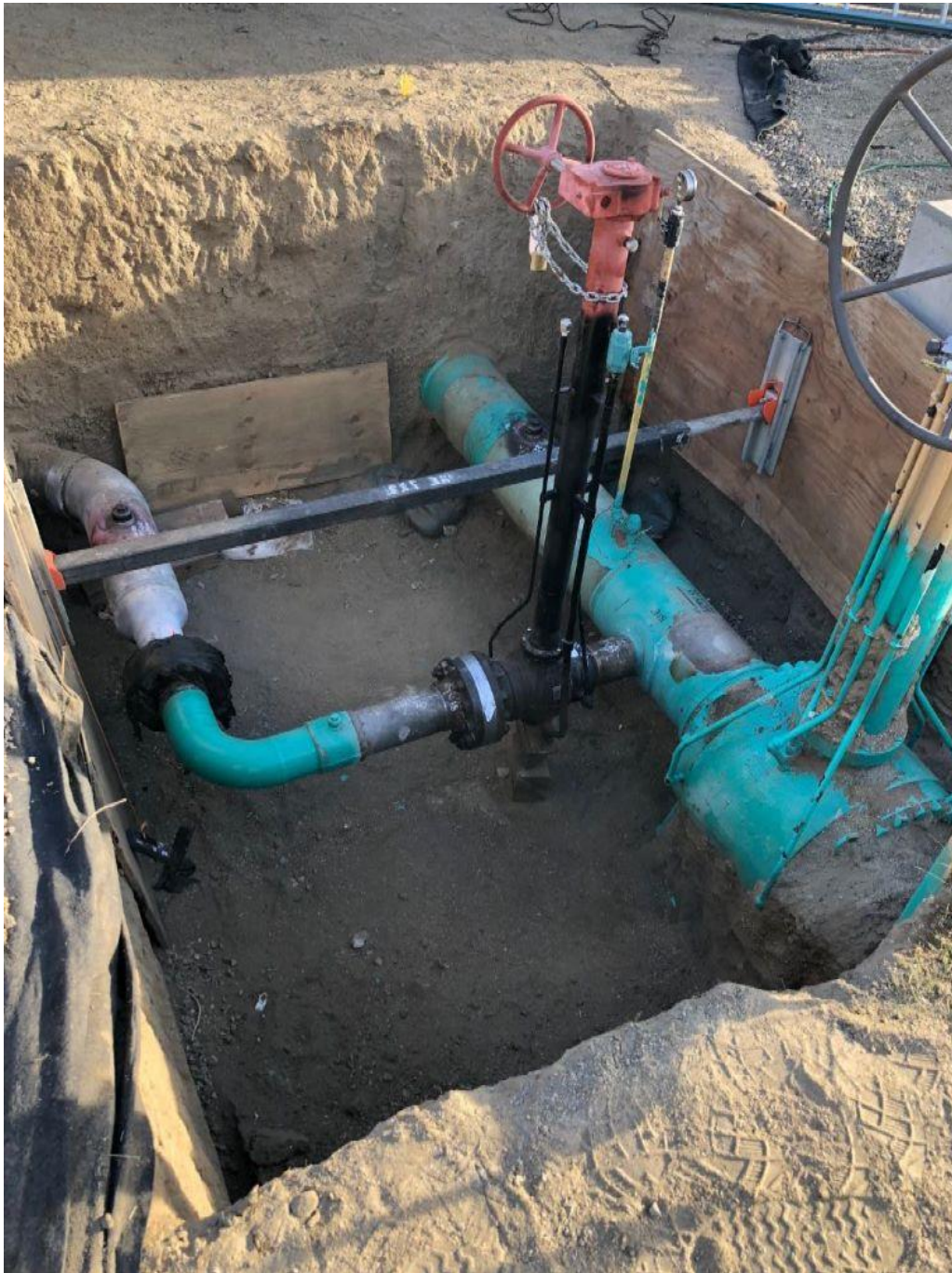
Figure 3: Mainline Valve and Bridle Excavation
