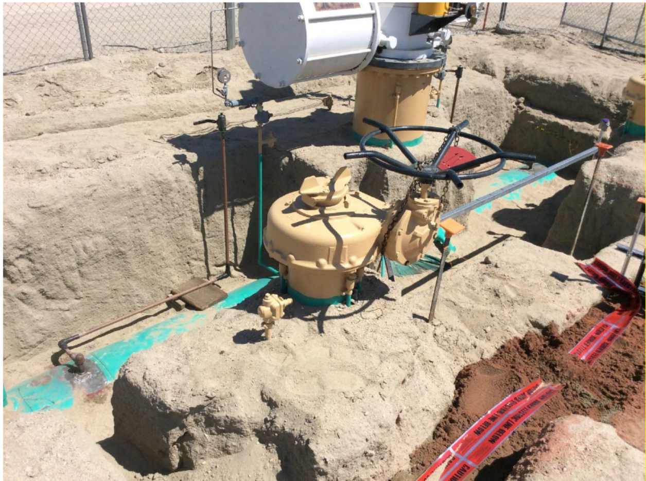
Figure 5: Pin-off Tee Installation for MLV 9B
