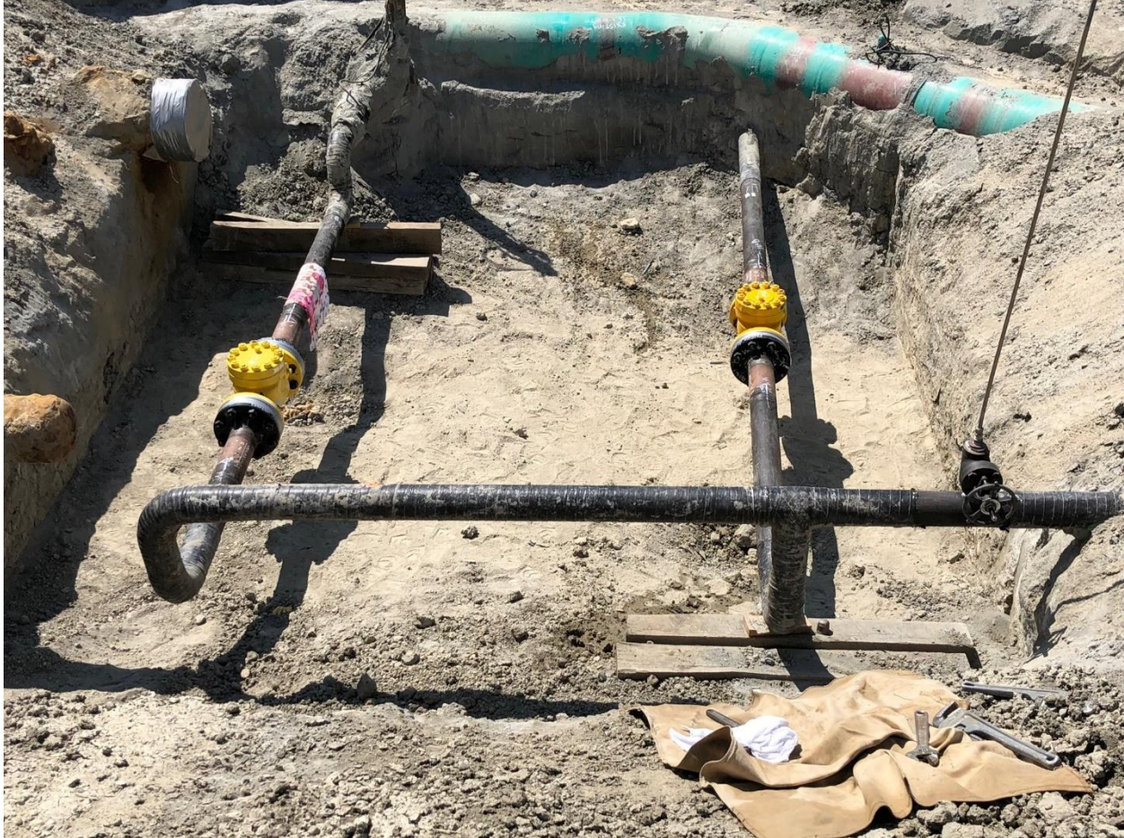
Figure 4: New Check Valve Assembly
