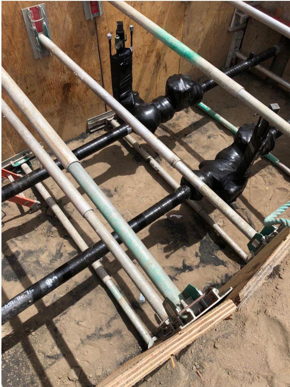
Figure 4: New Check Valve Installation
