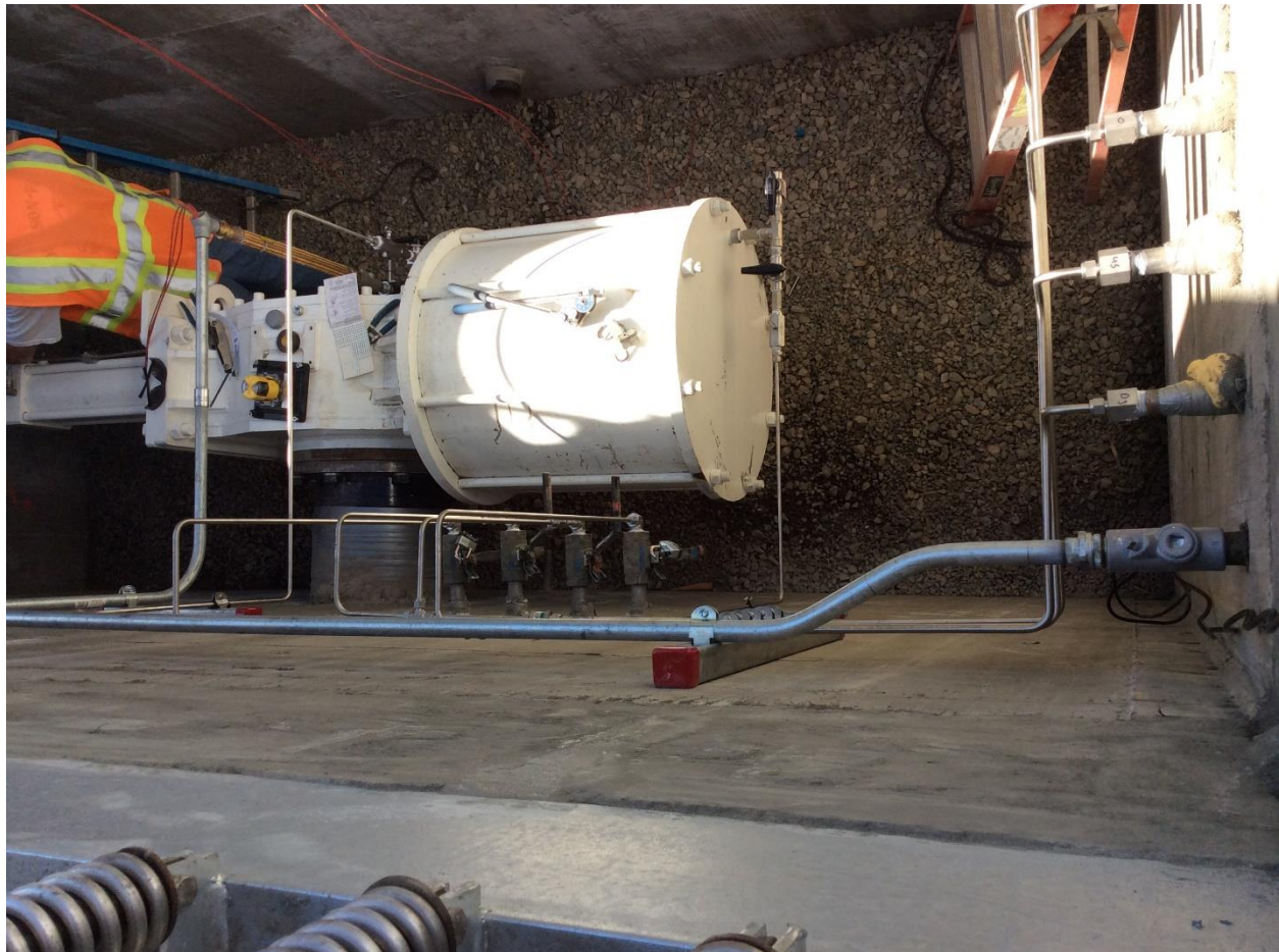
Figure 5: Overhead View of Actuator in Vault
