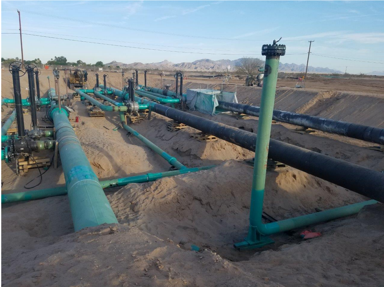
Figure 3: New Mainline Valves, Blowdowns Assembly, and Crossover Piping
