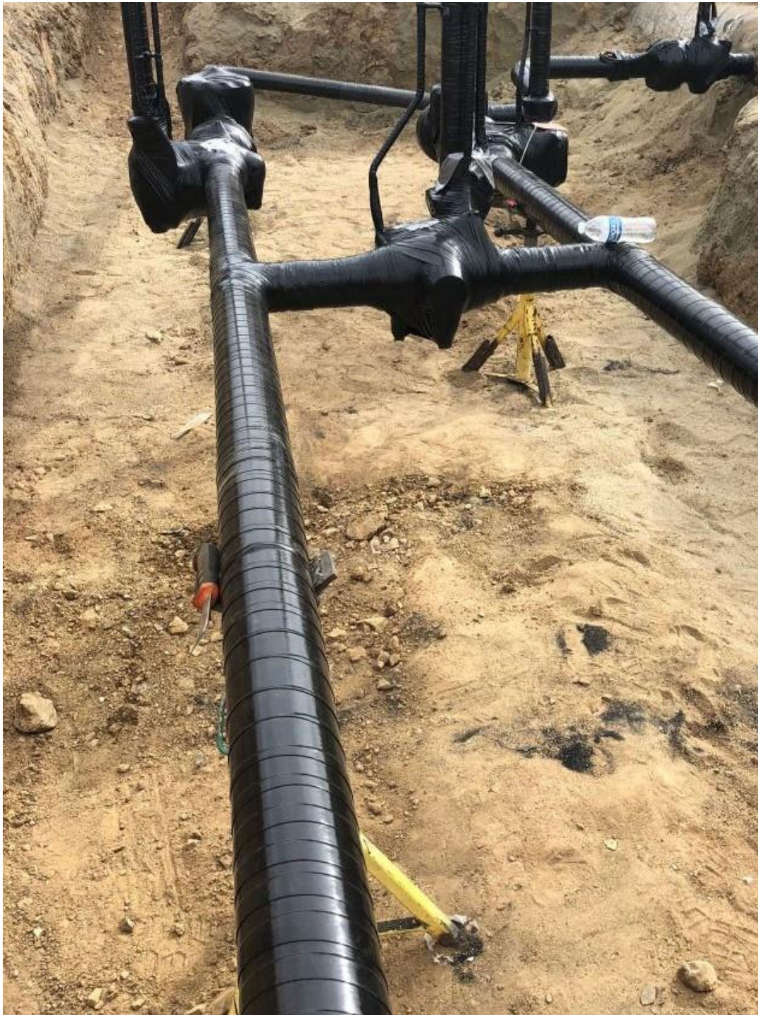
Figure 4: Installation of the Check Valves
