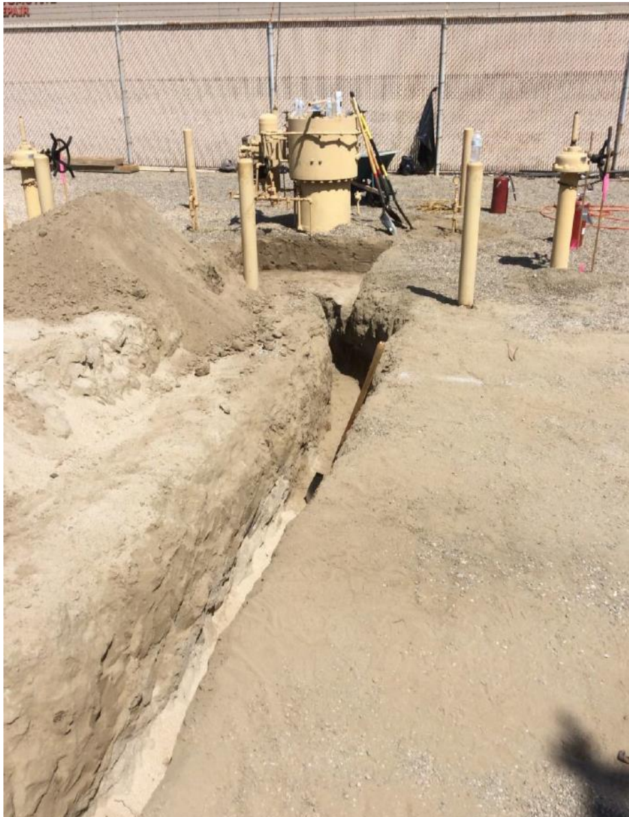
Figure 4: Preexisting Actuator Prior to Removal and the Trenching Work for Conduit to the Linebreak Panel.
