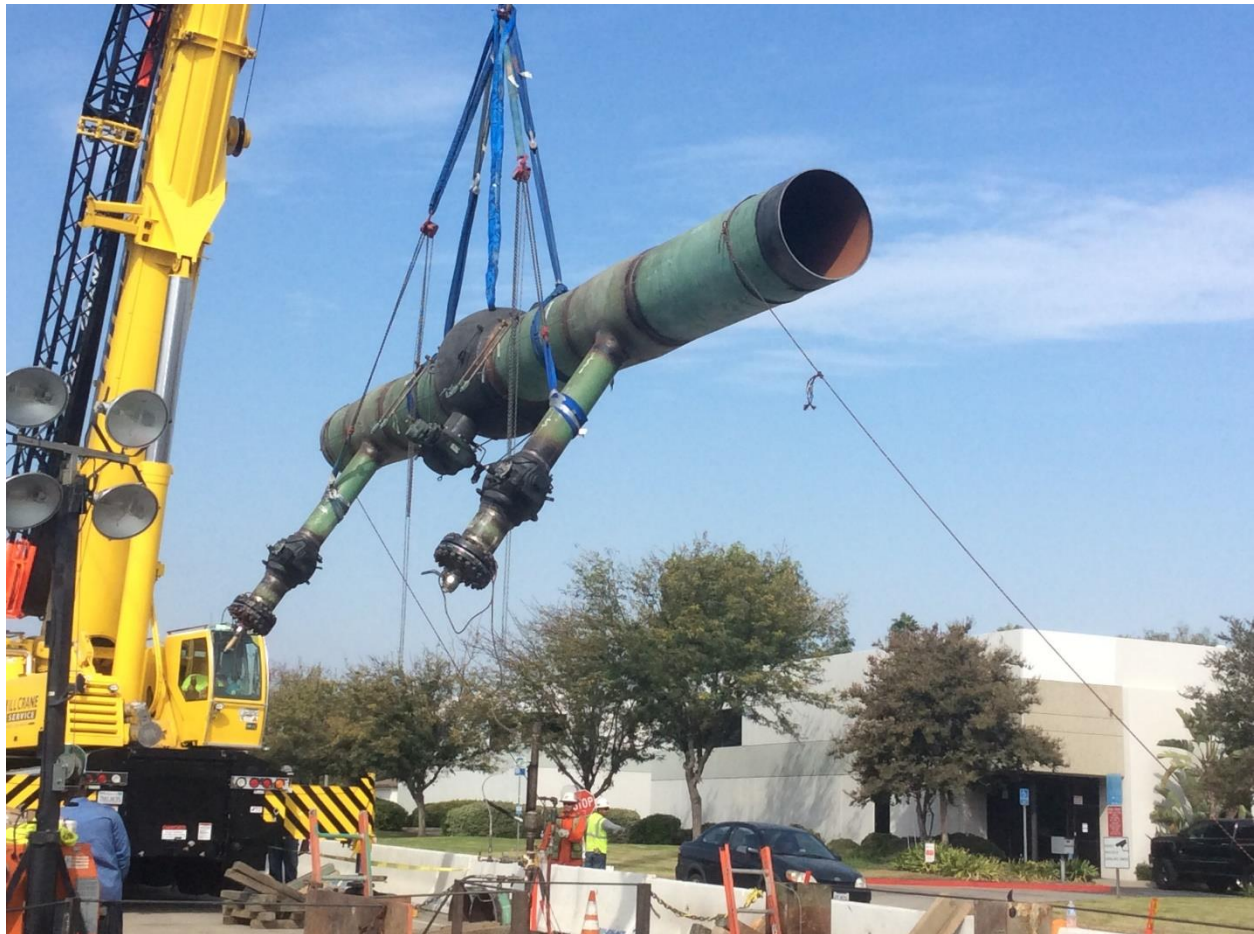
Figure 4: New Mainline Valve Installation at Benson and Chino
