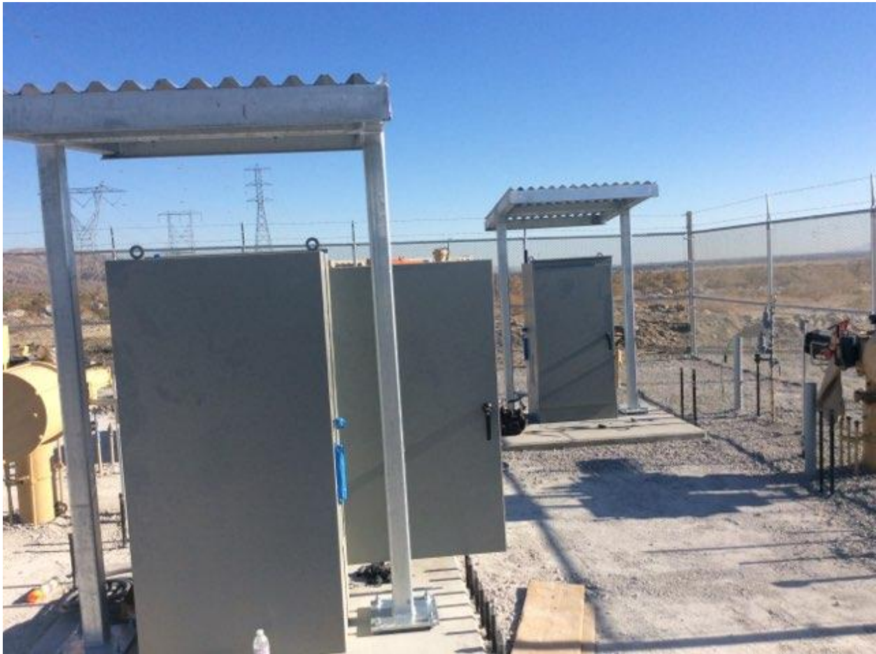
Figure 4: New Automation Equipment with Shaders
