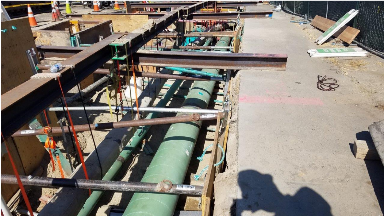
Figure 4: Excavation of Existing Pipeline
