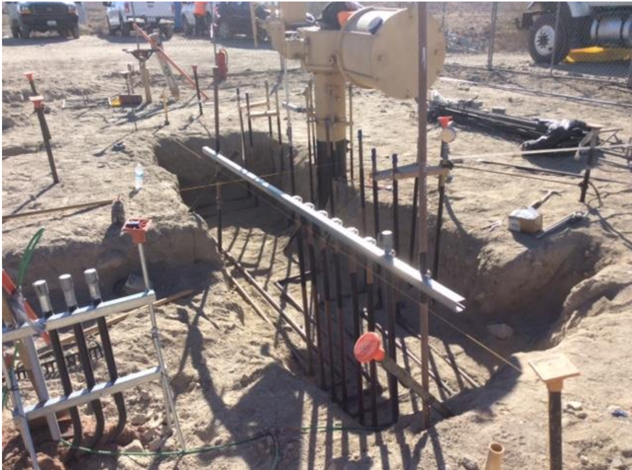
Figure 5: MLV 8 and 8A site: Sense Lines Routing to Linebreak Panel in Foreground, Actuator in Background
