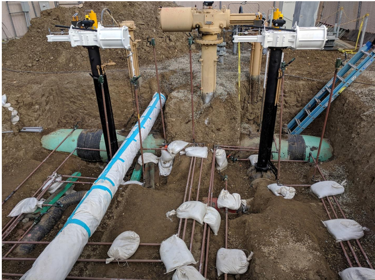
Figure 4: Excavation for the Instrumentation, New Actuators in the Foreground, Existing Actuator in the Background
