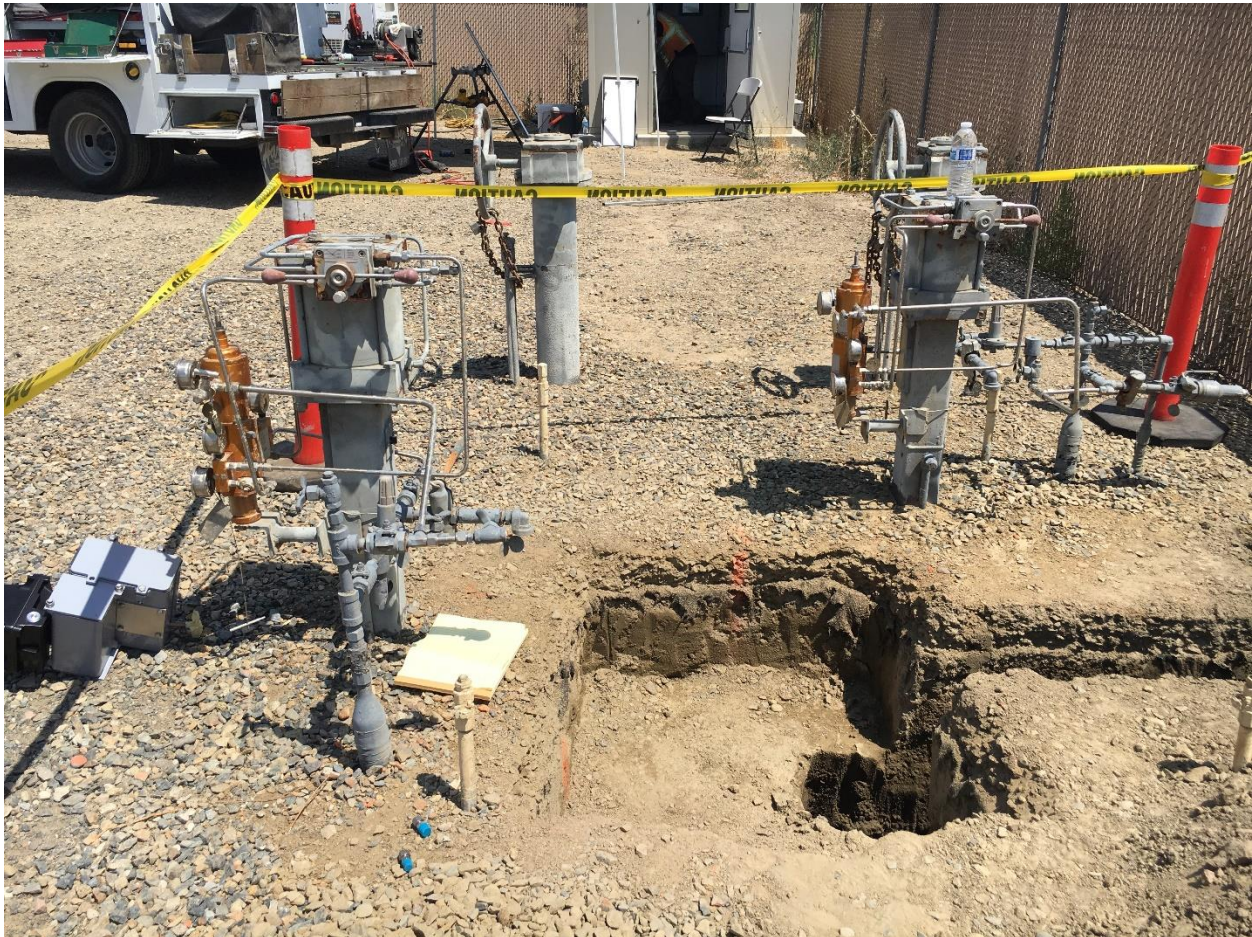
Figure 4: Existing Above Grade Actuators
