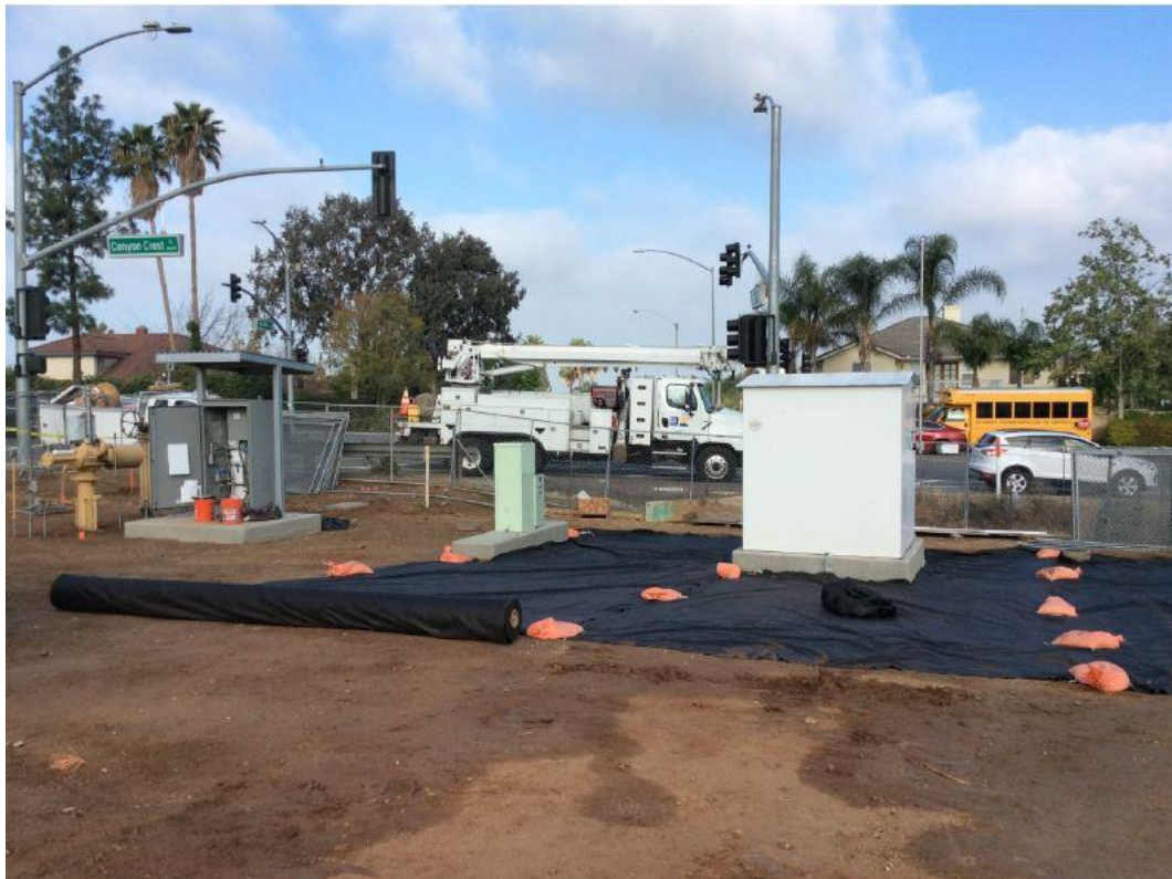
Figure 4: New Linebreak Cabinet, Power Pedestal, and Equipment Shelter
