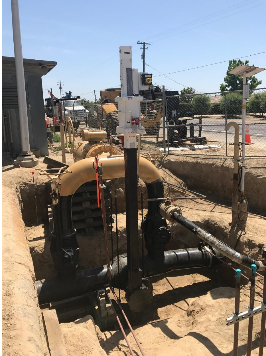
Figure 4: Excavation Around Valve Assembly and New Actuator
