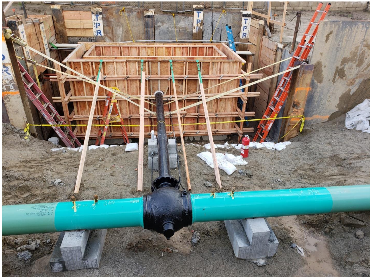
Figure 5: MLV and Framework Prior to Fabrication of the Cast-in-Place Vault
