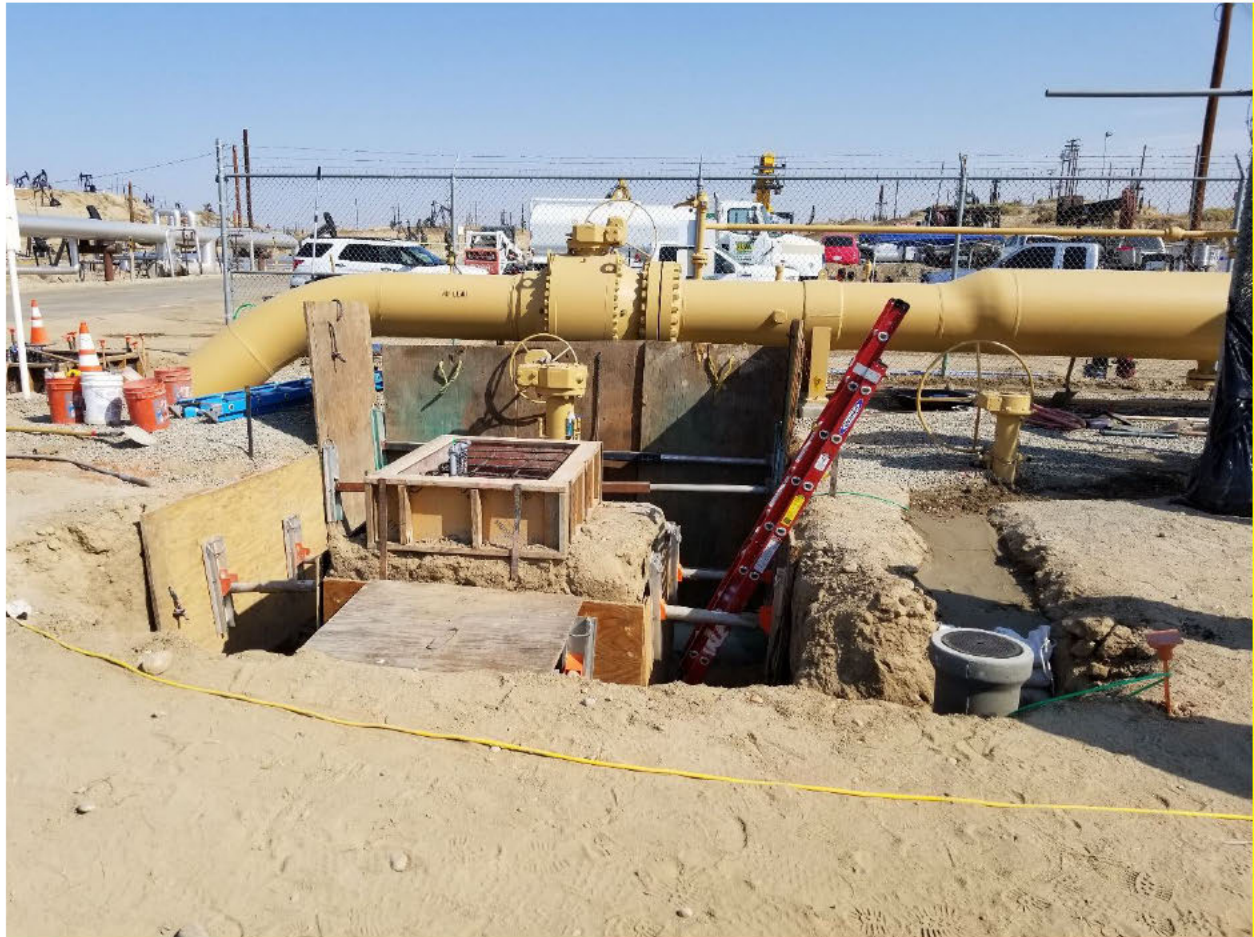
Figure 4: Excavation for new Actuator Installation in Foreground, Existing Pig Launcher in the Background
