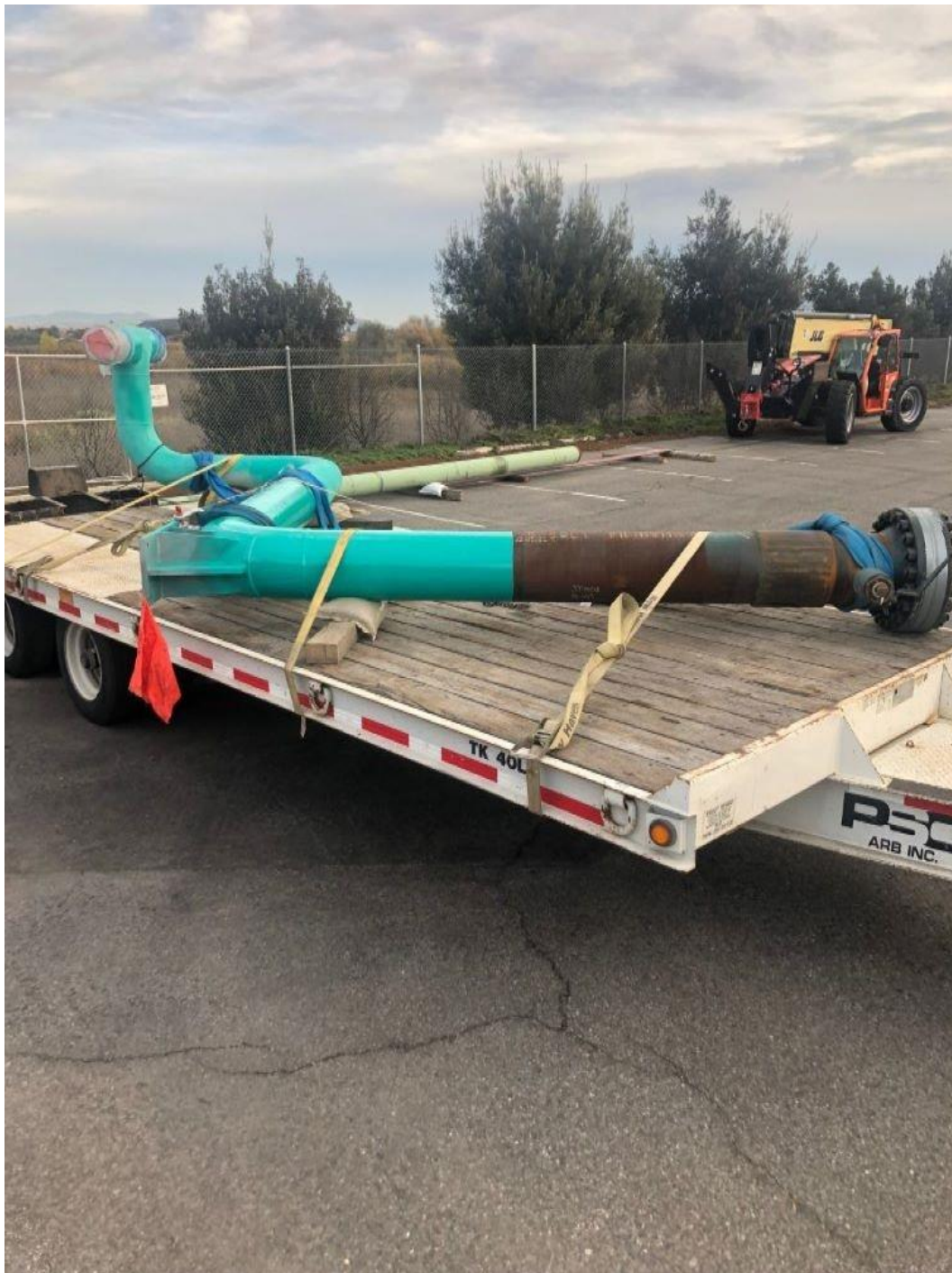
Figure 3: New Blowdown Piping Prior to Installation
