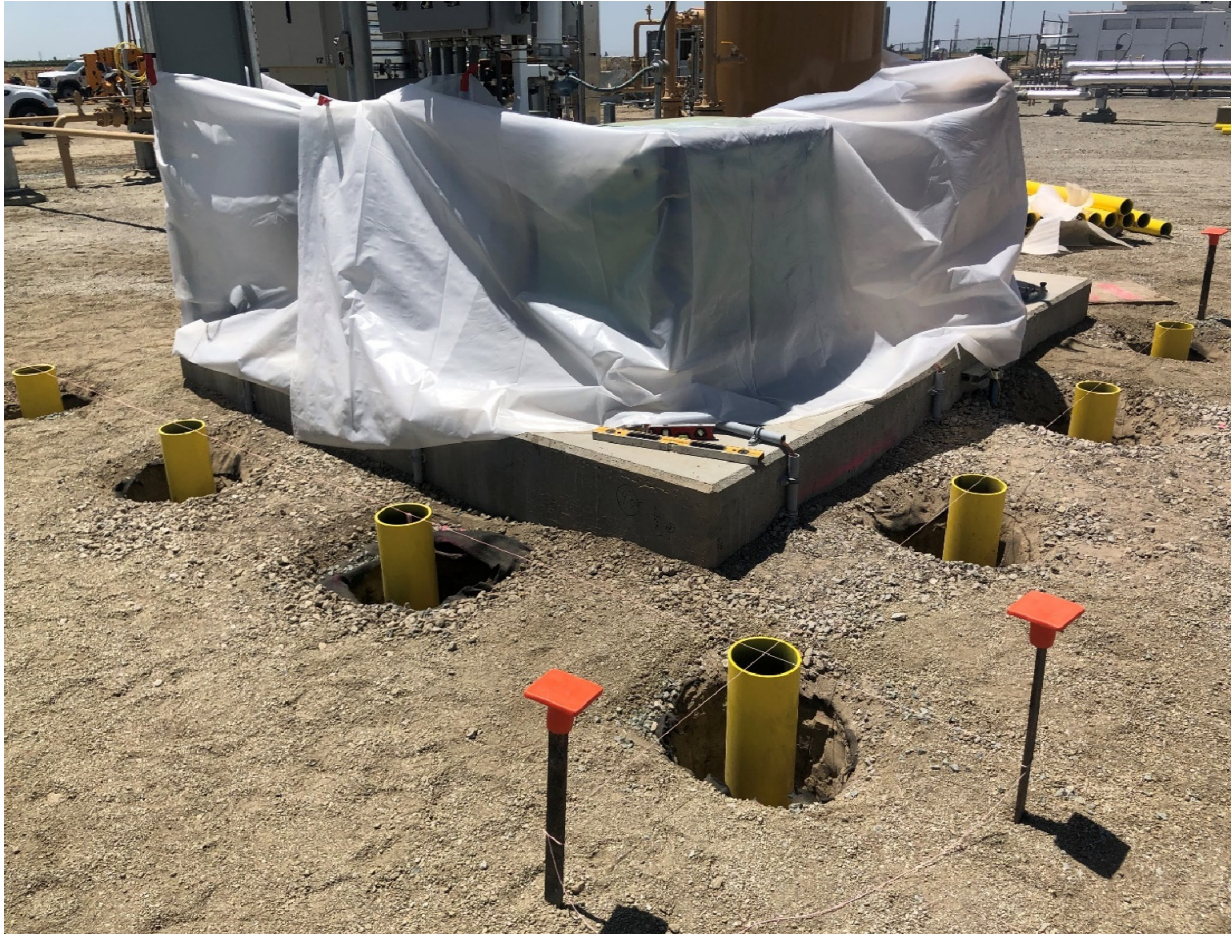
Figure 9: Installing Support Beams for Equipment
