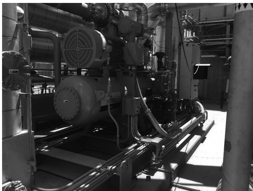
Figure 2 - Vilter Compressor Installed at Project Team's Calgren Dairy Fuels Biogas Conditioning Hub
