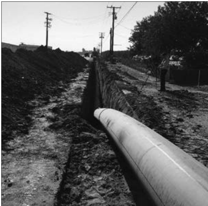
Biogas Pipeline in Tulare County
