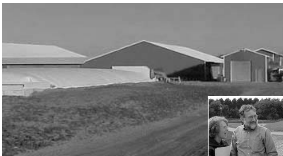
Haubenschild digester barn and electrical generation building is shown above. Dennis Haubenschild (right) visits with field day tour participants.
