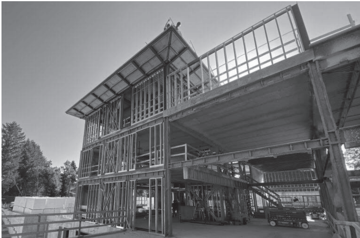
This 19,600-square-foot home near Toronto features high-performance building techniques, including steel framing.
