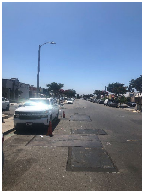
Figure 4. Recess Steel Plates over an Excavation
