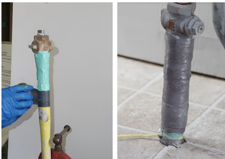
Figures 2 and 3. Anodeless Riser After Remediation
