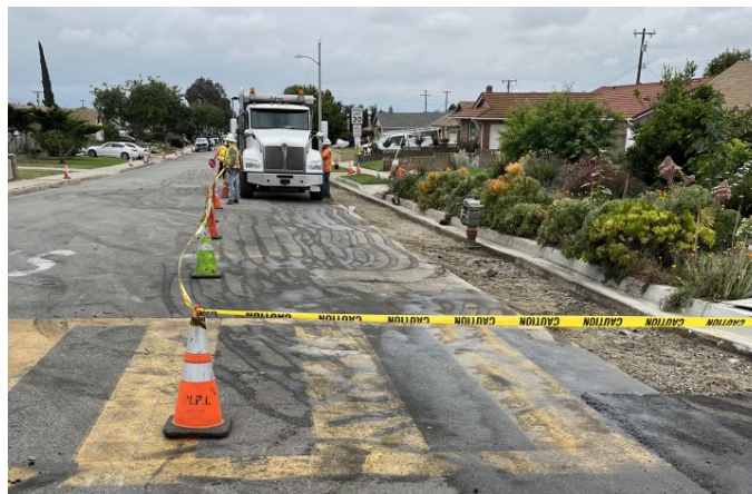
Figure 5. Removal of Asphalt During Paving
