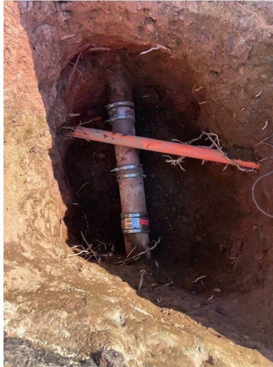
Figure 5. Repaired Cross Bore
