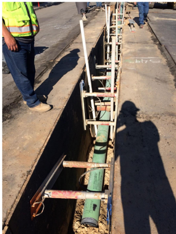
Figure 5: Pipe Being Lowered into Trench
