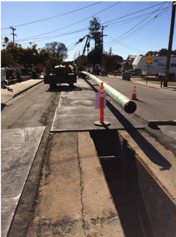
Figure 4: Pipe Strung Out Along Alpine Street
