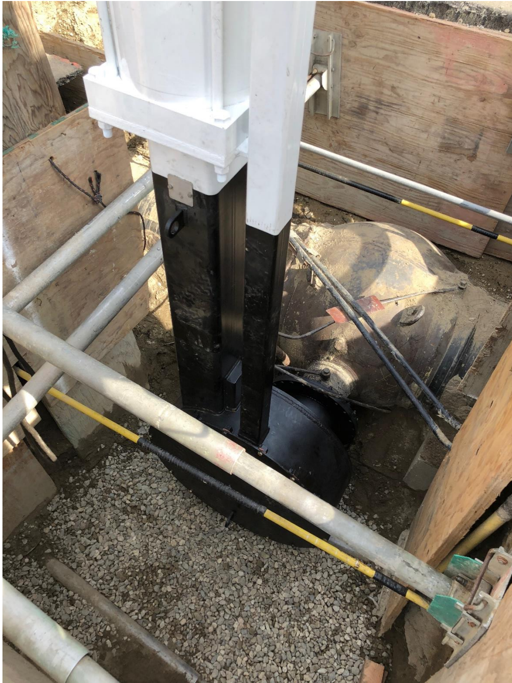
Figure 2: New Main Line Valve Actuator
