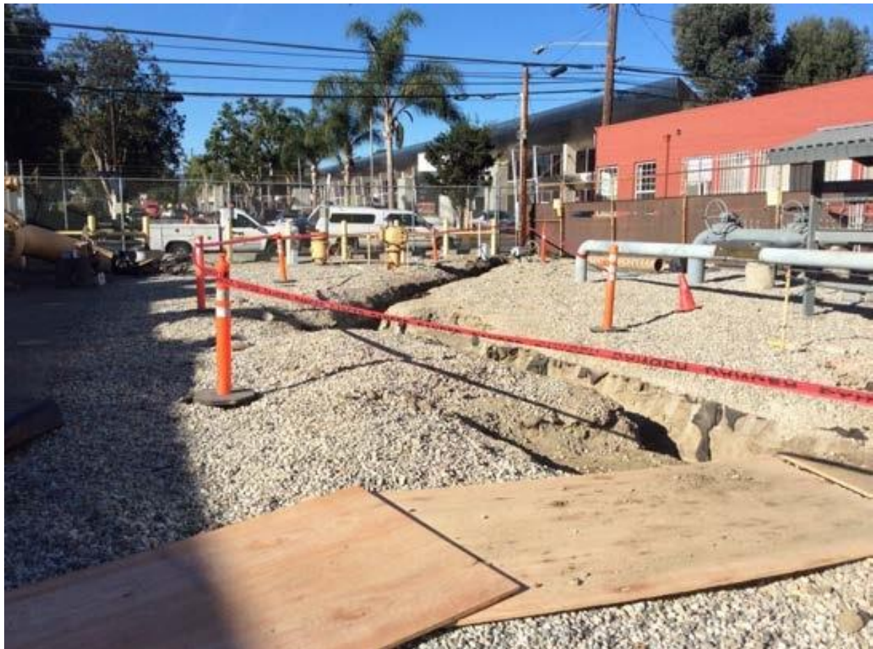
Figure 4: Trenching to Access Existing Electrical Power
