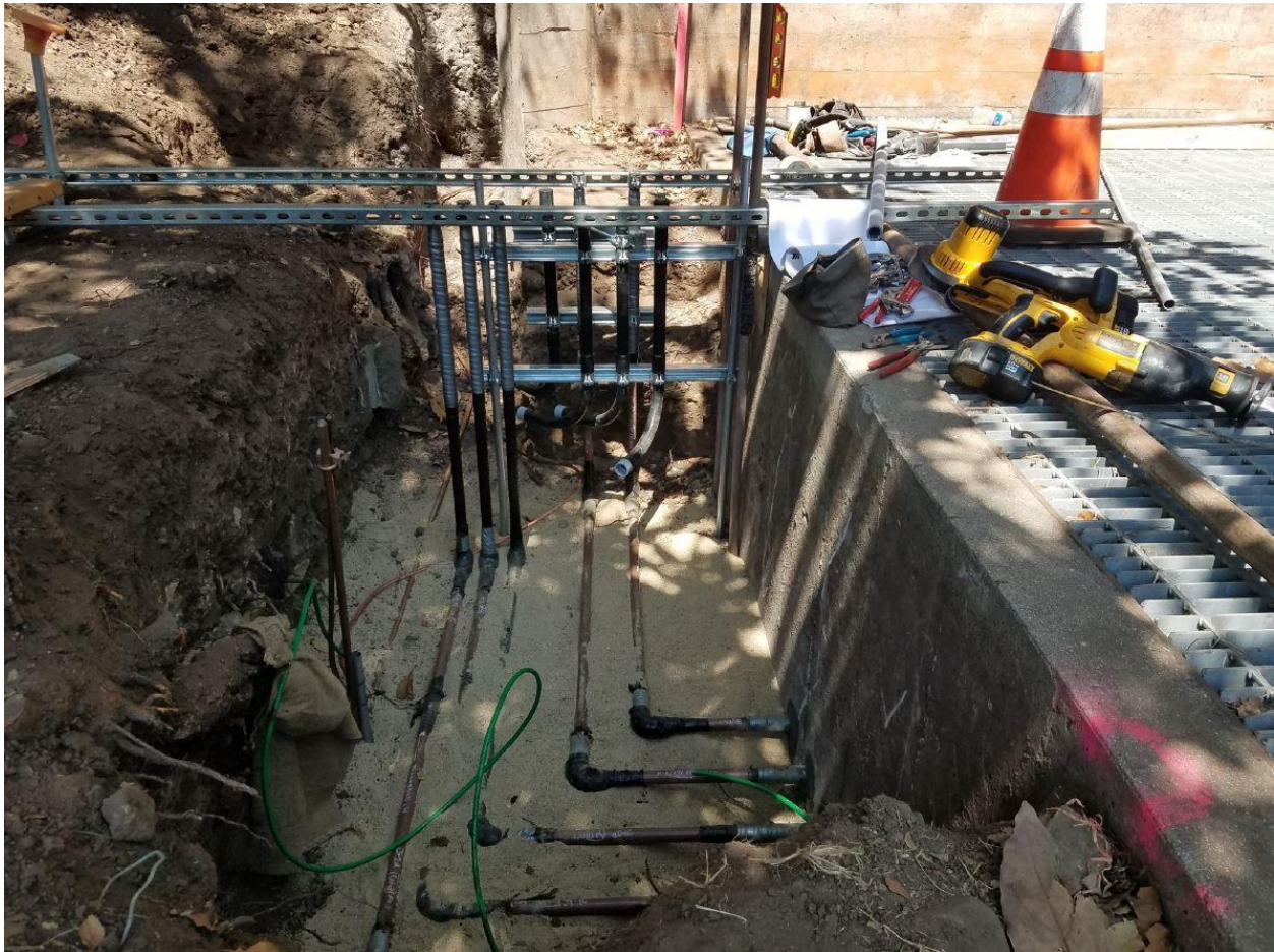
Figure 4: New Instrument Piping Exiting the Vault
