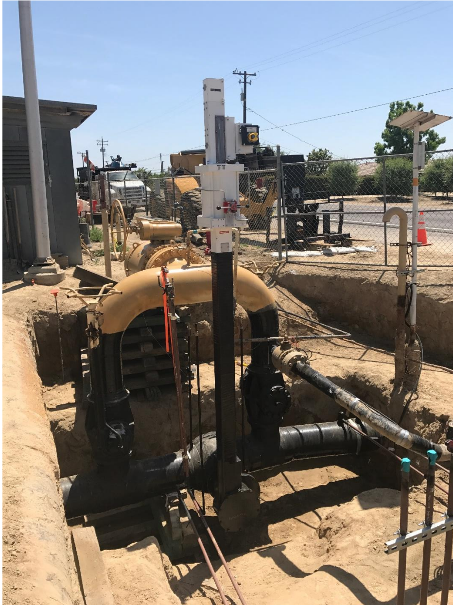
Figure 4: Excavation Around Valve Assembly and New Actuator
