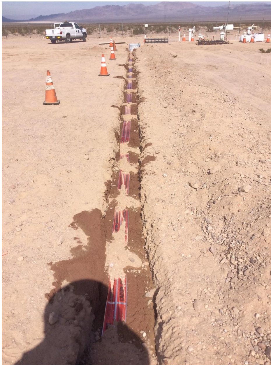
Figure 4: Partial Backfill of Conduit Trench
