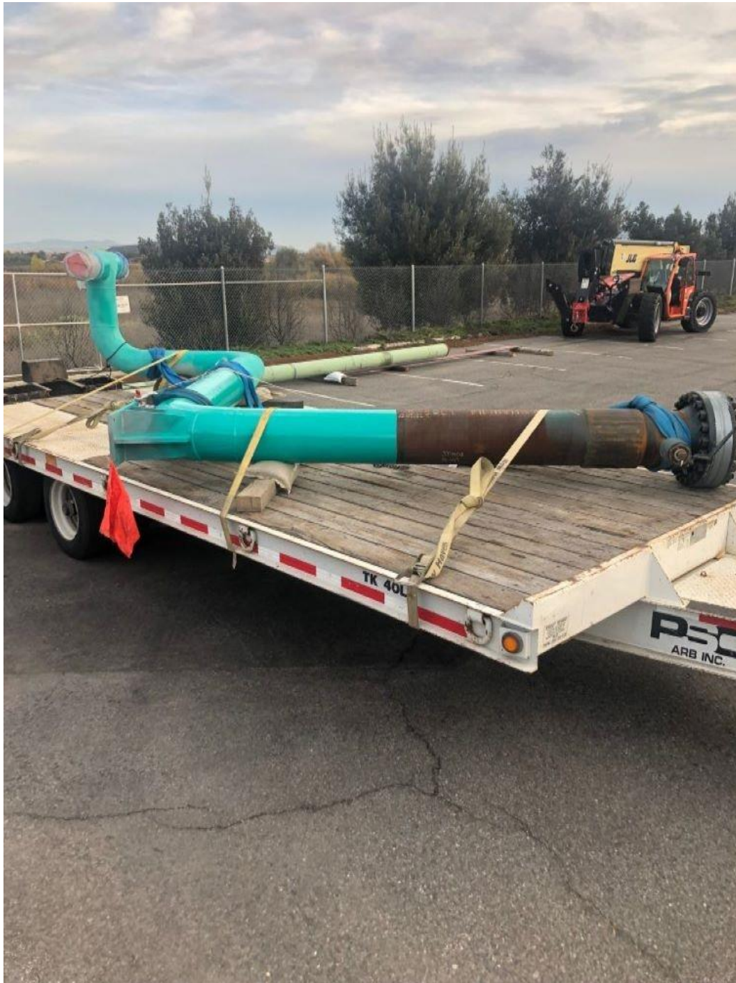
Figure 3: New Blowdown Piping Prior to Installation
