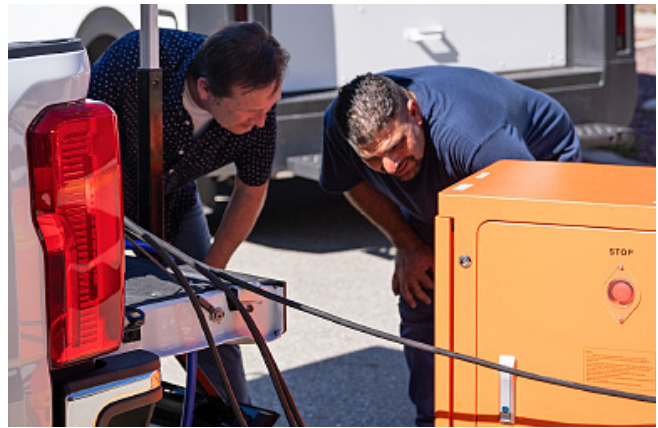
Figure 6: RockeTruck “Mini” Fuel Cell Generator Installation and Walkthrough at CSULA Demonstration
