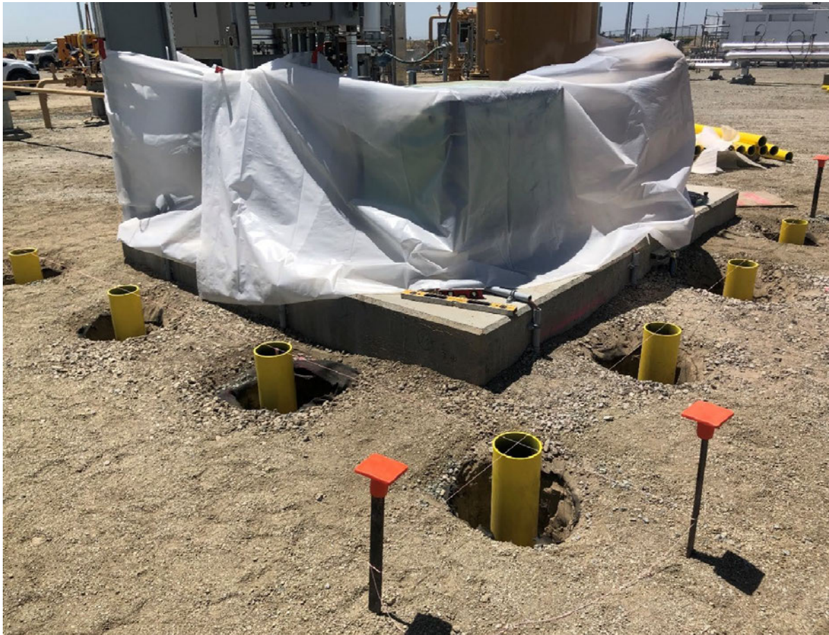
Figure 9: Installing Support Beams for Equipment
