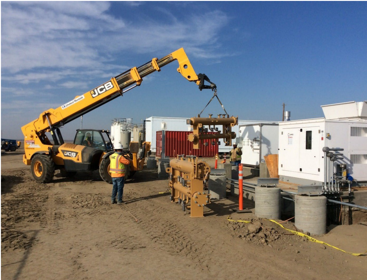
Figure 5: Placing Equipment in Lakeside Facility
