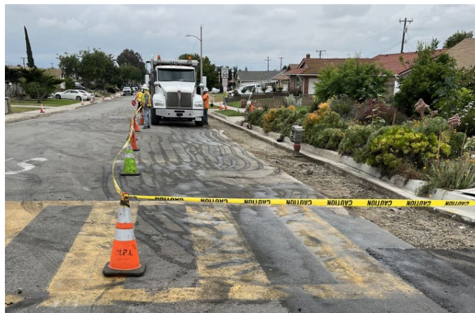
Figure 5. Removal of Asphalt During Paving
