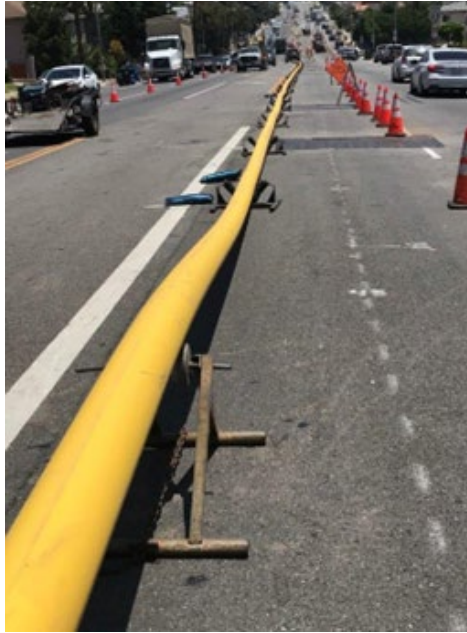
Figure 2. Trenchless Pipeline Installation Method
