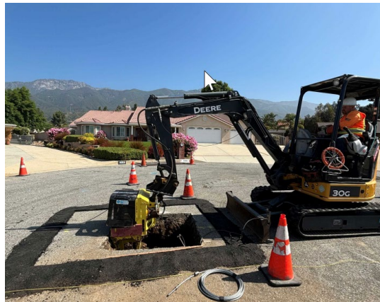
Figure 3. Pulling Installation Method
