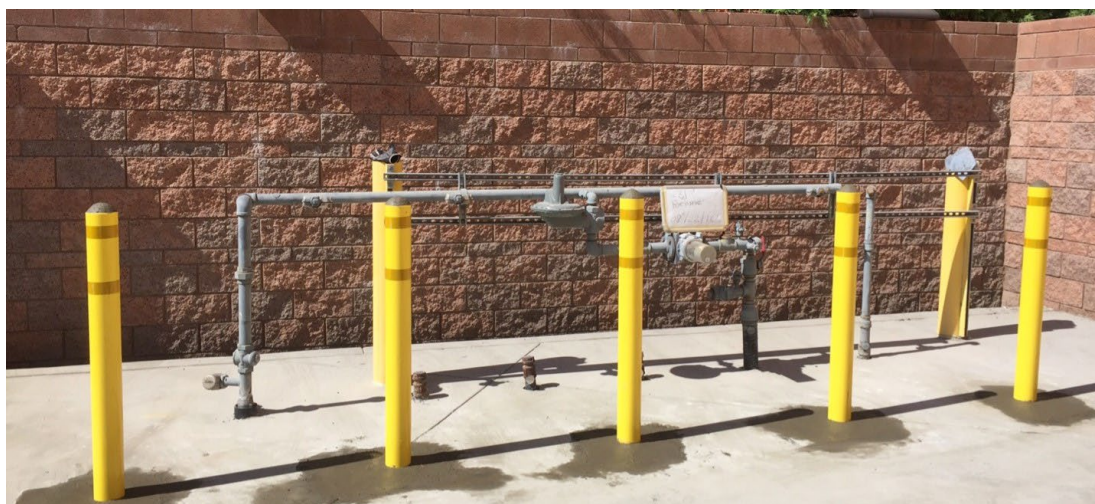
Figure 2. Bollards/ Standard Mitigation
