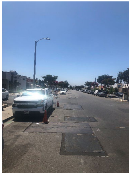
Figure 4. Recess Steel Plates over an Excavation
