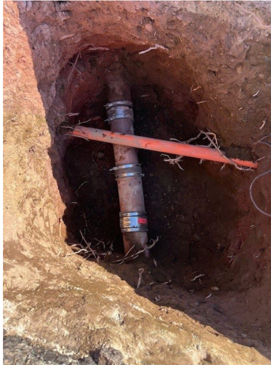
Figure 5. Repaired Cross Bore
