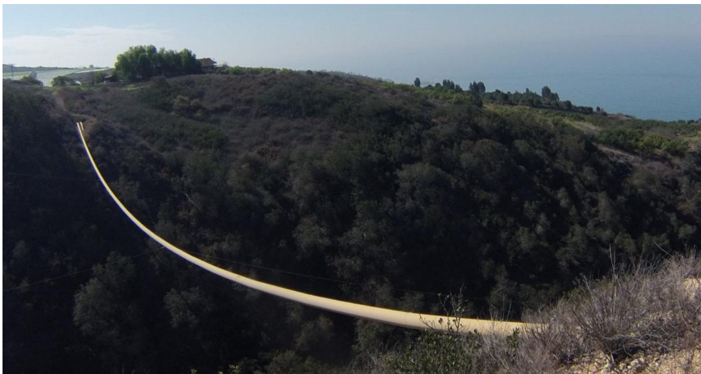
Figure 3 – Photograph of Existing Catenary Span to be Removed During the Project
