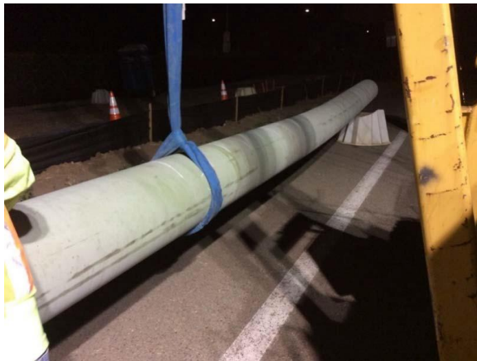
Figure 19: Pipe with Field Bend Laying on Supports
