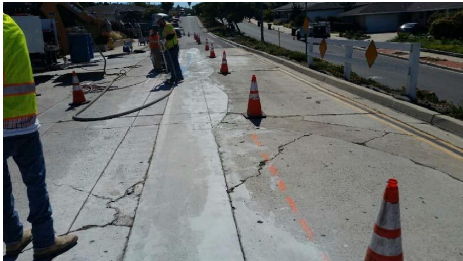
Figure 7: Saw Cutting Trench Pathway
