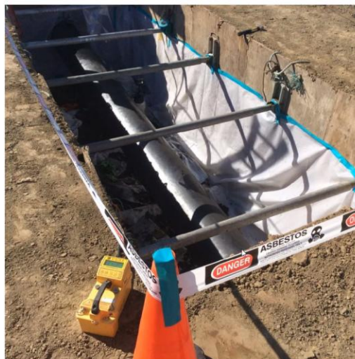
Figure 5: Typical Pipeline Abatement
