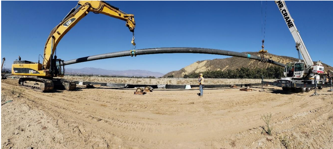
Figure 14: HDD Pullback
