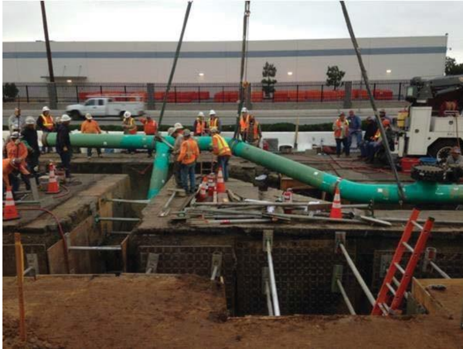
Figure 21: Lowering Section of Pipe into the Trench
