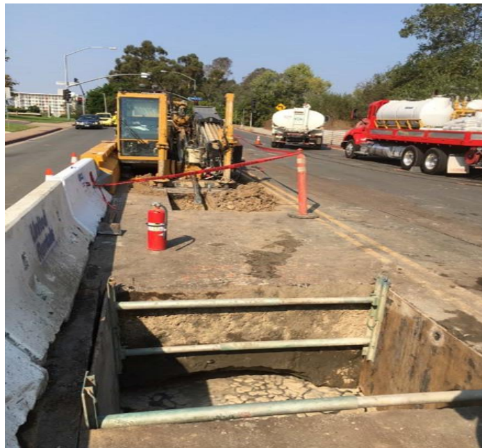
Figure 13: Horizontal Directional Drill (HDD) Equipment
