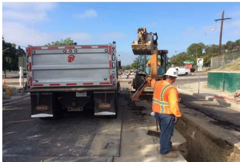
Figure 8: Trench Excavation with Backhoe
