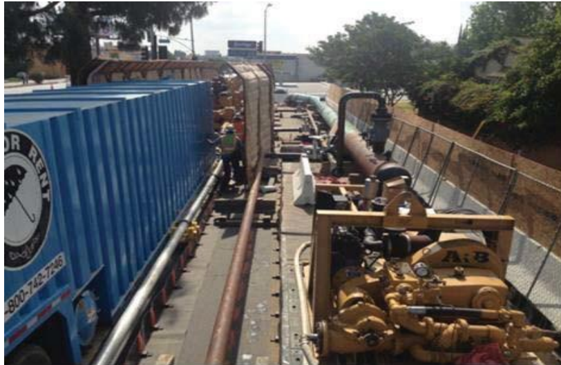
Figure 25: Hydrotest Equipment Set-up with Sound Proofing to Minimize Noise
