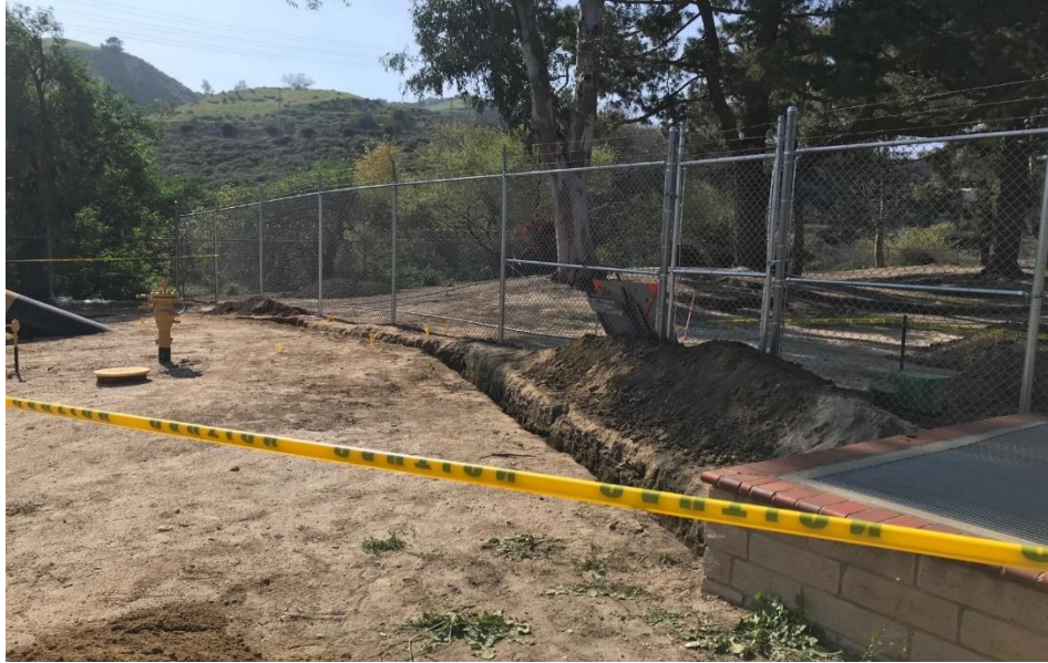
Figure 10: Hand Dug Trench
