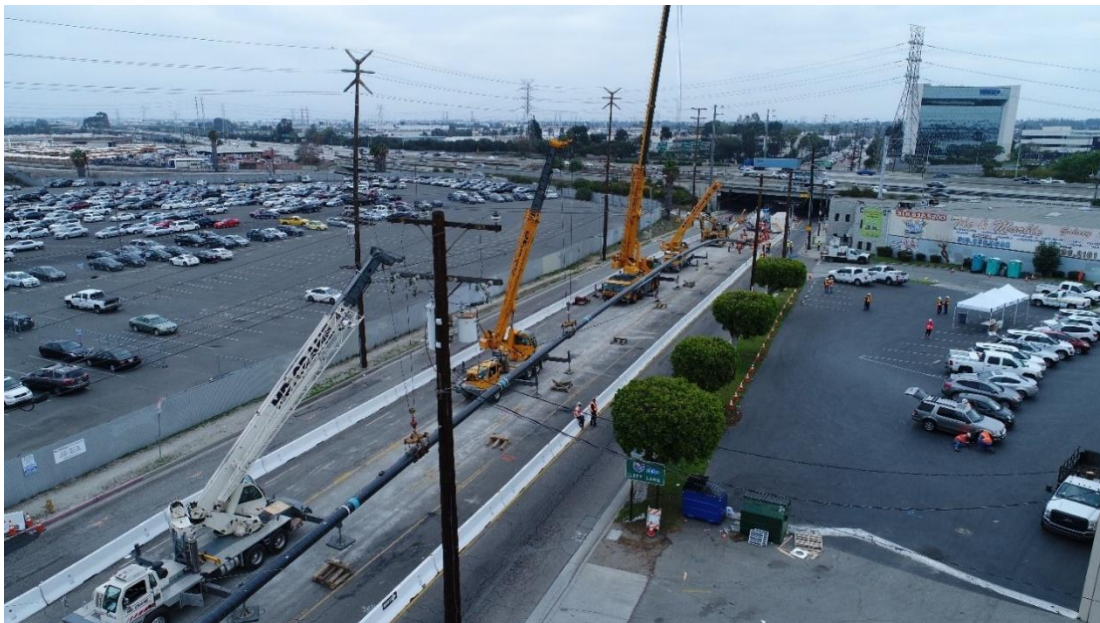
Figure 15: HDD Pullback
