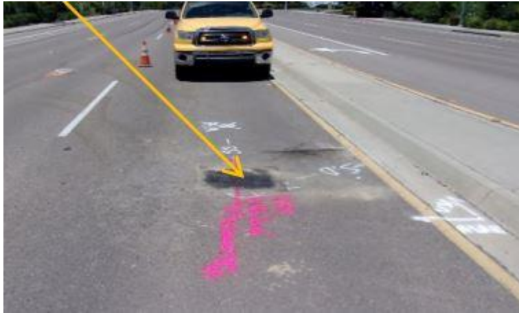
Figure 4: Potholing Location After Restoration
