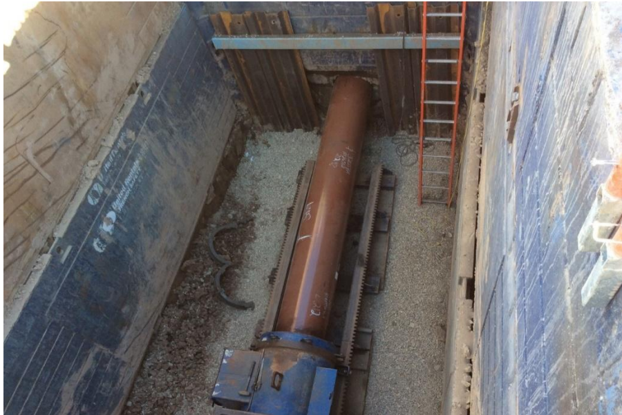
Figure 17: Boring Machine Pushing Casing Pipe
