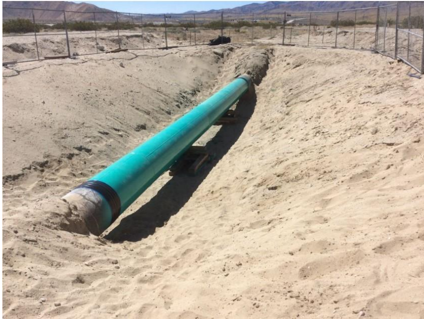
Figure 11: Pipeline Excavation and Repair Site
