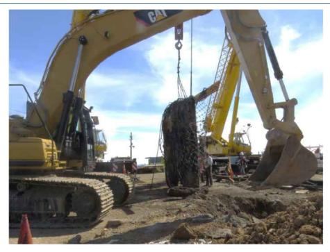
Figure 13: Concrete Slab Removed from Crater by Crane
