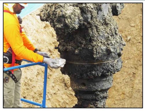
Figure 39: Cleaning the Top Bevel of Bradenhead for Surveyor Sighting Surface
