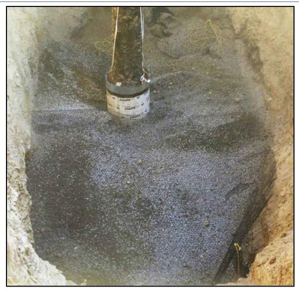
Figure 47: Top of Gravel & Geogrid Layers for Crater Bottom Stabilization
