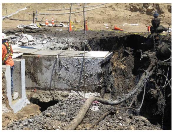
Figure 26: SS-25 Pipe Trench Segment Affixed to Crane
