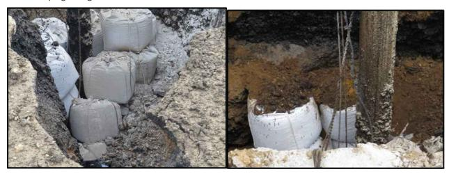
Figure 33: Conductor Appearance Before (Left) and After (Right) Excavation
