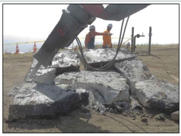
Figure 15: Concrete Slab Jackhammered into Pieces
