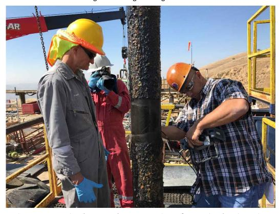
Figure 22: Inspecting the Area Below a Connection Before Cutting the 7 in. Casing
