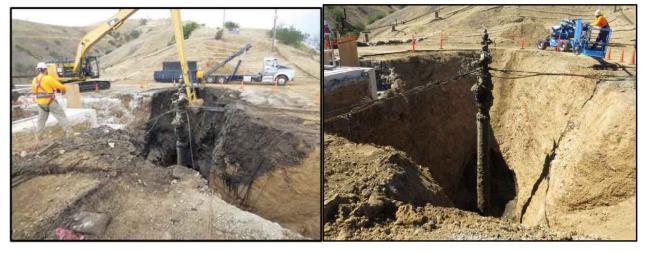
Figure 35: Crater Appearance Looking North Before (Left) and After (Right) Excavation
