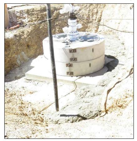
Figure 60: Backfilling Crater with CLSM Slurry Resumes
