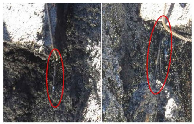
Figure 3: Visual Indications of Rebar
