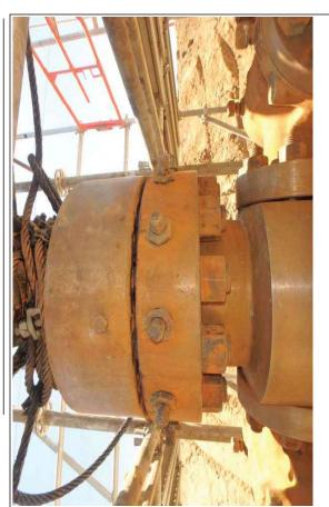
Description: Surface preparation of wellhead tree prior to MPI contrast paint
