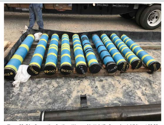
Figure 33: 7 in. Connection Sections Wrapped in Volatile Corrosion Inhibitor at PS-20
