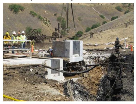
Figure 28: Another SS-25 Pipe Trench Segment Removed with Crane
