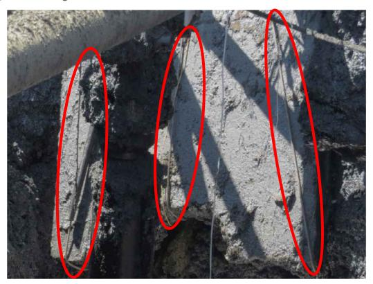
Figure 8: Three Safety Straps Were Tightened around Slab
