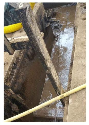
Figure 25: Cleaned Condition of Pipe Trenches and SS-25A and SS-25B Cellars
