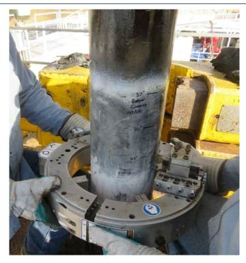
Figure 23: Cutting the 7 in. Casing
