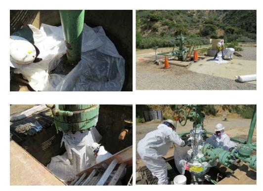
Figure 45: Applying Stripping and Wrapping to Frew 8 Wellhead
