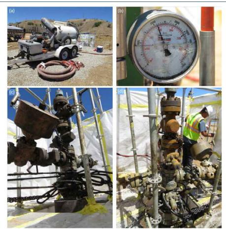
Figure 51: Hydroblasting of SS-25
