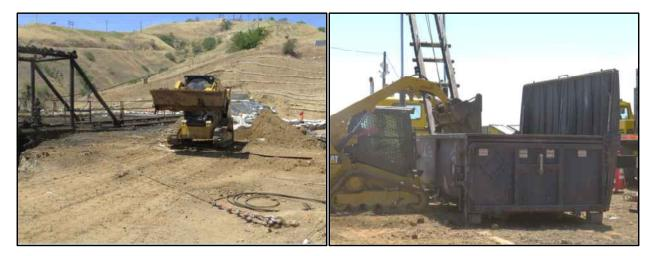
Figure 17: Excavated Crater Soil Placed in Bins with Front Loader
