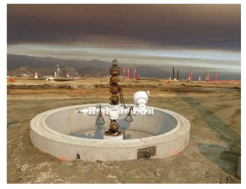
Figure 62: SS-25's Crater Slurry Backfilled to Site Grade Elevation
