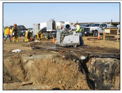
Figure 31: Concrete Well Pad Cut with Saw
