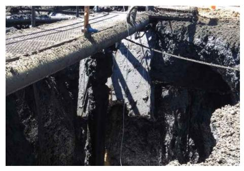
Figure 2: Concrete Slab Suspended from South Edge of Crater
