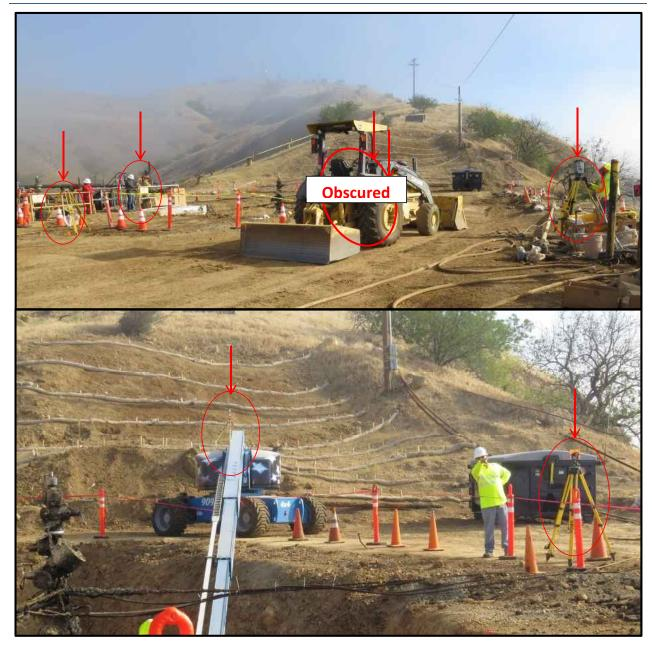
Figure 41: Site Benchmarked Vantage Points (Top), Picture of Obscured Points (Bottom)
