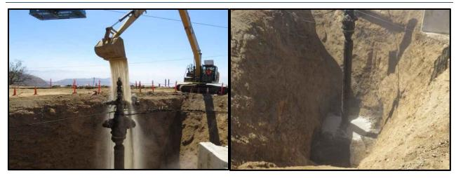
Figure 42: Placement and Mounding of Silica Sand on Crater Bottom
