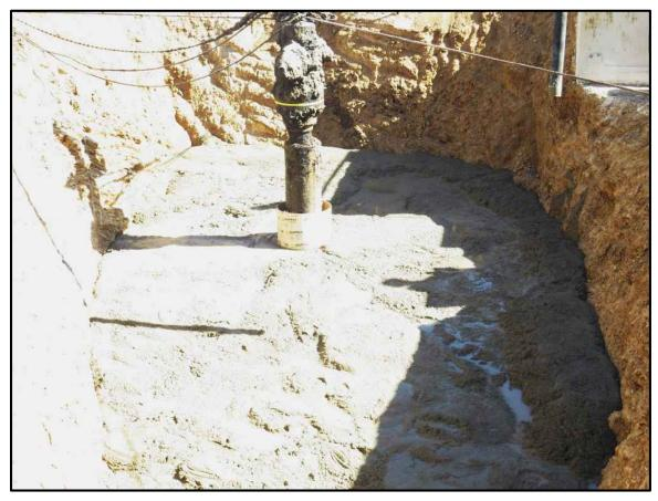
Figure 52: Crater After CLSM Placement to 12 ft Below Site Grade, Looking South
