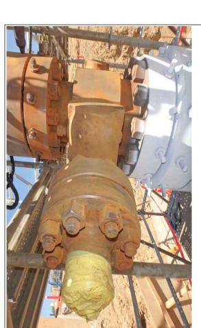
Description: Surface preparation of wellhead tree prior to MPI contrast paint
