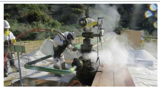
Figure 47: Waterblasting of the Frew 8 Wellhead
