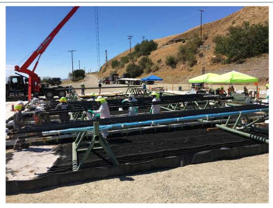
Figure 19: Tubing Unloading, Cleaning, and Coating Operations at PS-20
