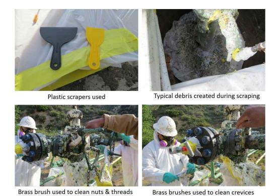
Figure 46: Removal of Debris After a 20 Hour Chemical Soak of the Frew 8 Wellhead
