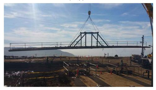
Figure 19: Wellhead Access Bridge - Crane Lifted from Crater
