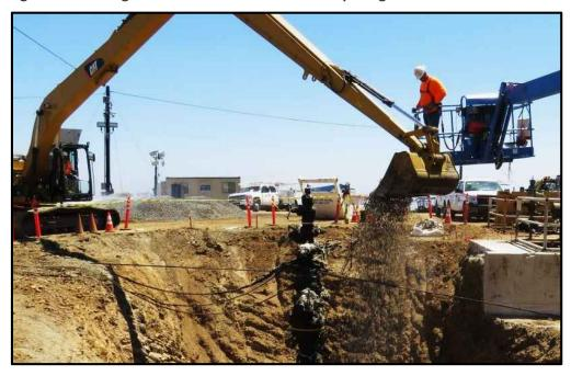
Figure 45: Placement of Gravel into Crater
