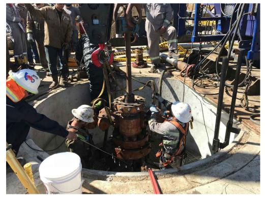
Figure 16: Removing the SS-25 Tree Assembly
