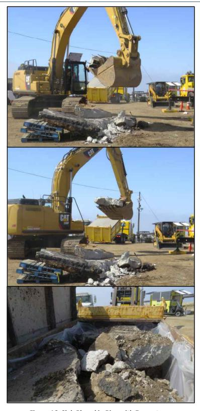
Figure 16: Slab Placed in Bins with Excavator
