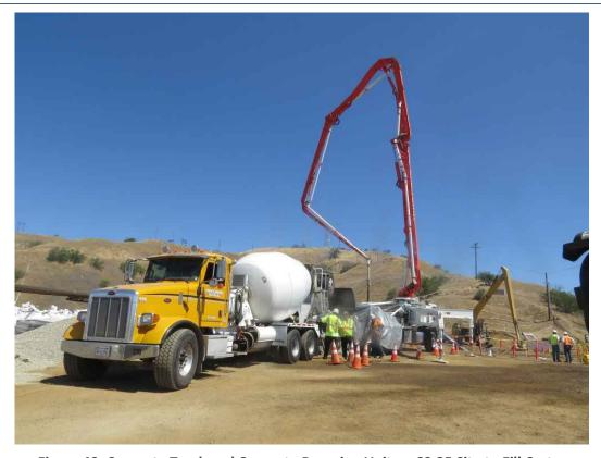
Figure 49: Concrete Truck and Concrete Pumping Unit on SS-25 Site to Fill Crater
