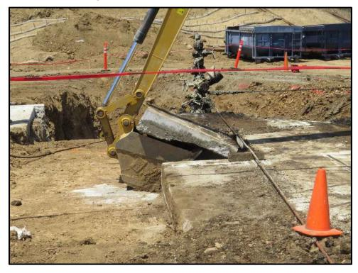
Figure 32: Concrete Well Pad Removed with Excavator
