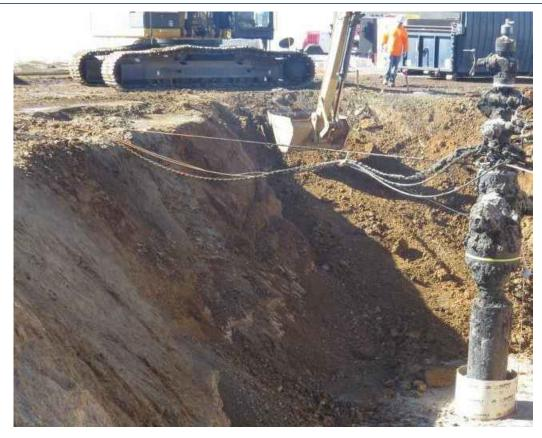
Figure 54: Excavator Used to Construct and Compact Earth Ramp with 3:1 Slope
