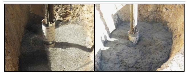
Figure 51: Crater Before (Left) and After (Right) First Concrete 24 in. Placement, Looking South
