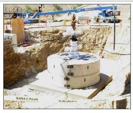
Figure 59: Two of Four 10 ft Diameter SS-25's Cellar Cylinder Segments of 2.5 ft Height Were Installed
