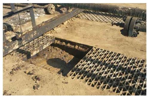
Figure 23: Debris in Pipe Trenches at Site Grade Elevation – Seen Upon Removal of Grating
