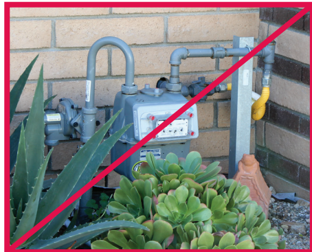
INADEQUATE WORKING SPACE
