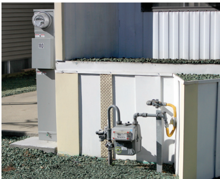
ADEQUATE WORKING SPACE
